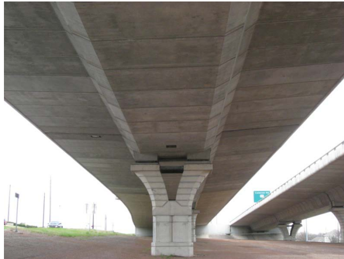
Figure 6.1: US 183 Bridge, Austin, Texas
