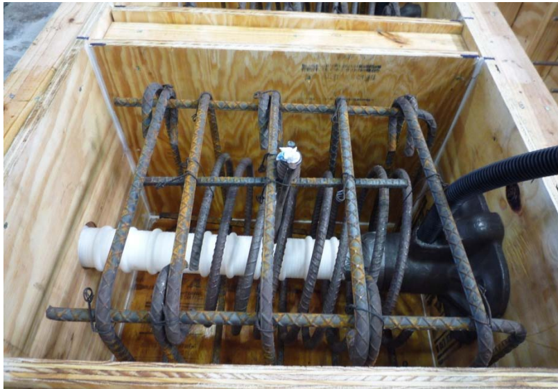
Figure 3.2: Reinforcement in Concrete Anchor Block
