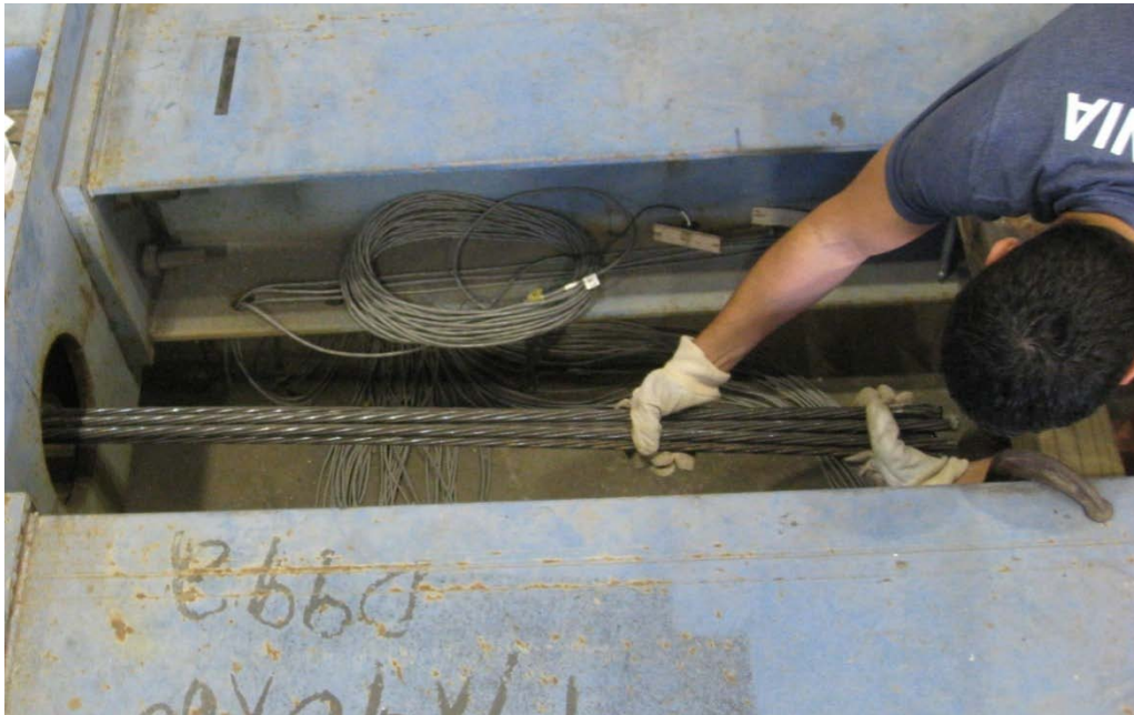
Figure 3.9: Pulling Strands Through Frame
