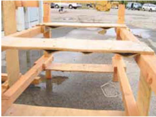
Figure 2.18 Buckling of Individual Plies in Plywood Braces ( FEMA StS2 Summary- Testing of Laced Post & Plywood Laced Posts, 2011 )
