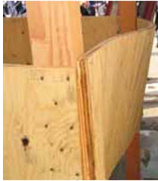
Figure 2.17 Lateral Torsional Buckling of Plywood Braces ( FEMA StS2 Summary- Testing of Laced Post & Plywood Laced Posts, 2011 )
