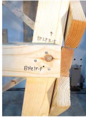
Figure 5.52 Photograph of 1 st Level Front Right Joint
