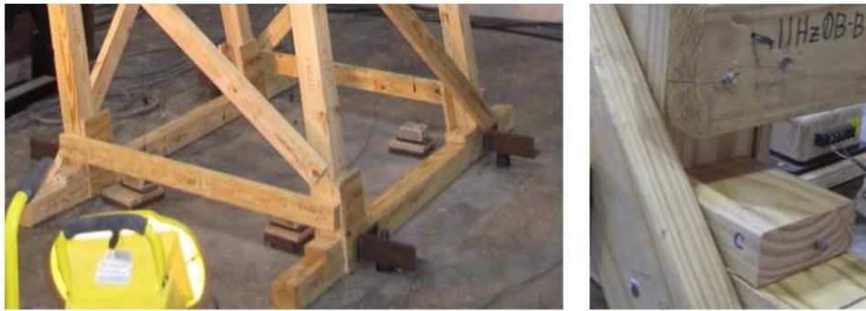
Figure 5.67 Status of the Wedges at Failure
