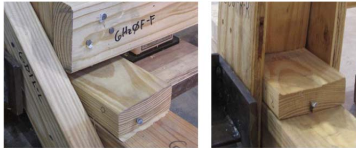
Figure 5.35 Condition of Wedges after Loading
