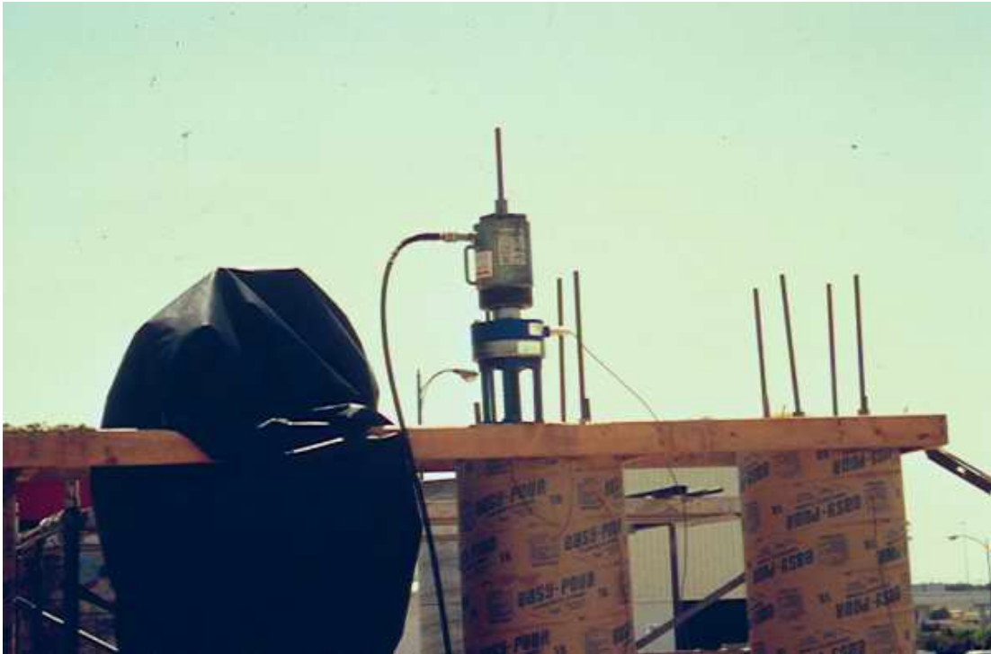
Figure 3.15: Stressing of Column 5 P/T Bars
