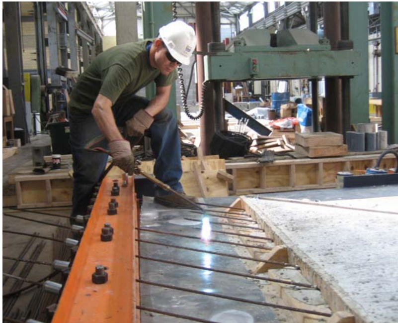
Figure 5.19: Cutting tensioned strands with acetylene torch
