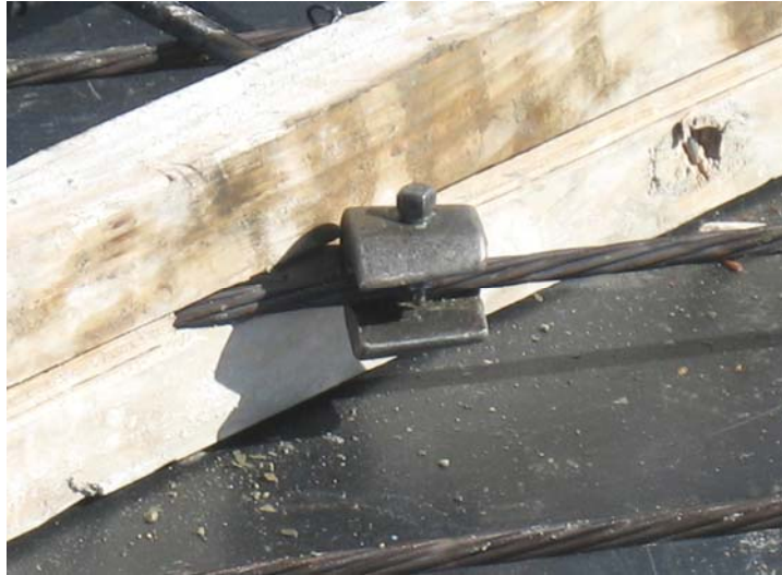
Figure 5.24: Clamp attached to strands to brace formwork
