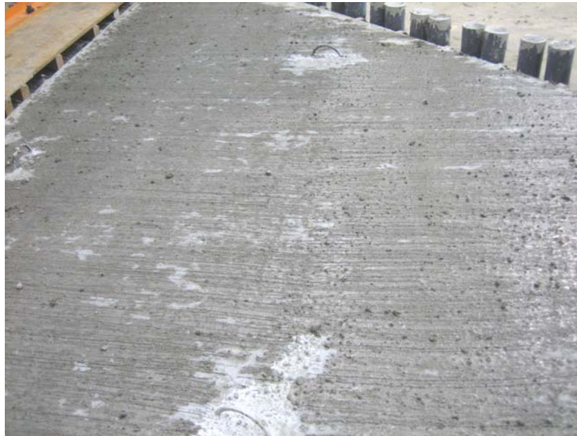
Figure 5.18: Finish created from broom
