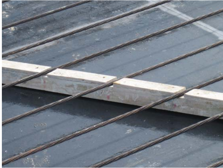
Figure 5.20: Bottom half of wooden forms for 30 degree skew panels
