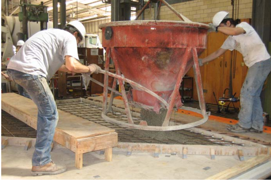
Figure 5.14: Placing concrete using one-yard bucket
