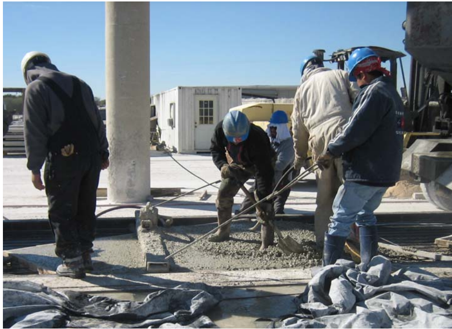
Figure 5.27: Leveling concrete with shovels and vibrating screed
