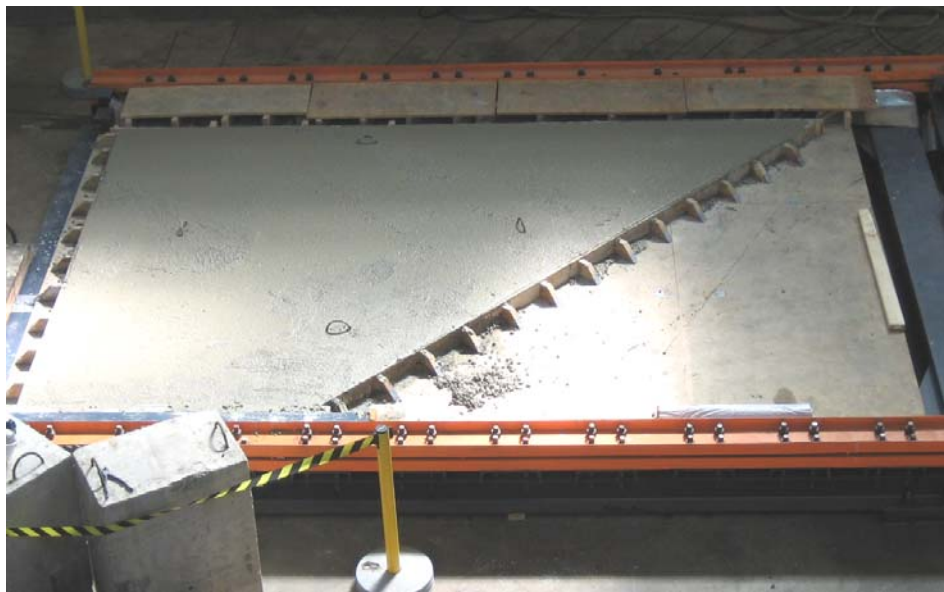
Figure 5.17: Completed panel prior to roughening the surface
