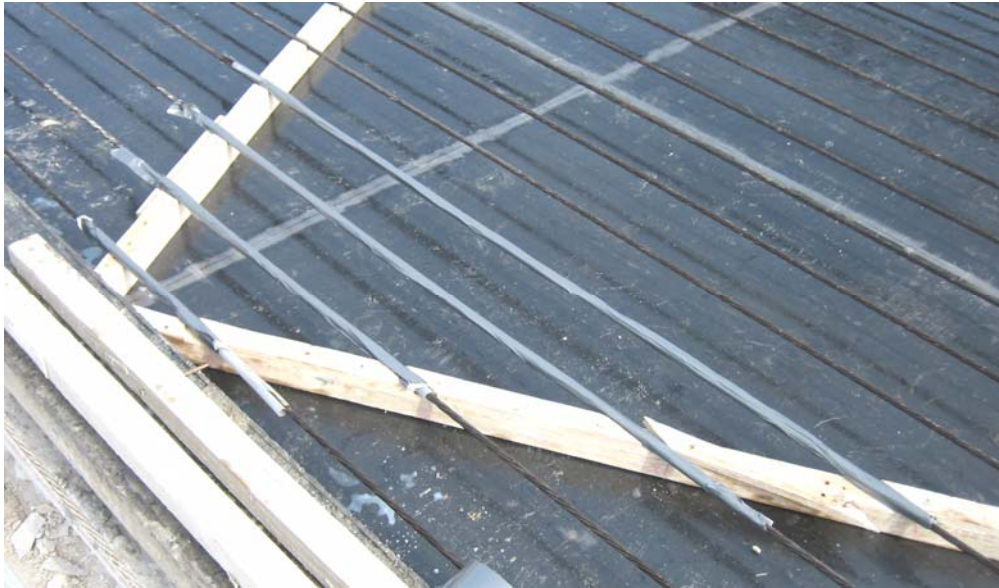
Figure 5.21: De-bonded strands for 30 degree skew panel
