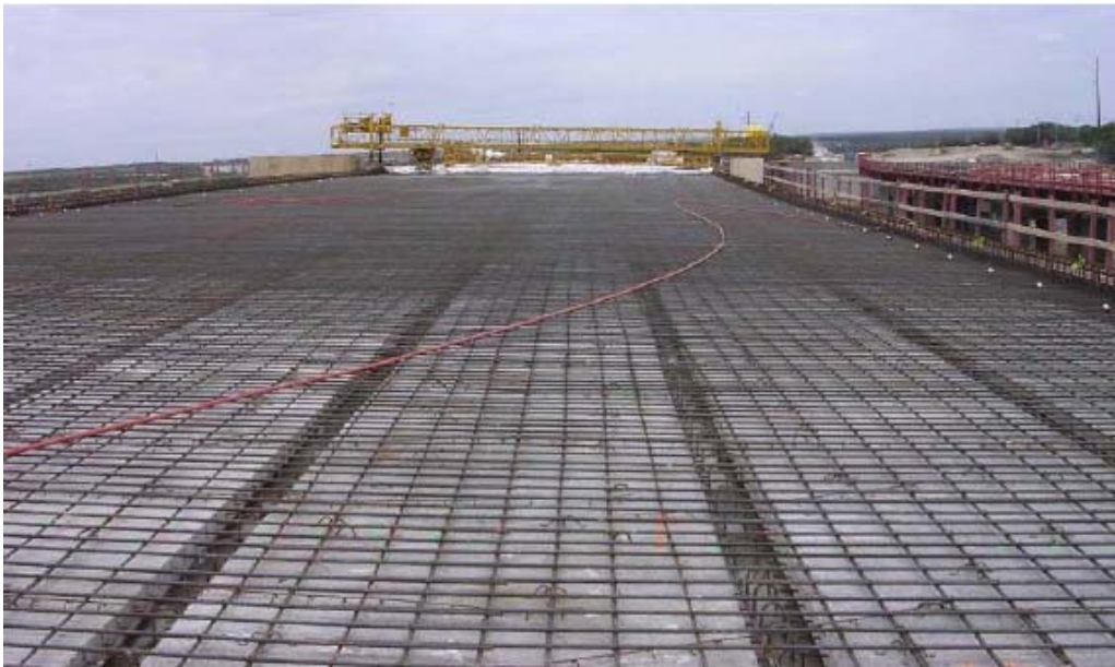
Figure 1.3: Panels and reinforcing steel prior to casting topping slab (Agnew 2007)
