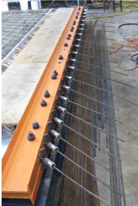
Figure 5.7: Live end anchorage after stressing strands for P45F60-1
