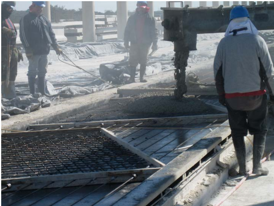
Figure 5.26: Placing concrete in casting bed
