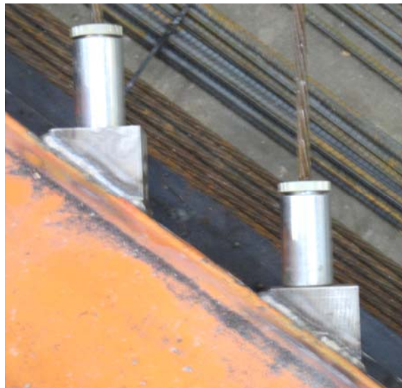
Figure 4.15: Plan view of typical bearing for parallel strands
