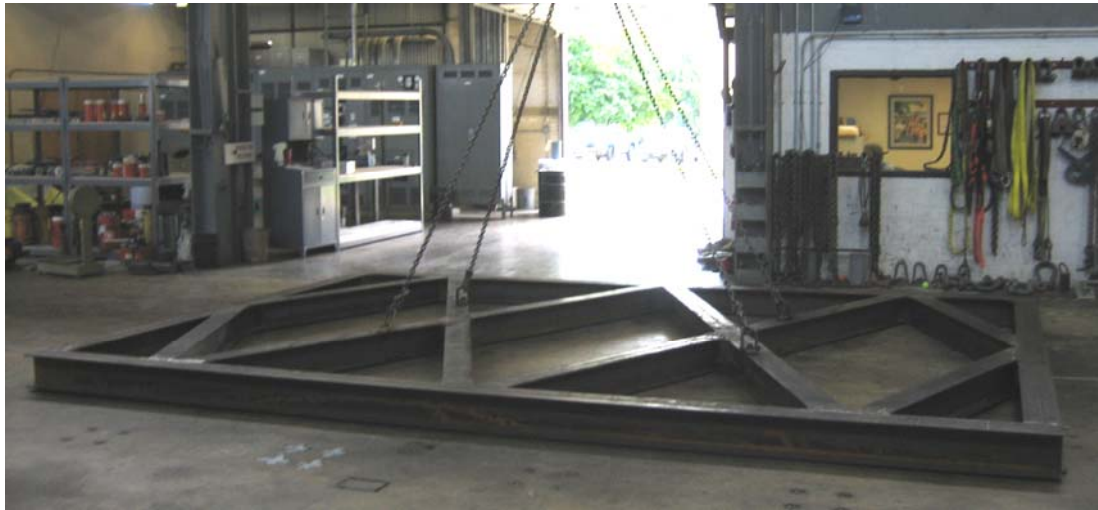
Figure 4.3: Completed base reaction frame
