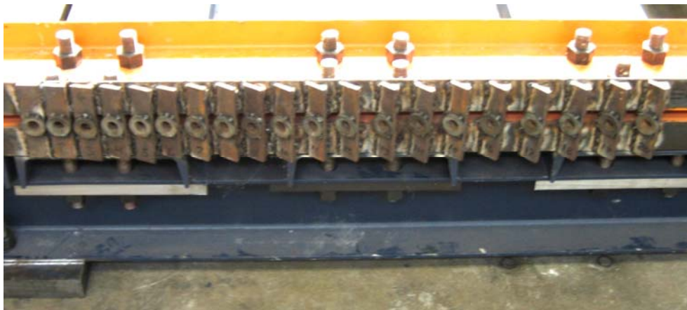
Figure 4.12: Completed dead end anchors for flared strands
