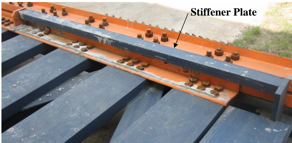
Figure 4.17: Stiffener plate
