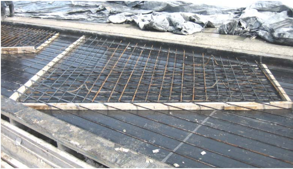
Figure 5.22: Finished rebar cage for 30 degree skew panel prior to formwork completion
