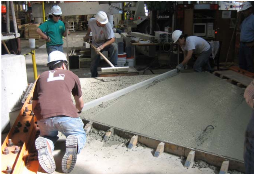
Figure 5.15: Leveling concrete with screed board
