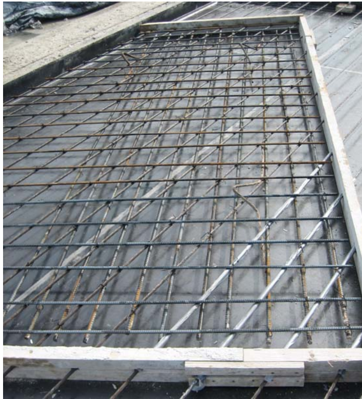
Figure 5.23: Flexural reinforcement in 30 degree skew panels
