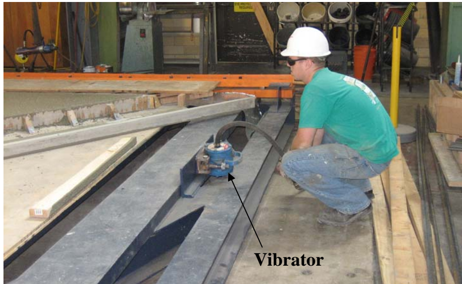
Figure 5.16: Form vibrator mounted on prestressing frame
