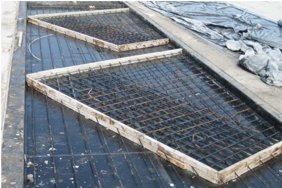
Figure 5.25: Two 30 degree skew panels ready for casting
