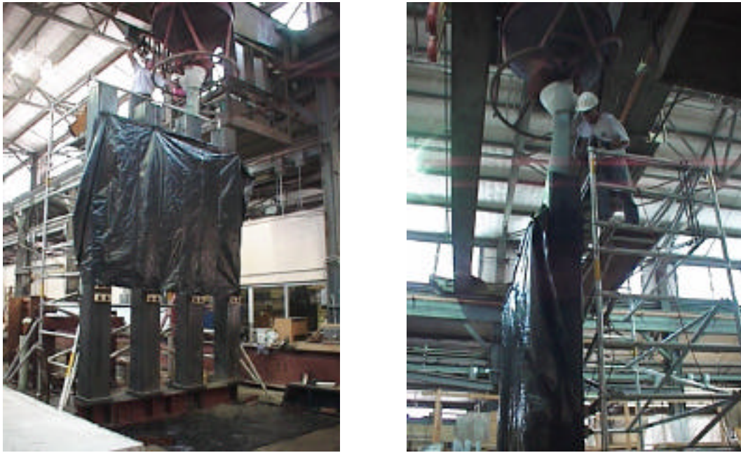
Figure 5.4 - Filling the tubes with concrete (left), and vibrating (right).
