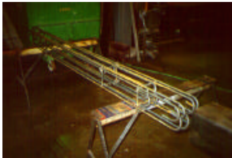
Figure 2.10 - Reinforcement for 8.B-C
