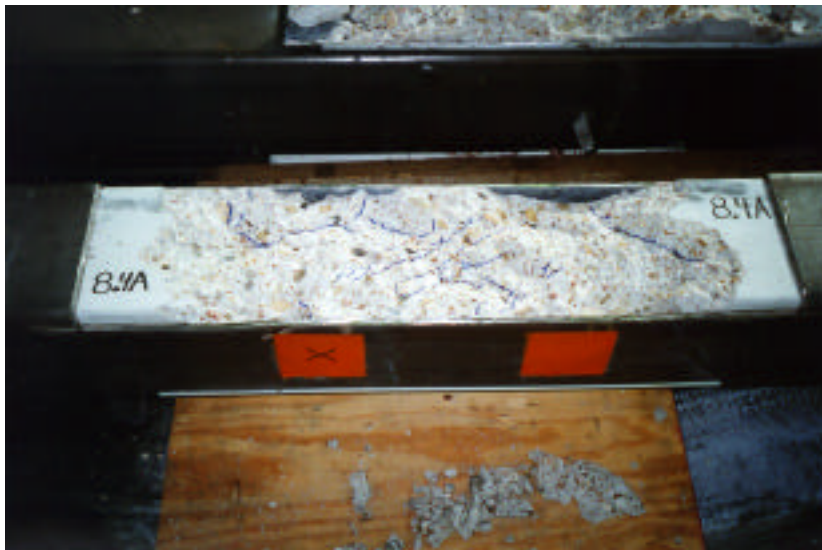
Figure 3.11 – General Crack Direction in 8.4A (Area of Contact Denoted by 4” x 4” Squares on Side)
