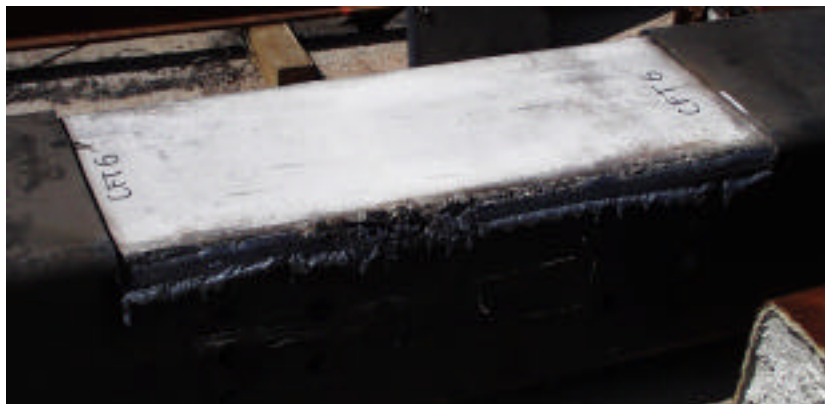
Figure 6.30 – CFT.6 with Panel-Zone Exposed and Intact
