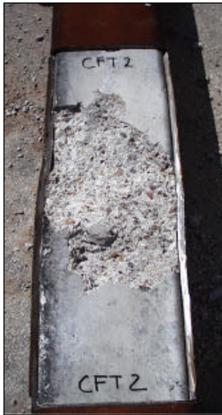
Figure 6.11 – Excavation of CFT.2 Concrete – Removal of Loose Material
