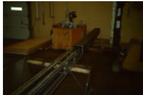
Figure 2.11 - Inserting Cage into 8.B-C
