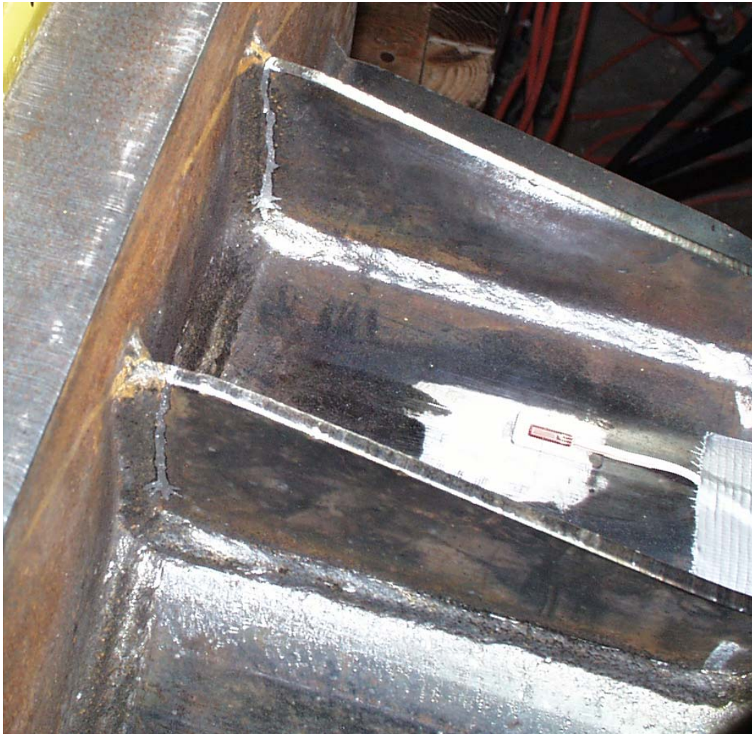
Figure 7.24 Failure of U-Rib Stiffened Specimen – Note: Painted lines represent extent of visible cracking.
