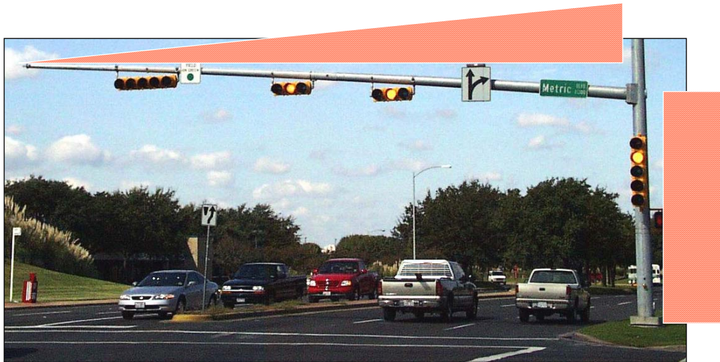
Figure 2.1 Moment Diagram on Cantilever Mast-Arm Traffic Signal
