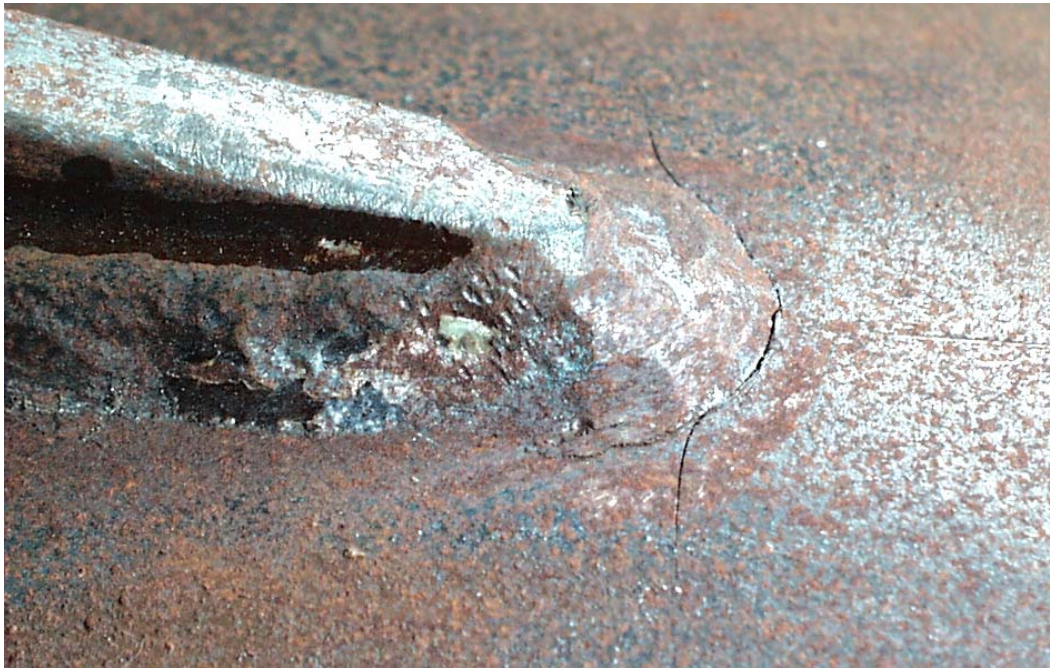
Figure 7.5 Failure of VAL 6x3/8 Specimen
