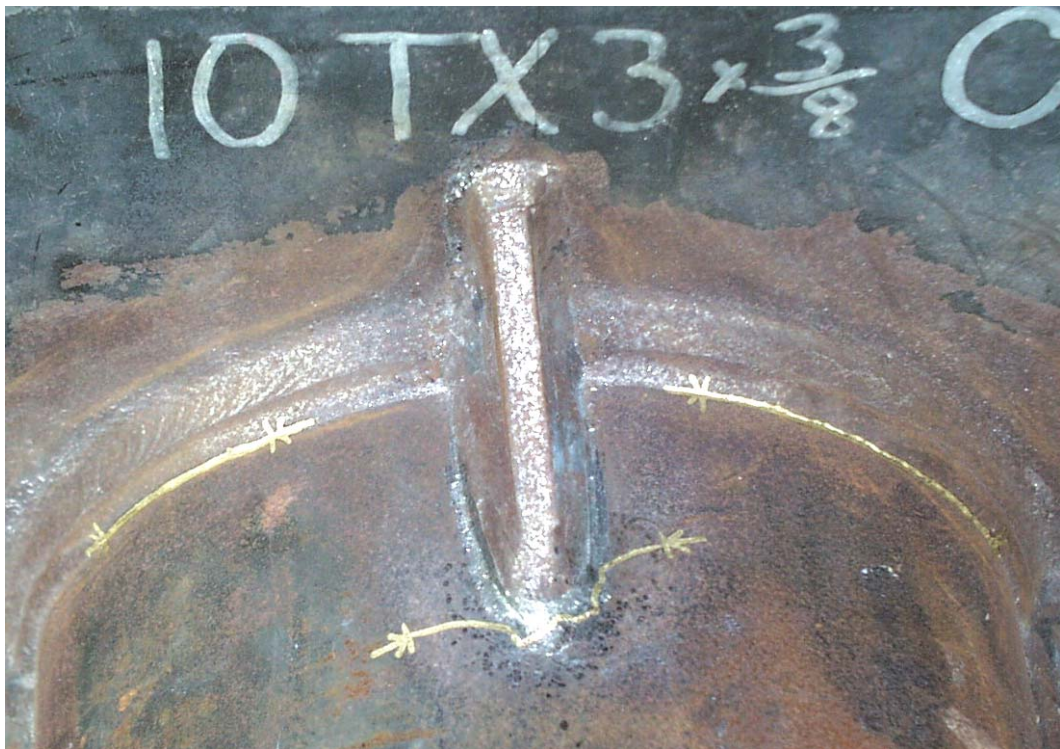
Figure 7.17 Failure of TX 3x3/8 CP Specimen – Note: Paint lines represent extent of visible cracking at termination of stiffener and socket weld toe.
