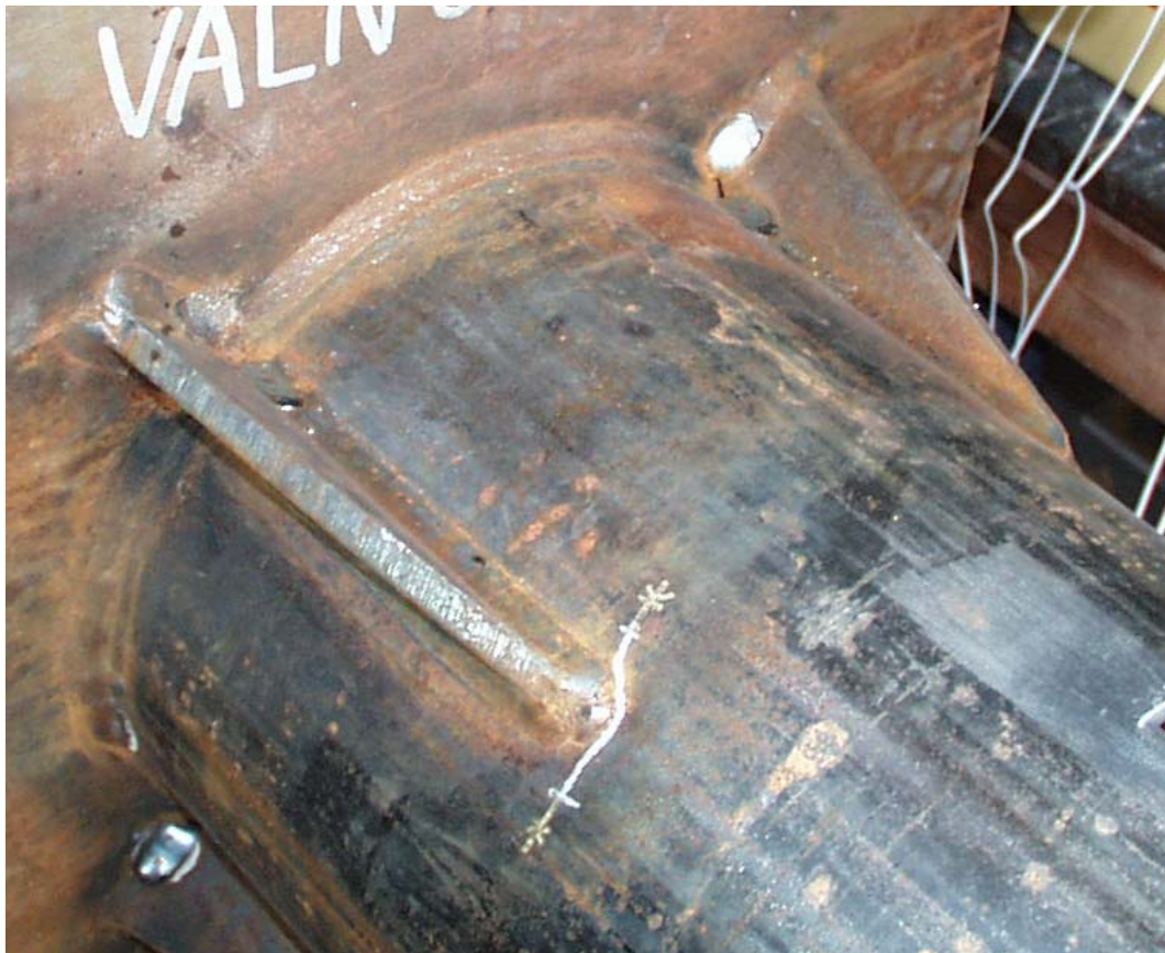
Figure 7.11 Failure of VALN 6x3/8@45 Specimen – Painted line indicates extent of visible cracking. Specimen tested at 6 ksi stress range.
