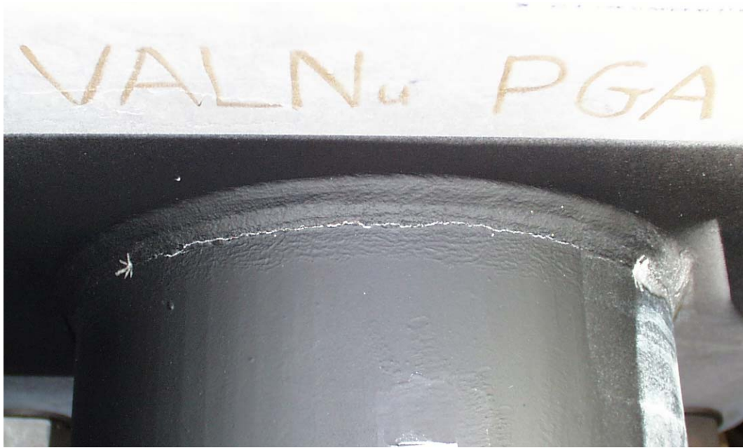
Figure 7.21 Failure of UIT Prior to Galvanization Specimen
