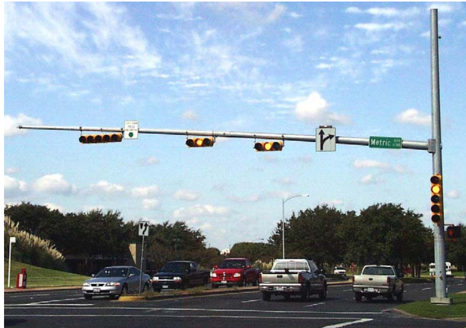
Figure 1.1 Typical Cantilever Mast-Arm Traffic Signal Support Structure
