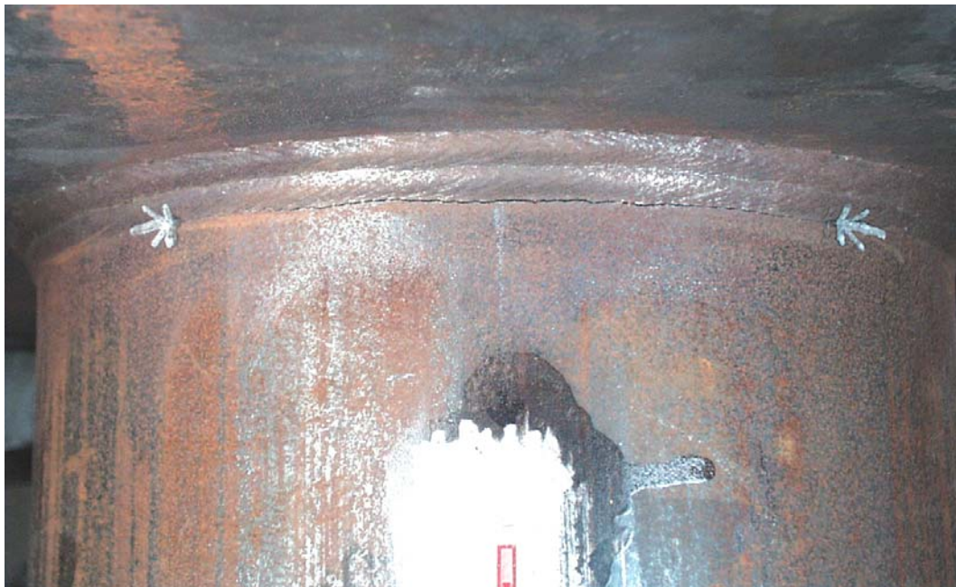
Figure 7.2 Failure of Socket Connection Specimen – Painted arrows indicate extents of visible cracking.
