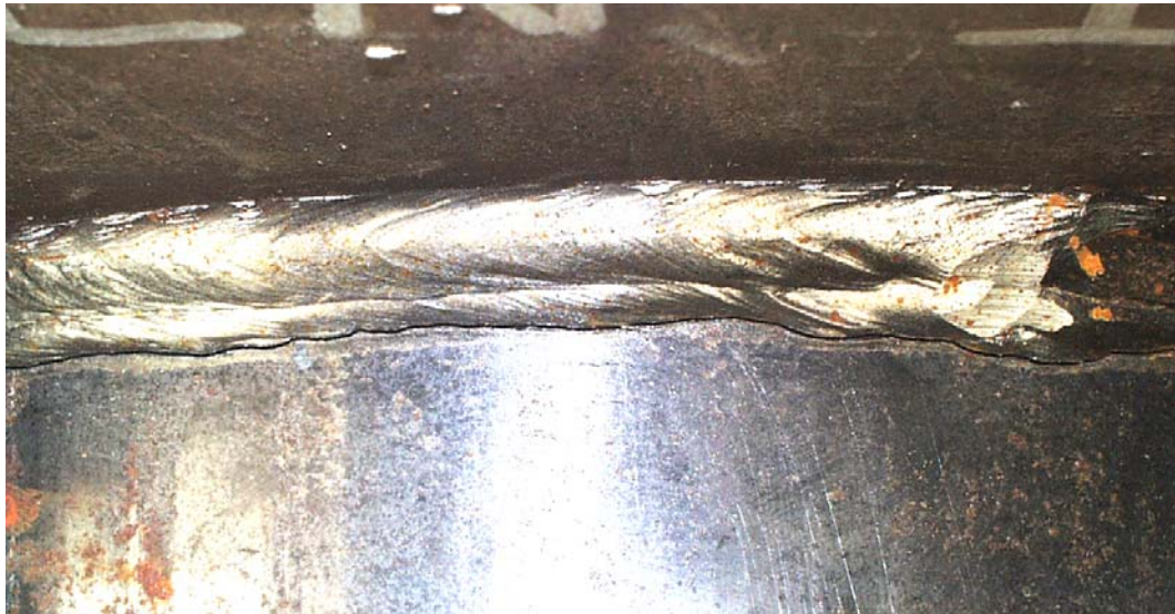
Figure 7.30 Failure of Internal Collar Stiffened Specimen
