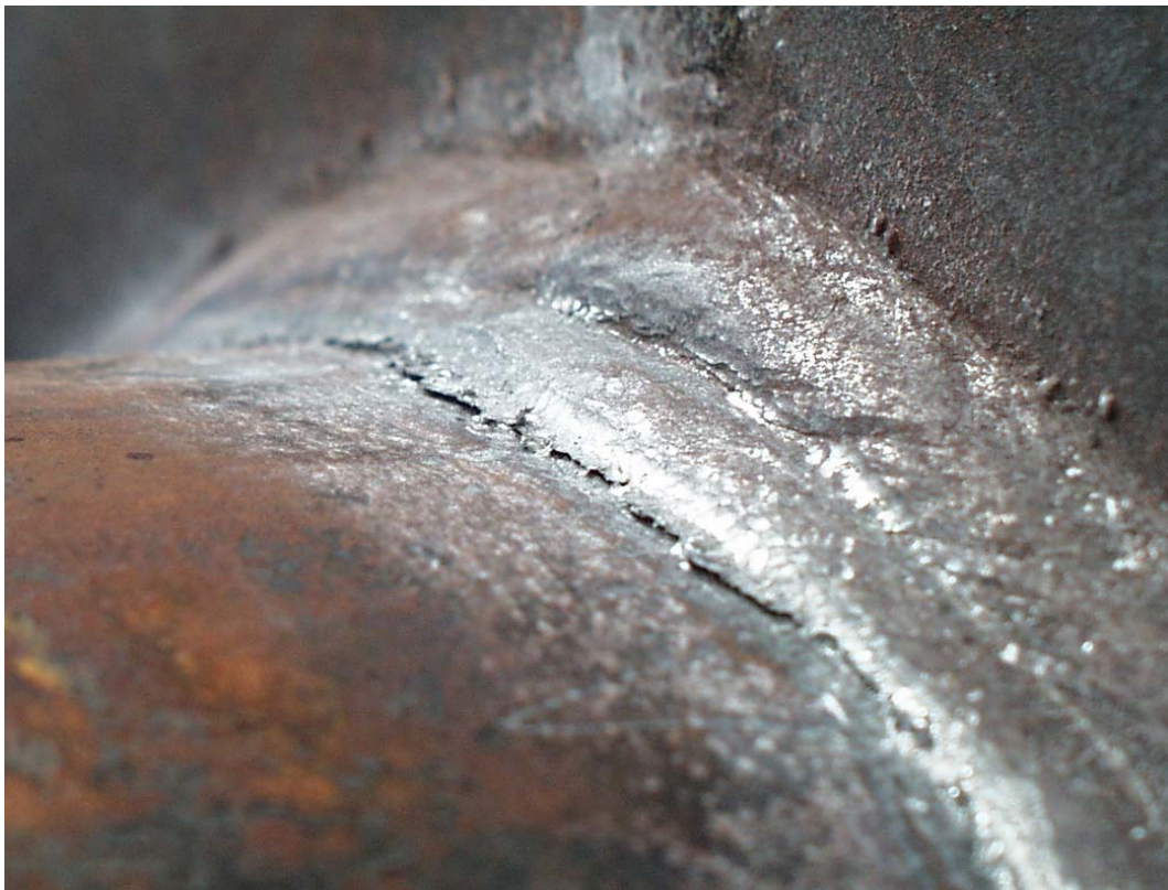
Figure 7.15 Failure of UIT Treated Socket Connection Specimen
