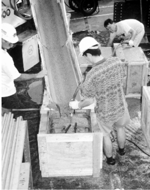
(a) Vibration of concrete
