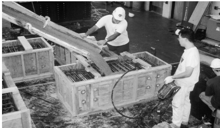
(b) Casting of concrete
