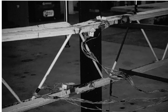
Figure 3.11 Failure Mode for 16K2-ND West Joist
