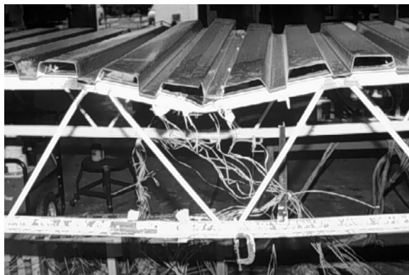
Figure 3.6 Failure Mode for 16K2-DX-1 East Joist
