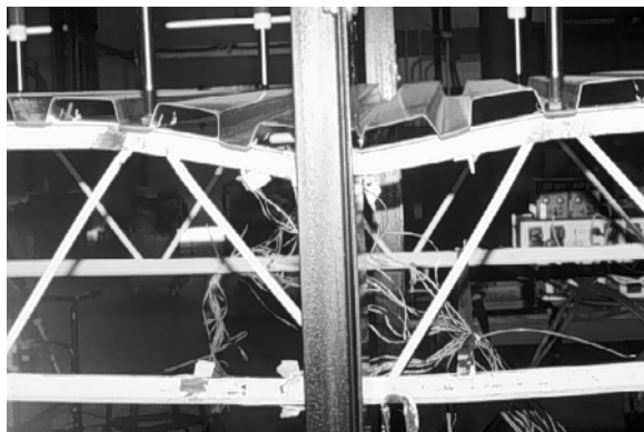
Figure 3.3 Failure Mode for 16K2-PW-2 East Joist
