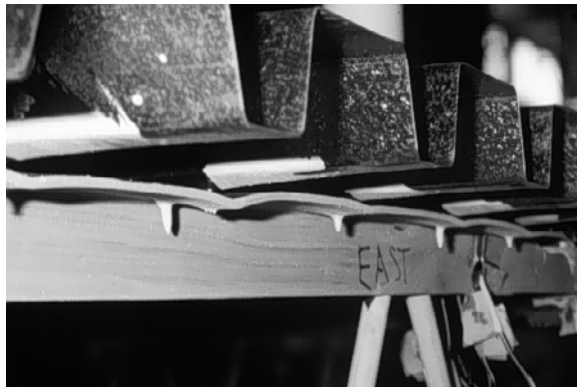
Figure 3.5 Distortions in Top Chord on Specimen 16K2-DX-1
