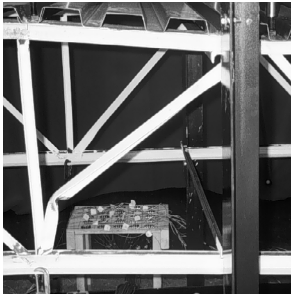
Figure 3.17 Failure Mode for 26K5-PW-2 West Joist
