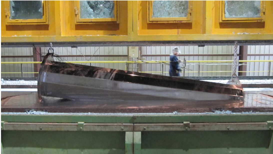
Figure 5-43: HMIP being lifted from the galvanizing bath
