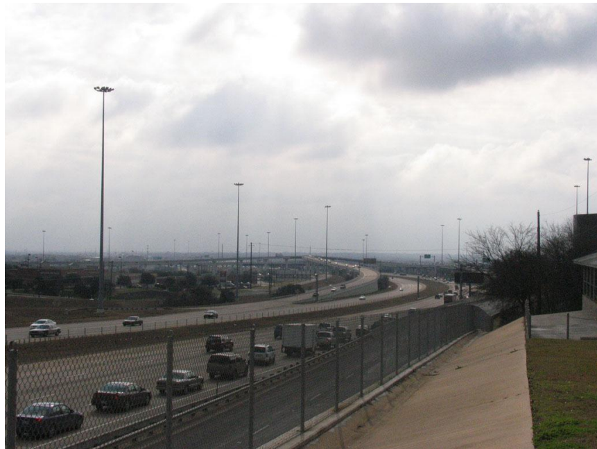
Figure 1-1: High masts at a freeway interchange (Rios, 2007)
