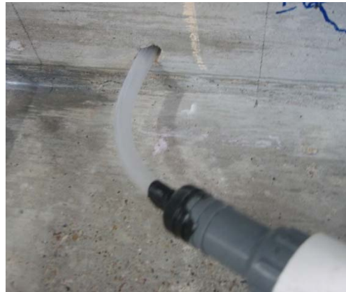
2) Cleaning the hole
