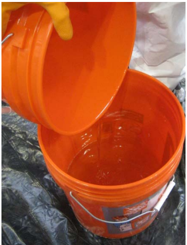
3) Mix component A and B
