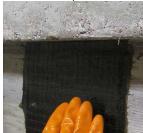
6) Attach the perpendicular directional patch
