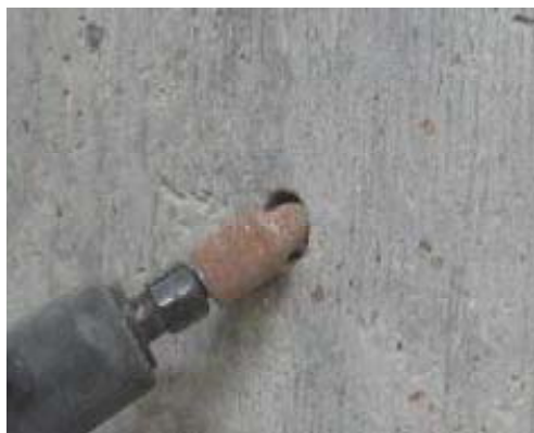
3) Rounding the edge of the hole
