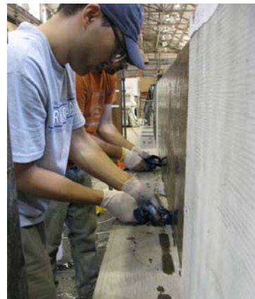
(b) Wetting the surface of the anchor holes
