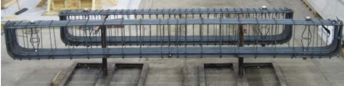
Figure A-4 12 ft. and 16 ft. bar cages
