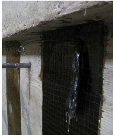
10) Placing into the embedded length
