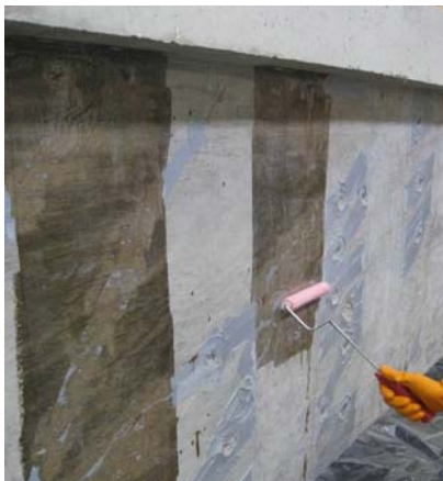
1) Saturate the surface of concrete
