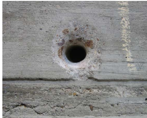
4) Completed CFRP anchor hole
