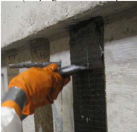
5) Removing excess epoxy
