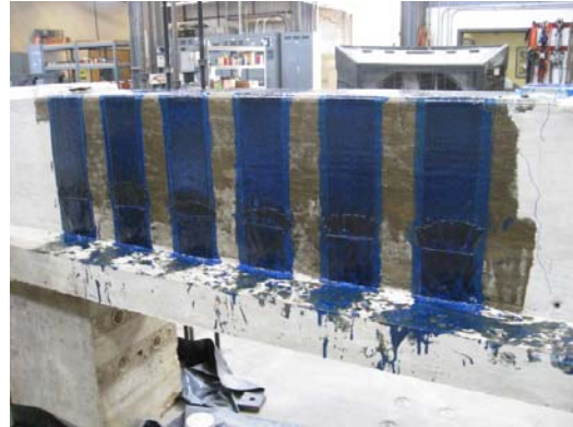
(f) Completed installation
