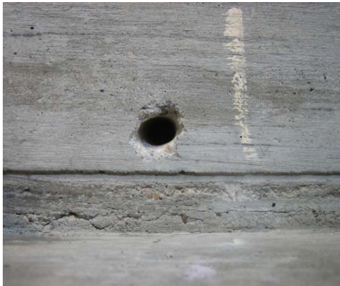
1) Drilling for anchor hole
