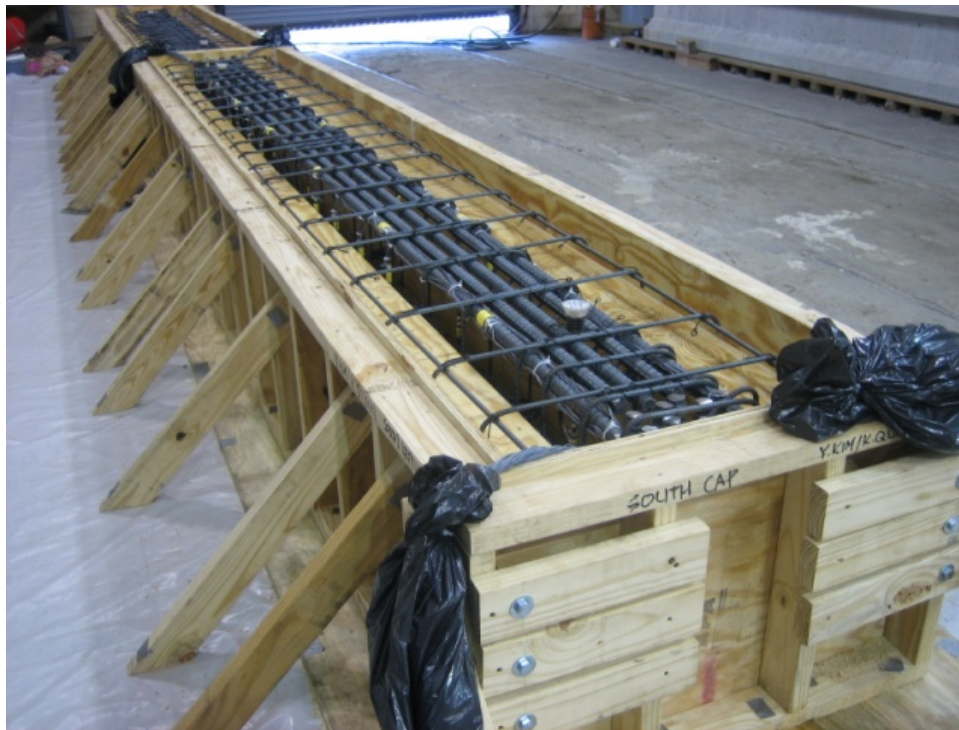
Figure A-3 Photos of the reinforcement in form (24 in.)
