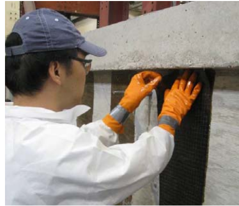
4) Attach CFRP strip to concrete surface
