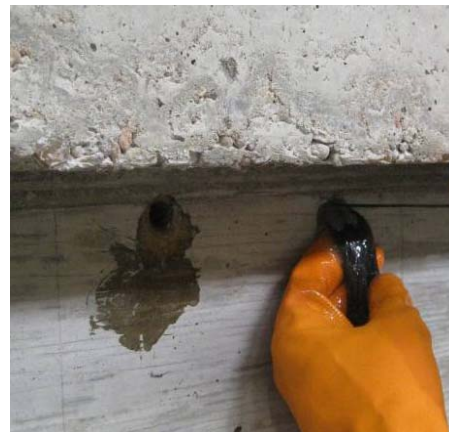
2) Saturate the anchor hole
