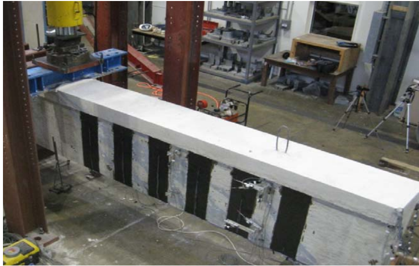
Figure 3-14 Photo of loading setup for 48 in. depth beams
