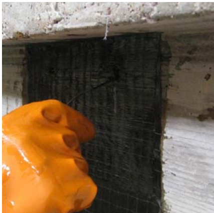
7) Creating an opening for CFRP anchor
