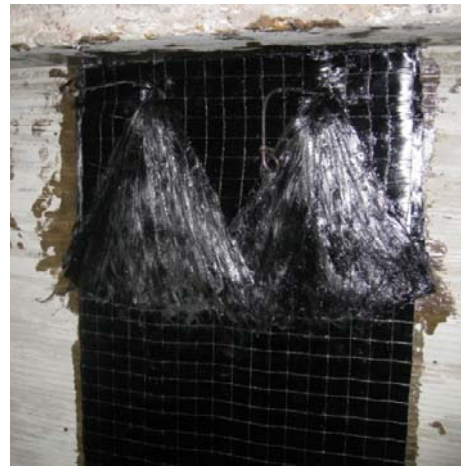
12) Repeating for another anchor
