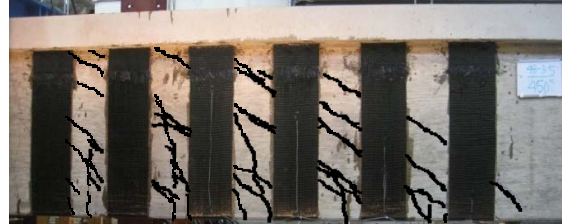
(b) Final crack pattern
