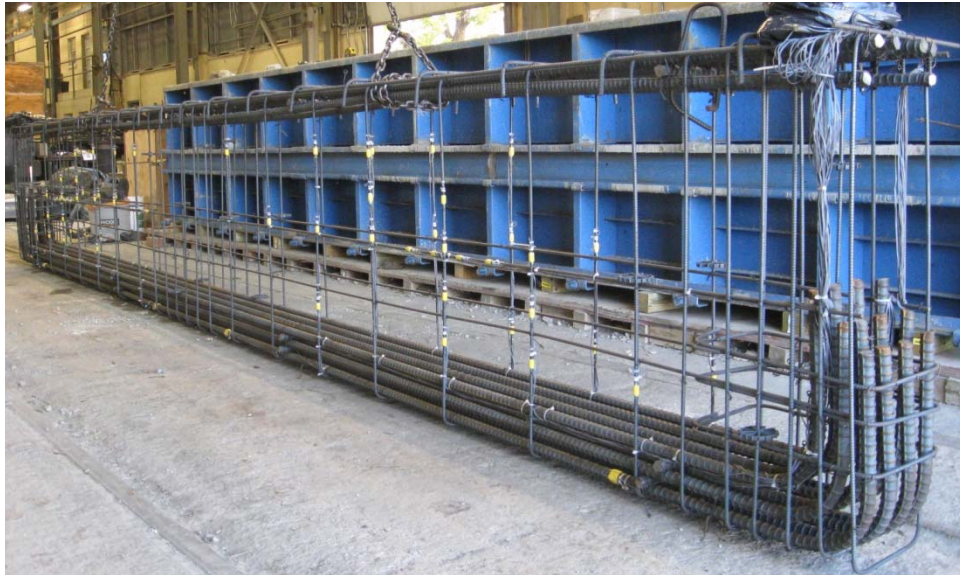
Figure A-8 Bar cage for 48 in. depth beam (#3@18")
