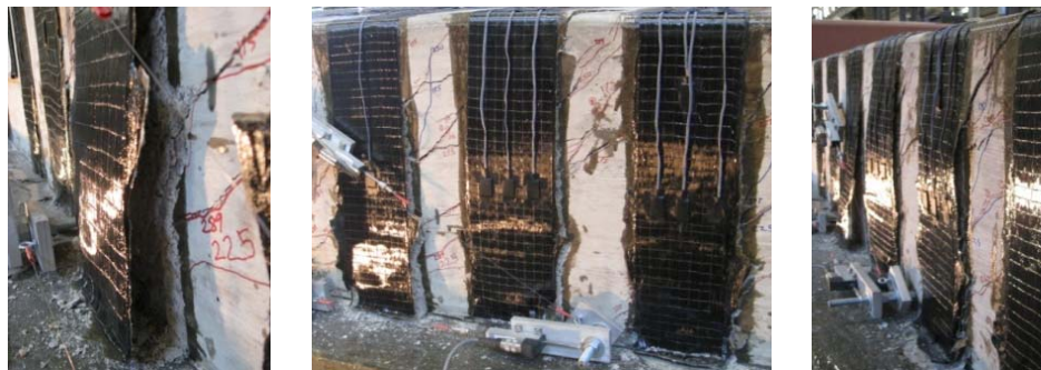
Figure 4-34 CFRP anchor failure of front side in 24-3-8
