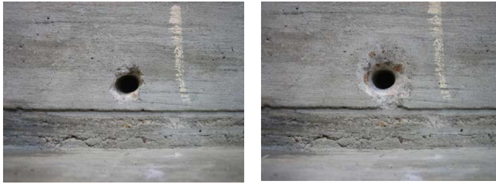
Figure 2-18 CFRP anchor holes before and after making hole chamfer
