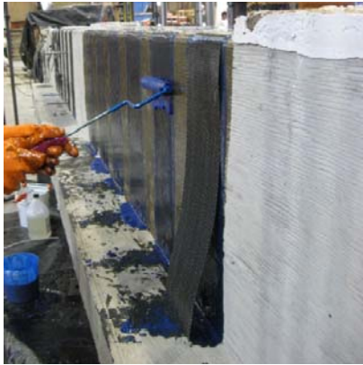
(e) Sealing the CFRP laminates with epoxy
