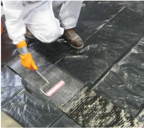
3) Impregnate CFRP strip
