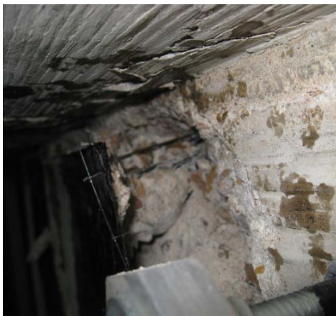
Figure 4-84 Fracture of CFRP anchors
