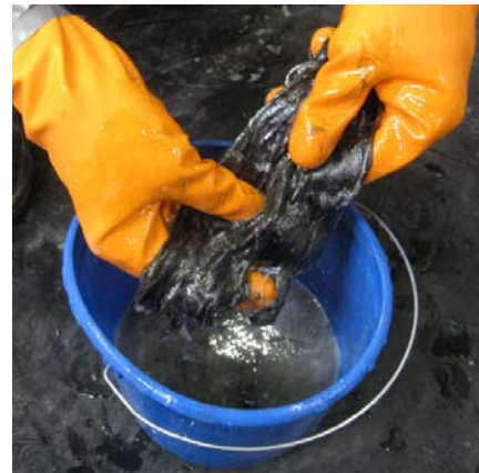
8) Impregnated the CFRP anchor
