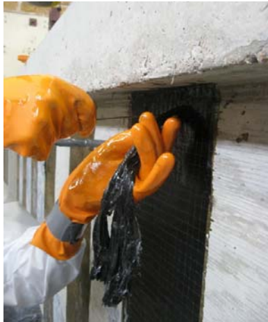
9) Inserting the anchor into hole
