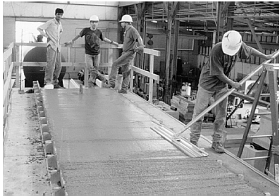
Figure 3.18- Bull-floating of Concrete Deck
