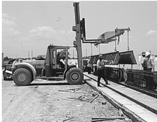
Figure 3.8- Placement of the Steel Side Forms
