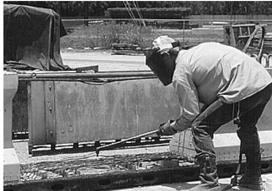
Figure 3.12- Release of Prestress by Flame-Cutting
