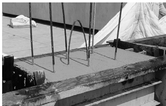
Figure 6.4- Finished Concrete Pull-Out Block
