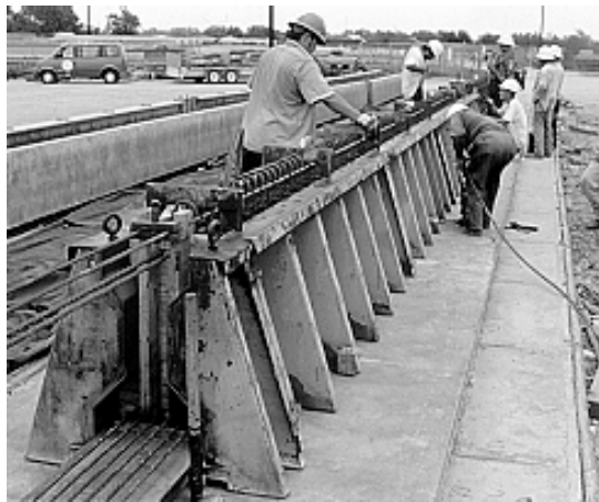
Figure 3.9- Anchoring of the Steel Side Forms
