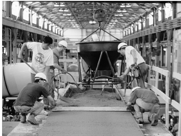
Figure 3.17- Transportation, Placement, and Vibration, and Screeding of Concrete
