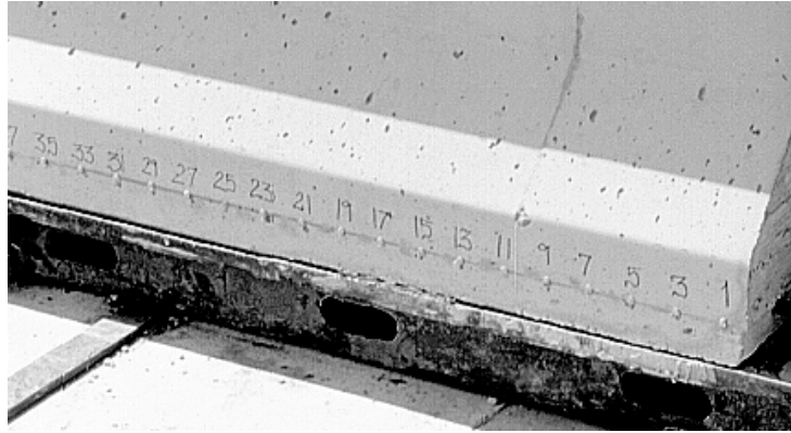
Figure 4.2- Demec Points Placed Along One Side of One End of One Beam
