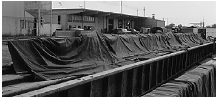
Figure 3.11- Curing of Concrete Beams
