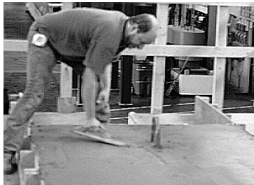
Figure 3.19- Finishing of Concrete Surface
