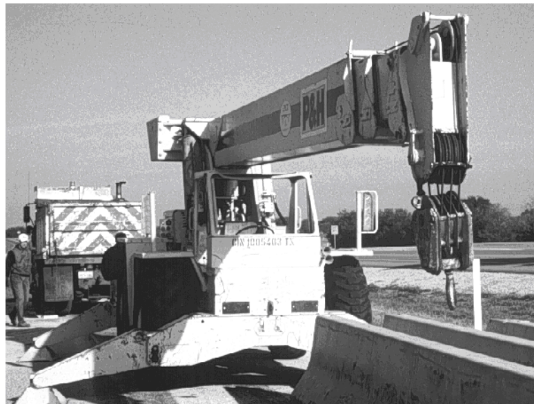
Figure 5.4 Loading Crane provided by Contractor.
