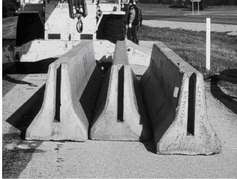
Figure 5.5 Jersey Barriers provided by Contractor.
