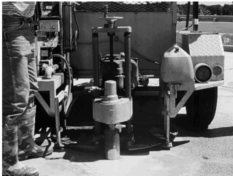
Figure 4.10 Drilling of Concrete Core in Progress.
