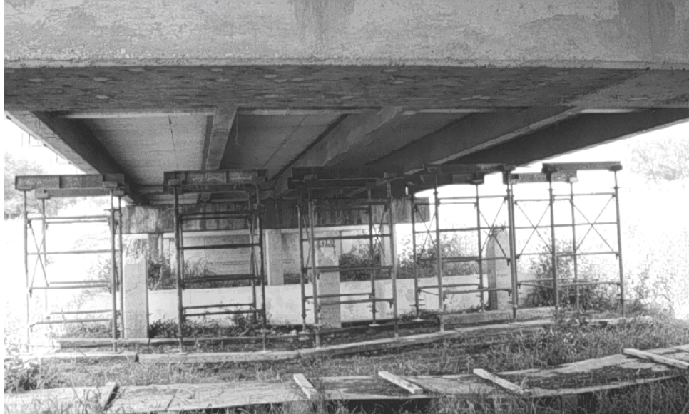
Figure 5.2 Temporary Shoring in Place under Unit-N.
