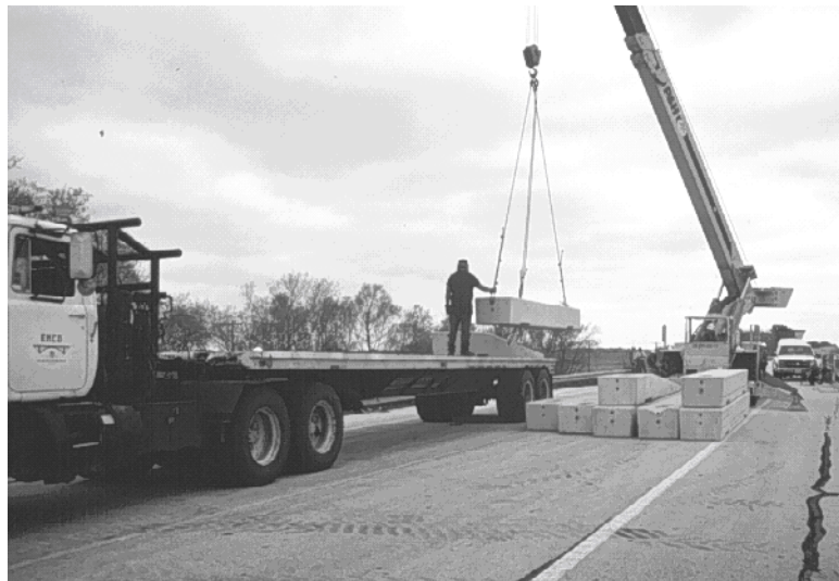
Figure 5.8 Barrier Placement on Flatbed of Trailer.
