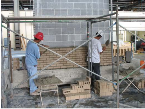
Figure 2-9 Laying clay masonry veneer
