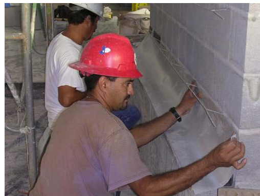
Figure 2-8 Installation of flashing
