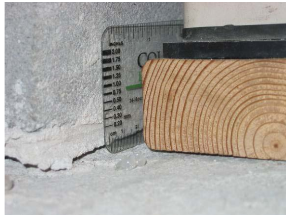
Figure 5-12 North end of CMU wall at the base under the first 1.0 in. loading to the north (Specimen UT CMU 3)
