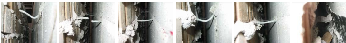
Figure 4-21 Connectors at 0.5-in. tensile displacement (top to bottom at west side)
