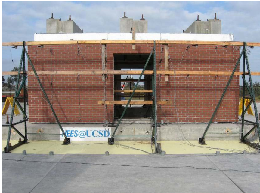
Figure 7-7 Clay masonry veneer on east side with reference frame system
