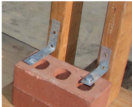
Figure 1-3 Connectors for wood-stud frame backing, corrugated connector (left) and rigid connector (right)
