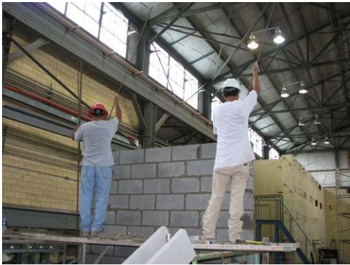
Figure 2-5 Placement of vertical reinforcement
