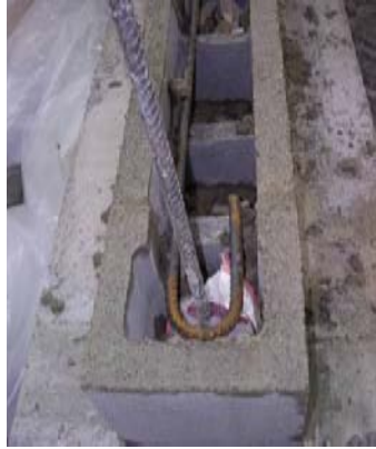
Figure 2-3 Detail of horizontal reinforcement and knocked-out webs
