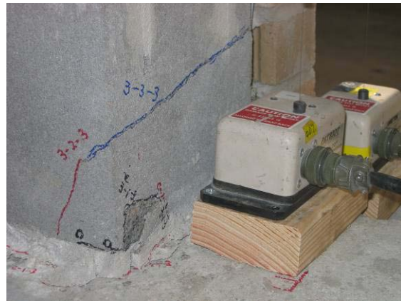
Figure 5-24 North end of CMU wall at the base under the first 1.0 in. loading to the north (Specimen UT CMU 4 MC)
