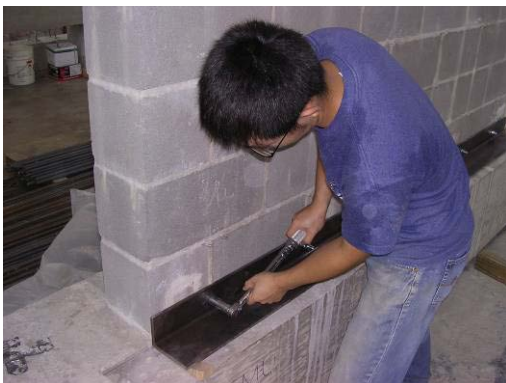
Figure 2-7 Placement of shelf angle
