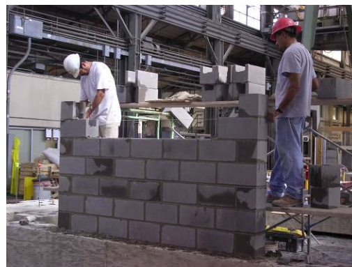
Figure 2-2 Hollow concrete masonry units being laid
