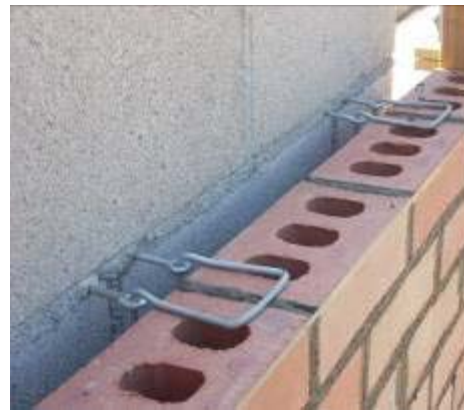
Figure 2-12 Double eye-and-pintle connectors
