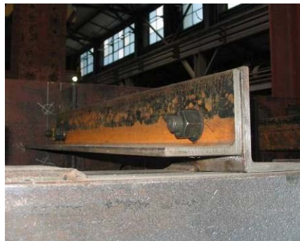
Figure 4-9 Simple connection between top of CMU wall and braced reaction frame
