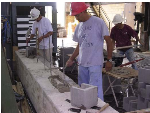
Figure 2-1 Base foundation with dowel bars
