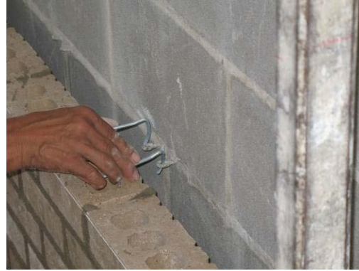
Figure 2-10 Installing connectors to clay masonry veneer
