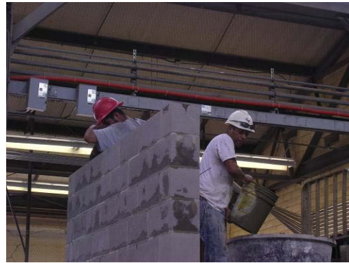
Figure 2-6 Grouting of concrete masonry
