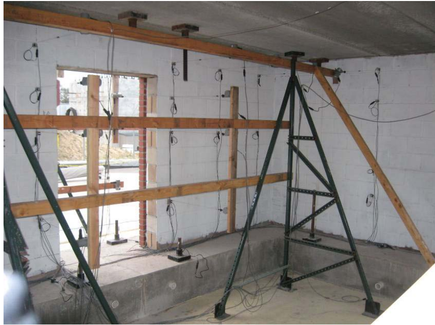
Figure 7-6 CMU wall on east side with reference frame system
