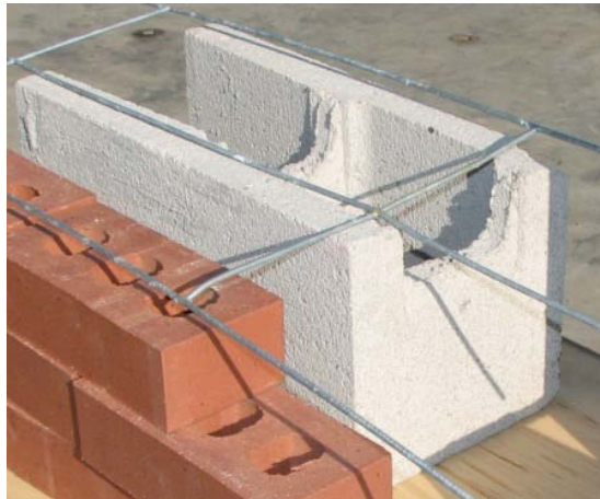
Figure 1-4 Connectors for concrete masonry backing, tri-wire connector
