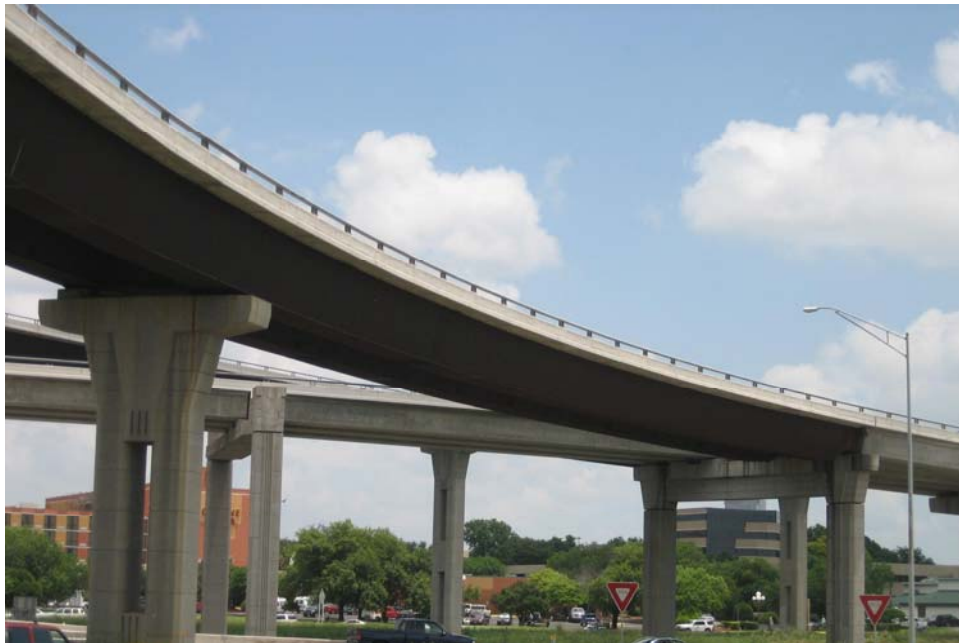
Figure 1-1: A typical twin box-girder overpass in Austin, TX
