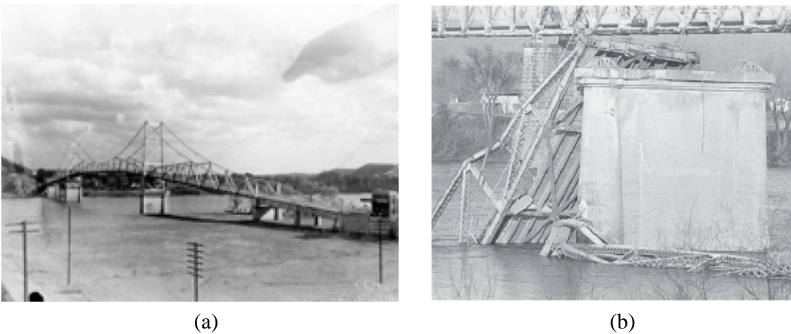
Figure 2-3: The Point Pleasant Bridge, (a) pre- and (b) post-collapse (unknown, Connor et al. 2005)
