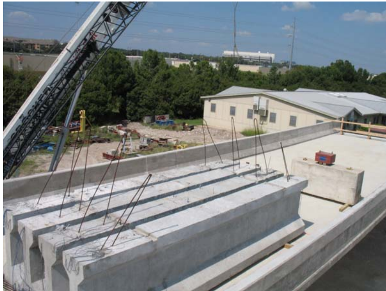
Figure 3-11: Concrete used to represent the AASHTO truck on the test specimen
