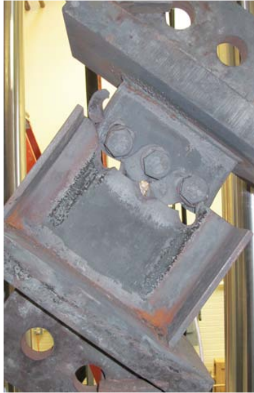
Figure 5.29 Connection failure after inclined tension test at 700°C – 1 inch A325 bolts
