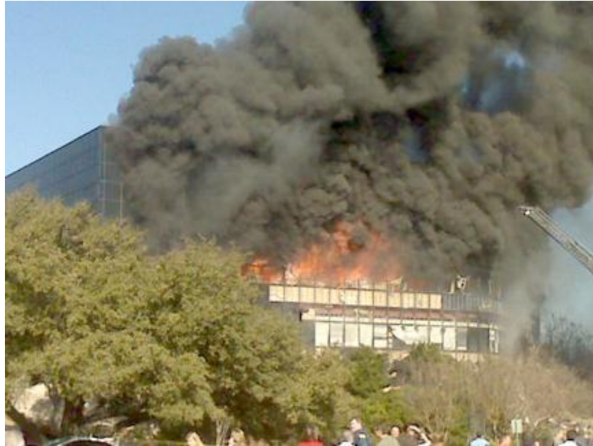
Figure 1.7 Echelon Building fire in Austin Texas ( www.myfoxboston.com , February 18 2010)
