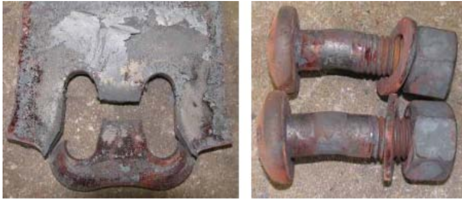
Figure 2.23 Block shear connection failure at 800°C (Yu 2006)
