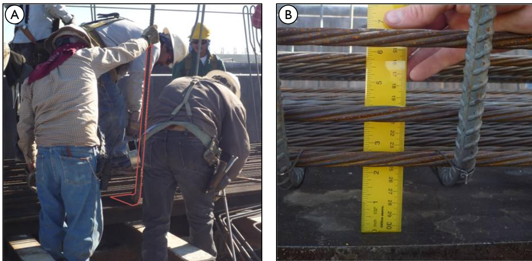
Figure 5-10: Workers using a 1.5 in. pry bar (outlined) to lift bottom strands; (B) resulting strand locations.
