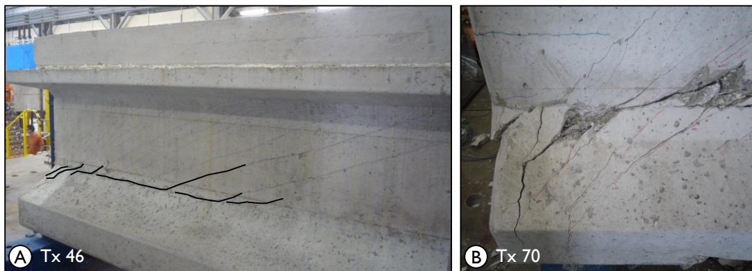
Figure 2-17: Horizontal shear damage visible in specimens (A) Tx46-S and (B) Tx70-N.
