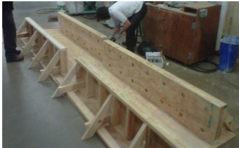
Figure 4-8 Construction of formwork for beams
