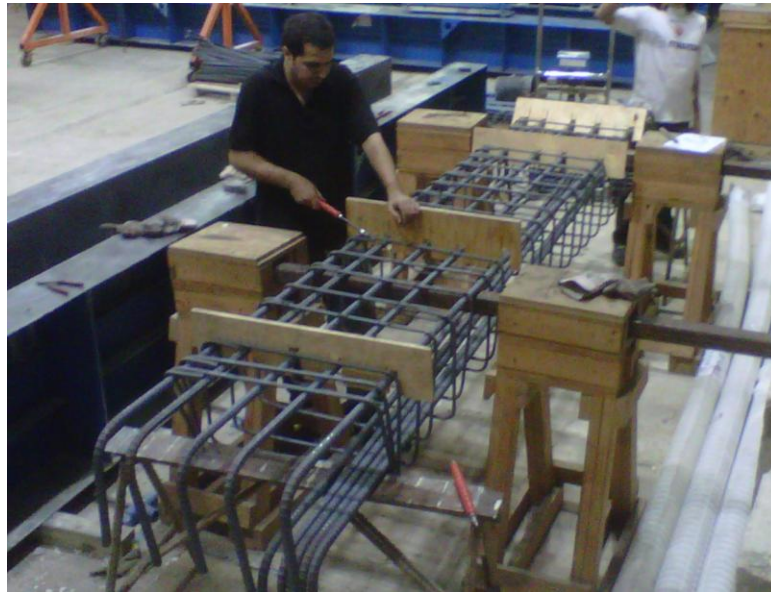
Figure 4-9 Assembling reinforcement cages for beams
