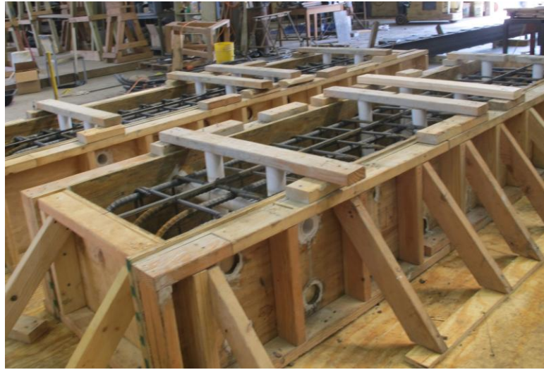
Figure 4-10 Typical beams before casting
