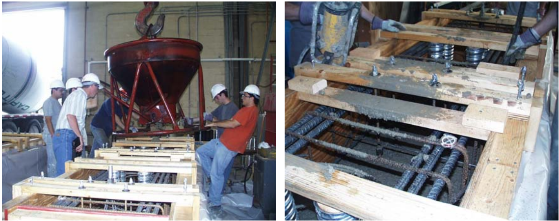
Figure 4.12 Placement of Concrete
