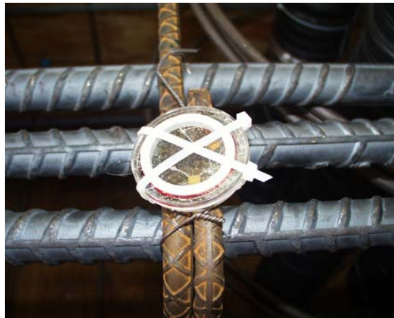
Figure 4.11 Sensor Attached to the Rebar Cage
