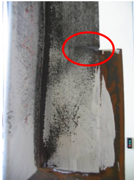
Figure 33. Typical Static Failure of Angle
