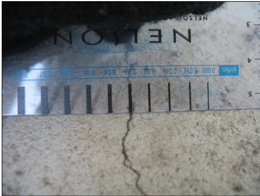
Figure A-20 – Top of ledge at interface (0.03 inches) (c in Figure A-17)
