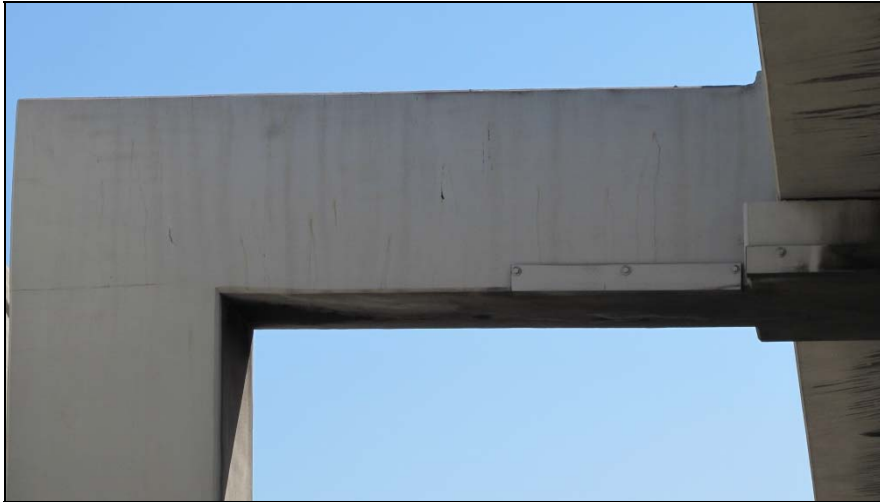
Figure A-51 - Overall of NW corner of Bent 5
