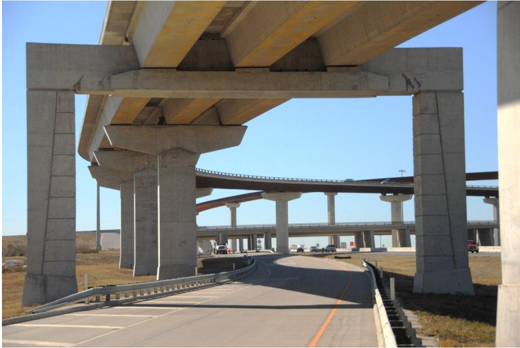
Figure A-57 – Overall of north side of Bent 17
