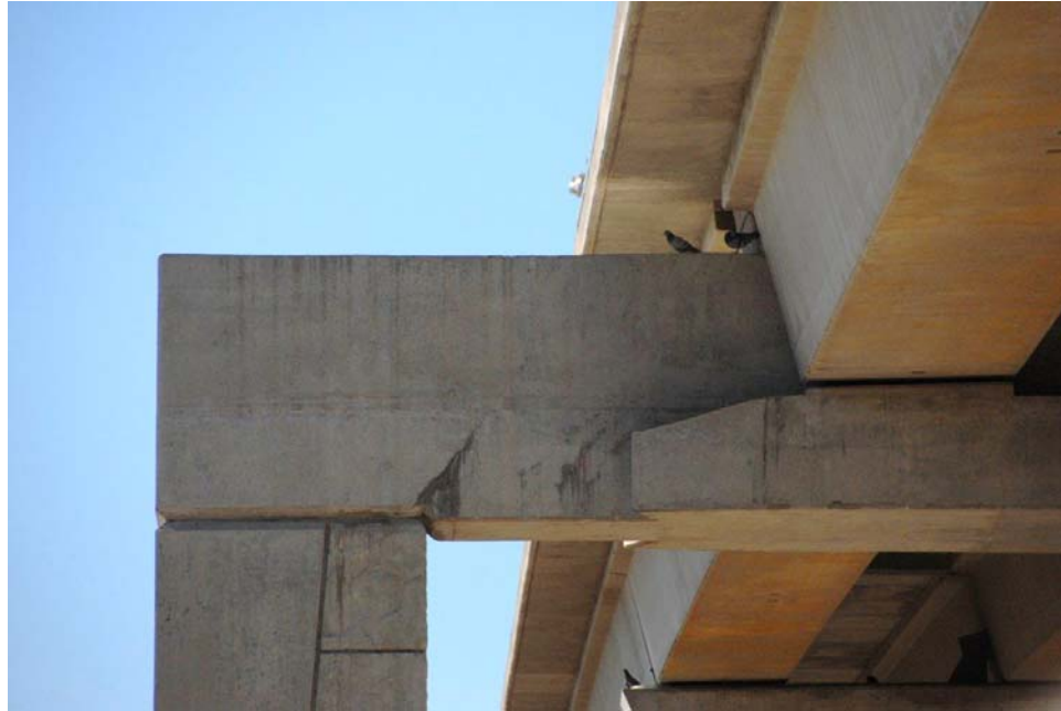
Figure A-58 - Overall of NE corner of Bent 17
