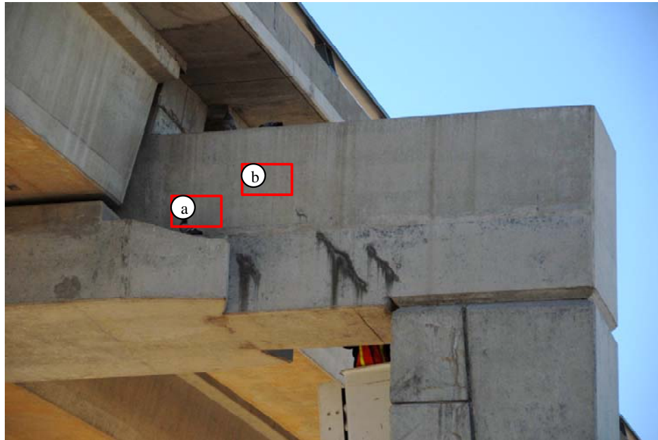
Figure A-59 - Overall of NW corner of Bent 17
