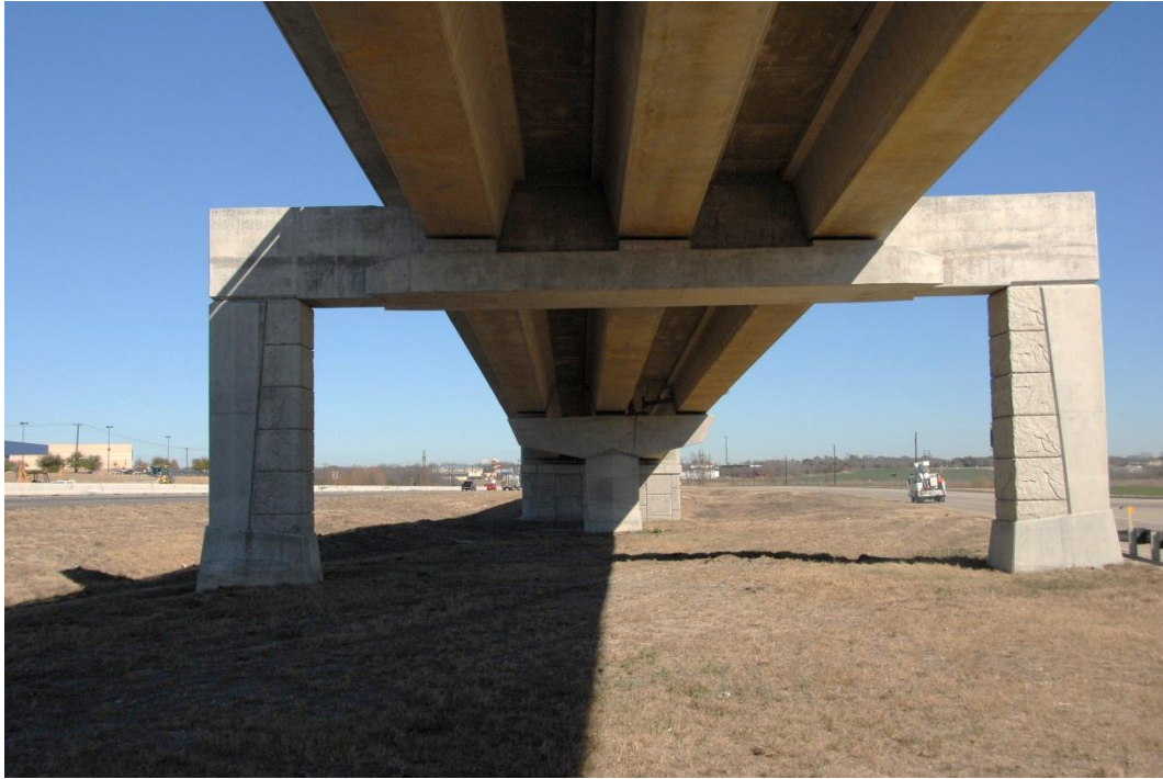
Figure A-78 – Overall view of south side of Bent 19
