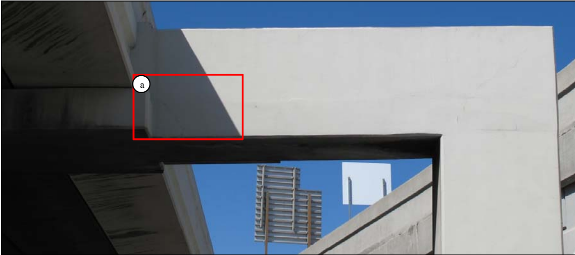
Figure A-53 - Overall of NE corner of Bent 5
