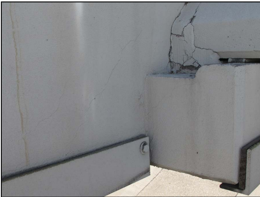
Figure A-52 - Shear crack and web ledge interface crack (a in Figure A-51)
