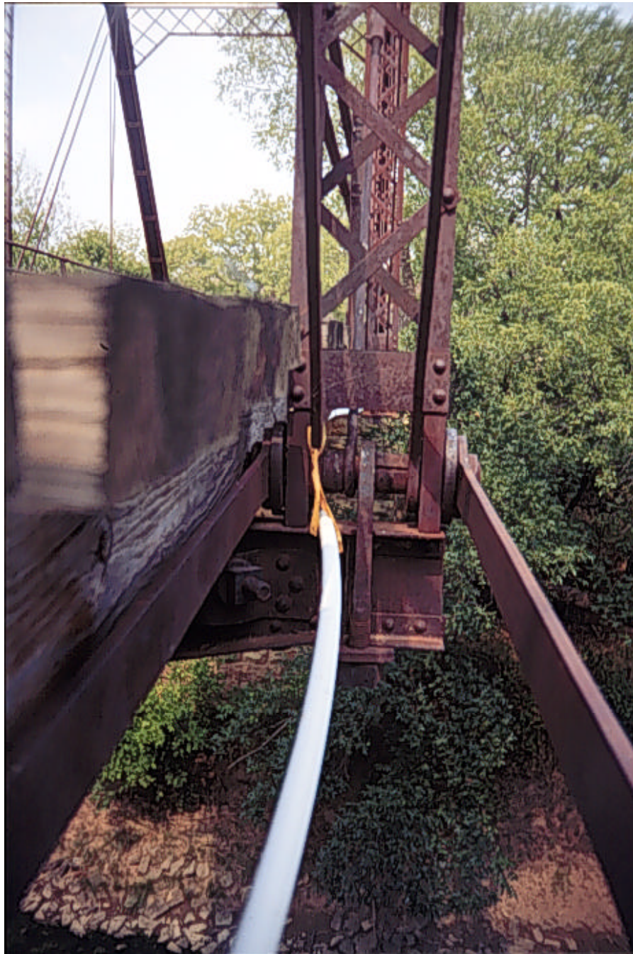
Photograph A.10: Details at bottom chord joints L2, L3, and L4
