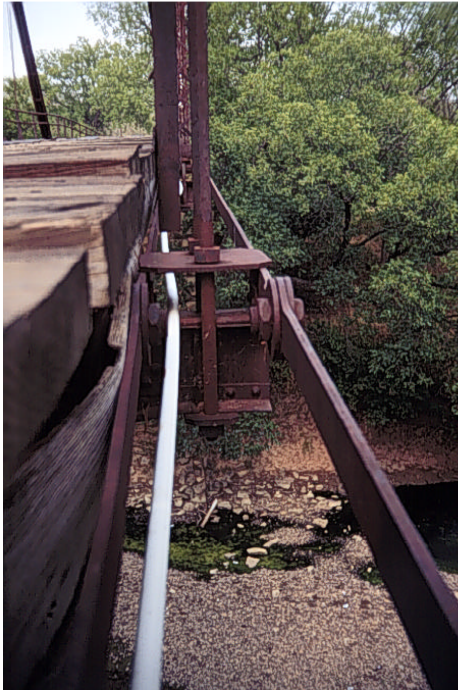
Photograph A.9: Details at bottom chord joints L1 and L5
