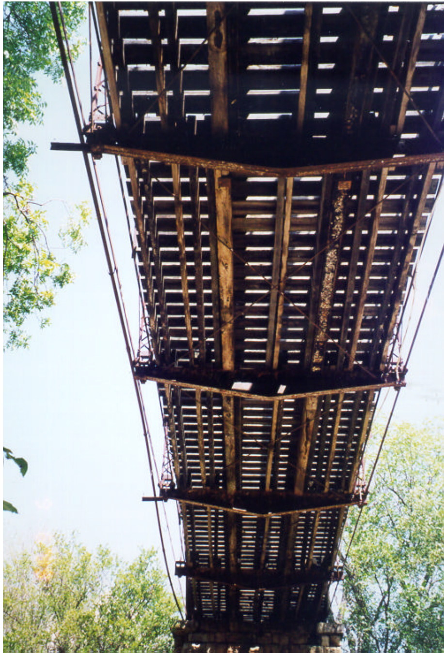
Photograph A.18: Details of bridge deck
