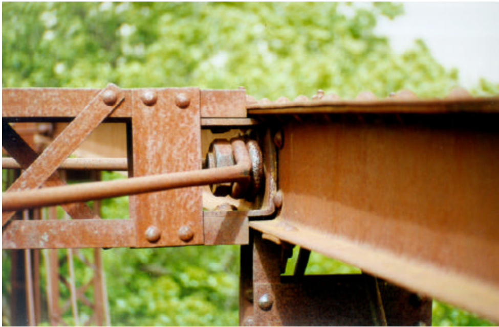
Photograph A.16: Details of top bracing connection
