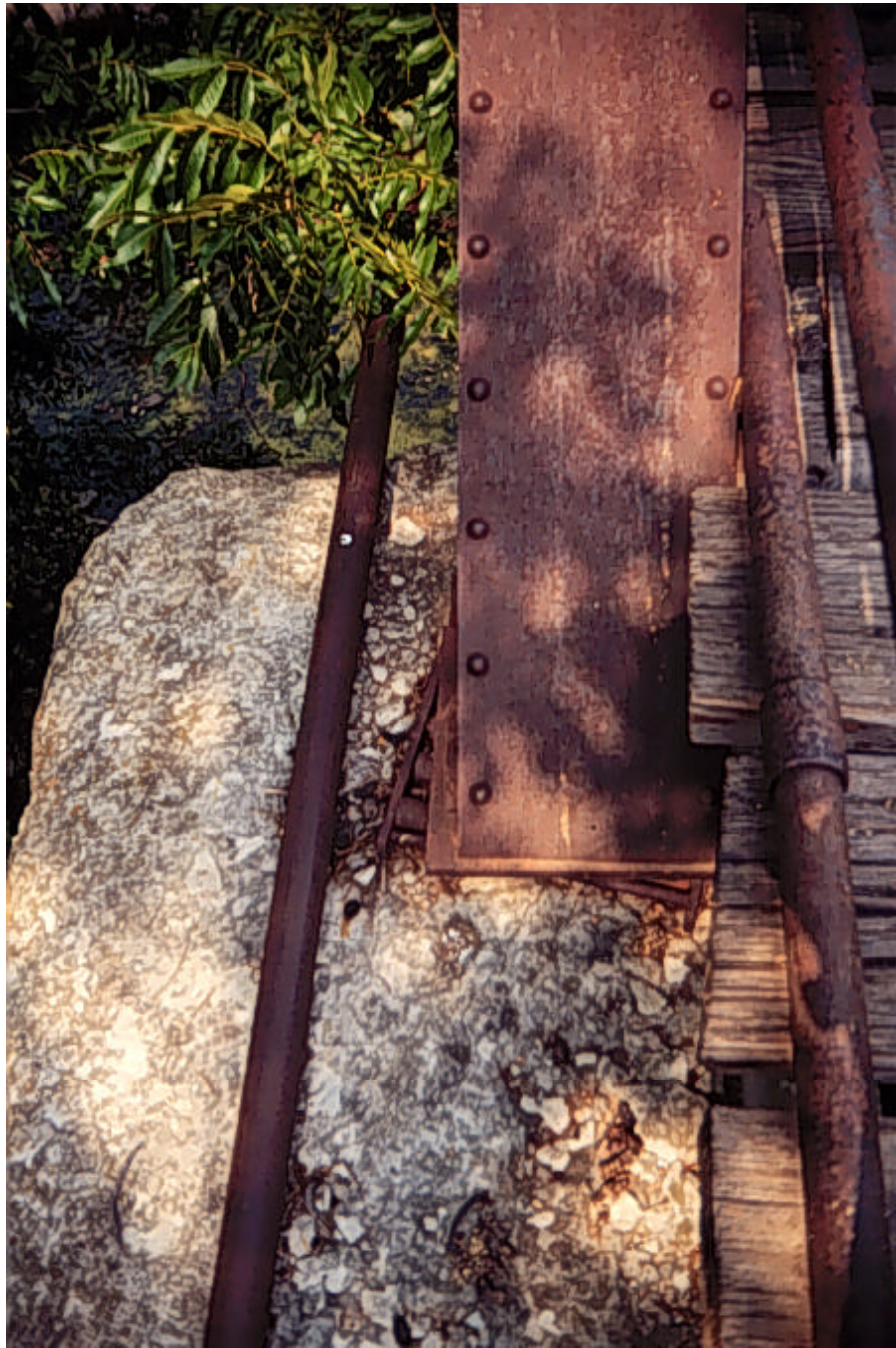
Photograph A.7: Details of the southwest roller support
