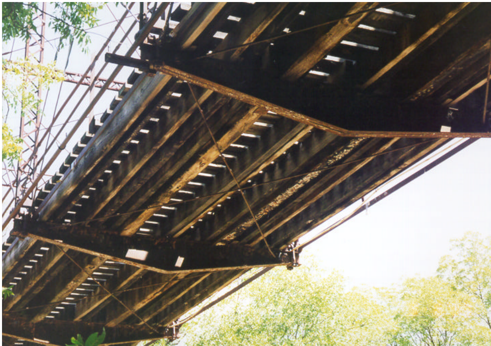
Photograph A.17: Details of bridge deck
