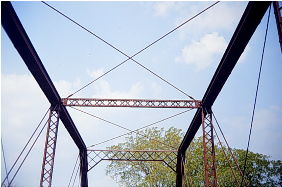
Photograph A.21: Details of the top lateral bracing system
