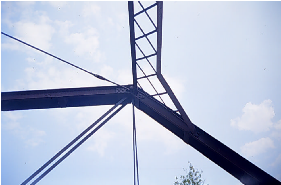
Photograph A.14: Details at upper chord joints U1 and U5
