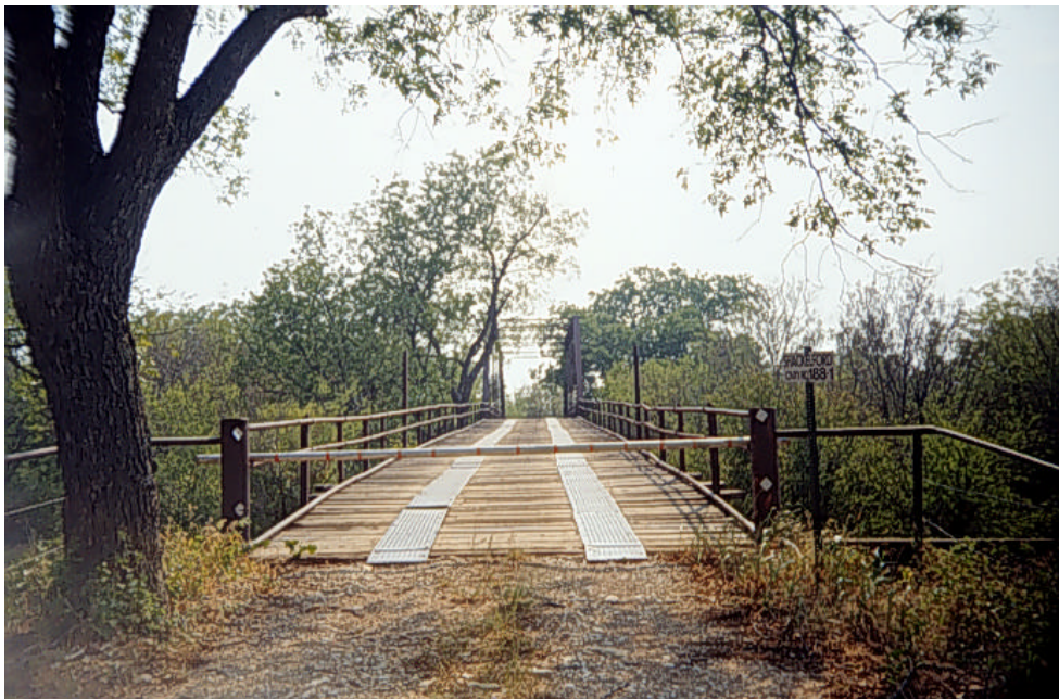
Photograph A.1: Case study bridge – looking towards south
