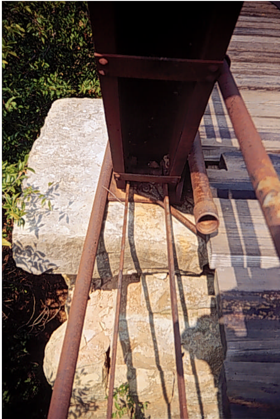
Photograph A.8: Details of the northwest hinge support
