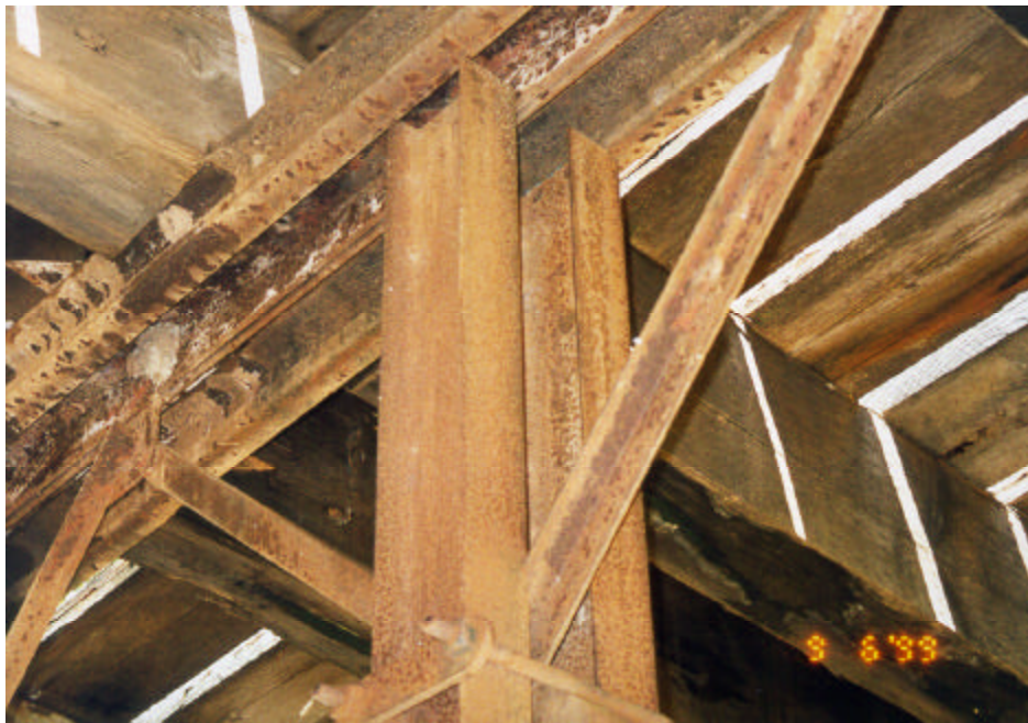
Photograph A.36: Details of metal bent for north approach span
