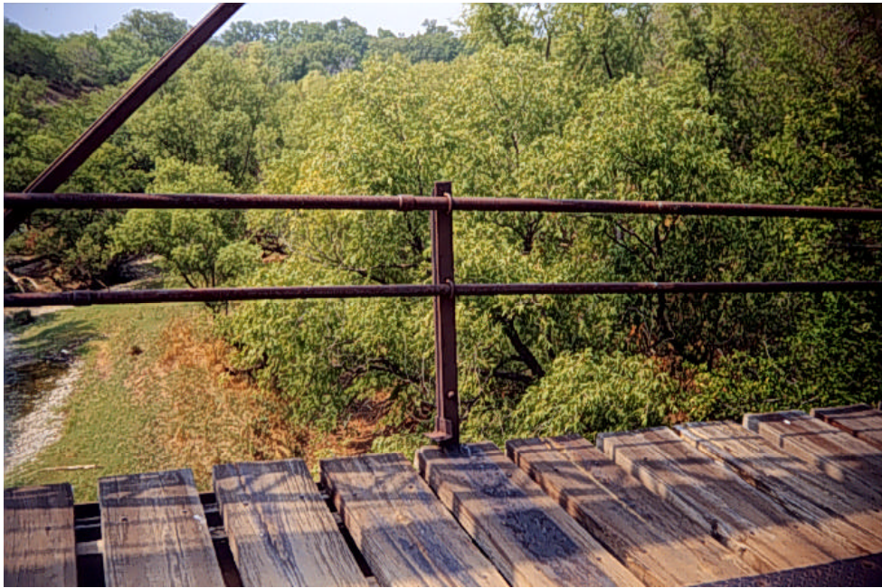
Photograph A.23: Details of metal railing
