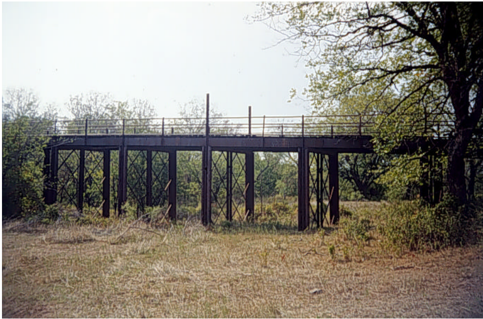
Photograph A.4: Side view of the north approach span
