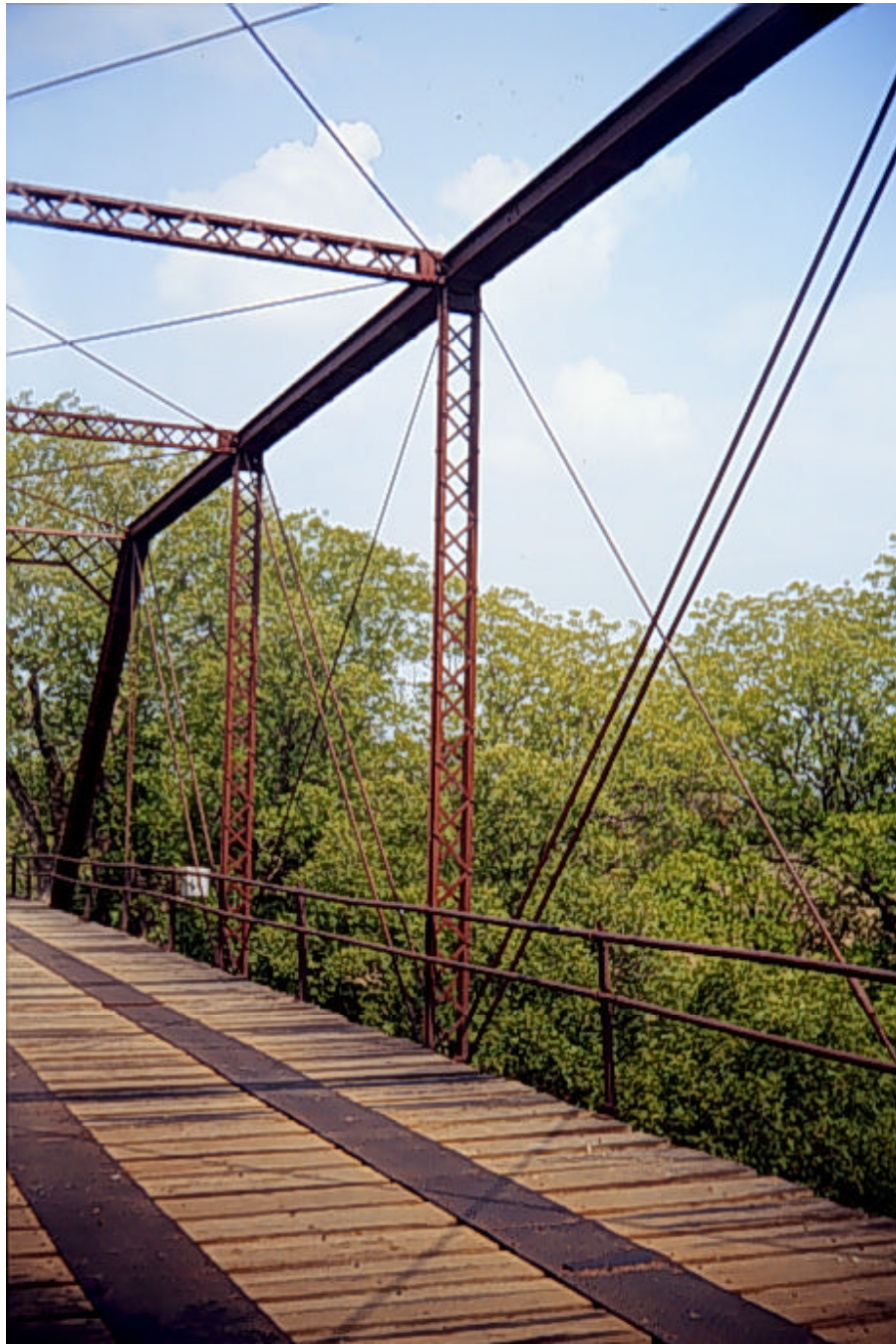
Photograph A.6: Details of the downstream truss
