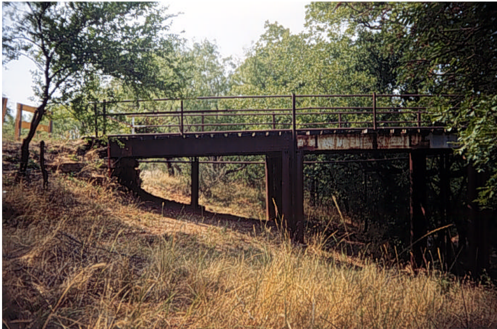
Photograph A.2: Side view of the south approach span
