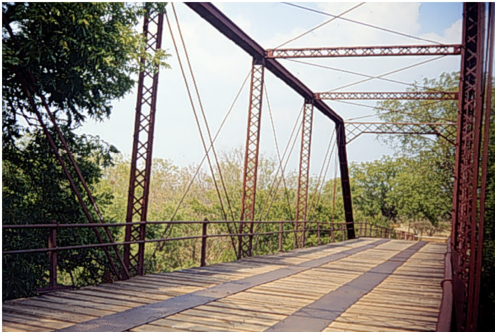
Photograph A.5: Details of the upstream truss
