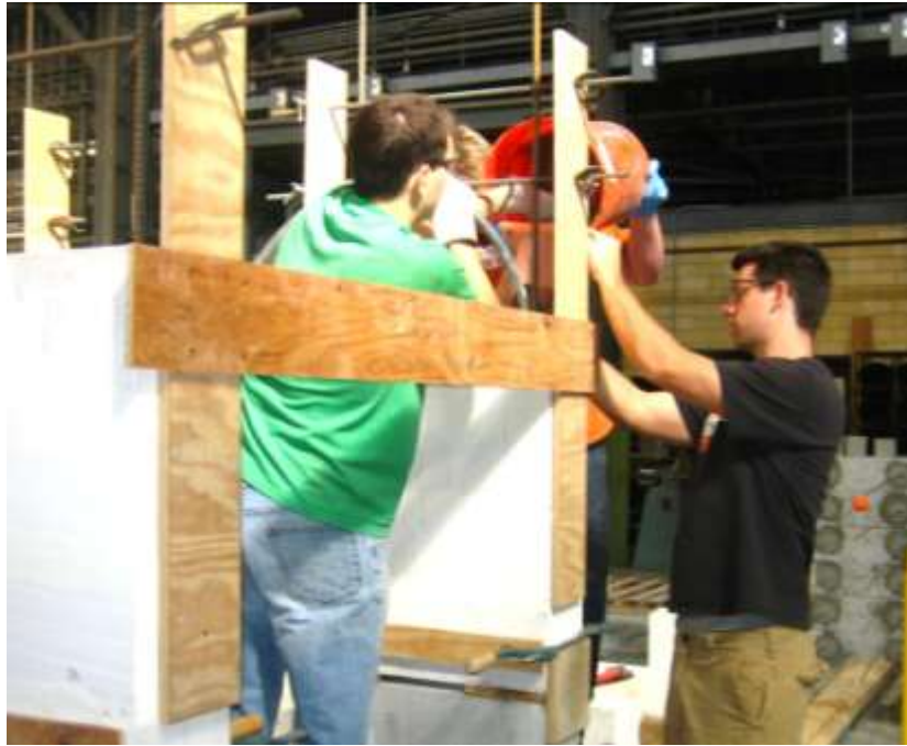
Figure 3.15 Grouting of lap-splice specimens with No. 5 bars
