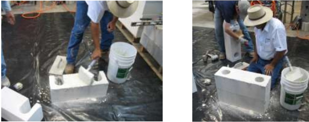
Figure 3.8 Construction of base-walls
