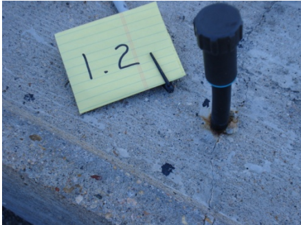
Figure 2.8: Rust Spots on Beam 1.2 and 2.2
