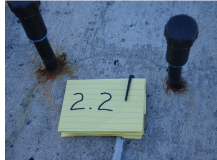
Figure 2.8: Rust Spots on Beam 1.2 and 2.2
