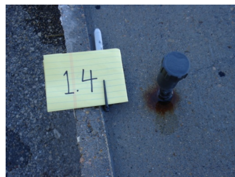
Figure 2.9: Rust Spots on Beams 4.1 and 1.4
