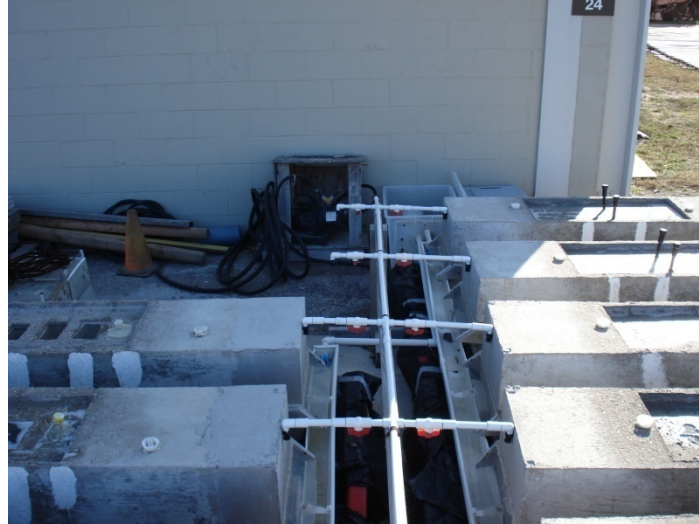
Figure 2.3: System Spraying Chloride Solution onto the Bearing Plates Beneath the Grout
