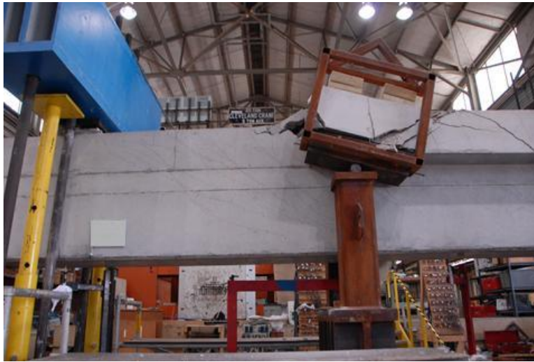
Figure D-53: Specimen after failure
