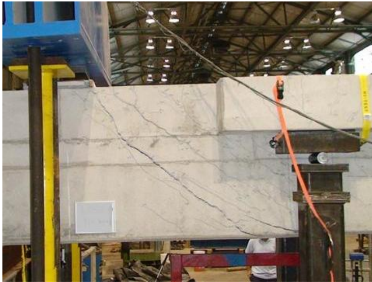
Figure D-13: Specimen after failure
