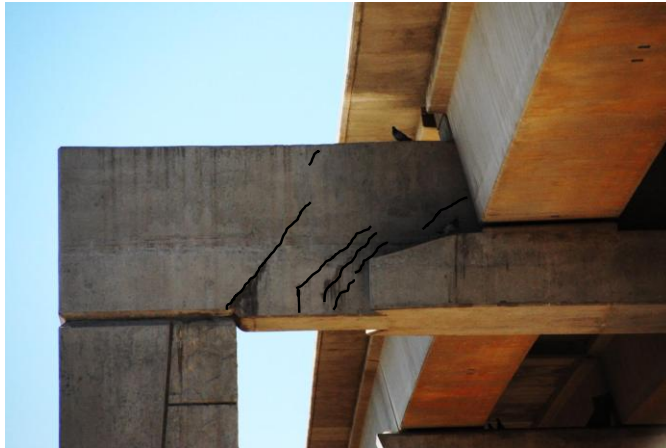
Figure 2-2: Simply supported bent cap in IH-35 / LP 340, Waco, TX.
