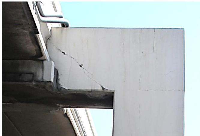
Figure 2-3: Partial moment connection bent cap in I-10/Geronimo, El Paso, TX.
