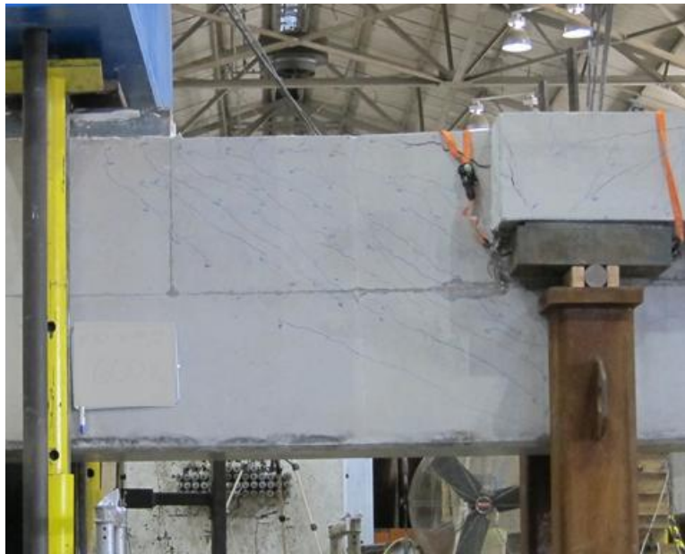
Figure D-59: Specimen after failure
