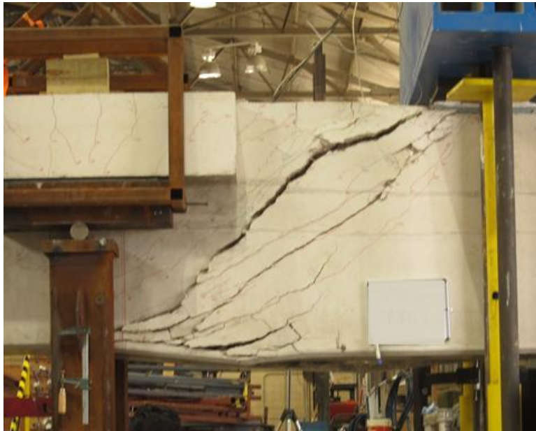
Figure D-45: Specimen after failure
