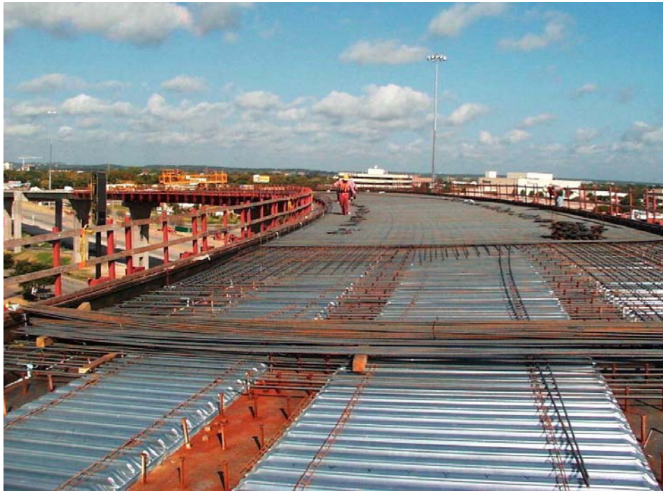
Figure 4.4: Deck Forms and Reinforcement Installation
