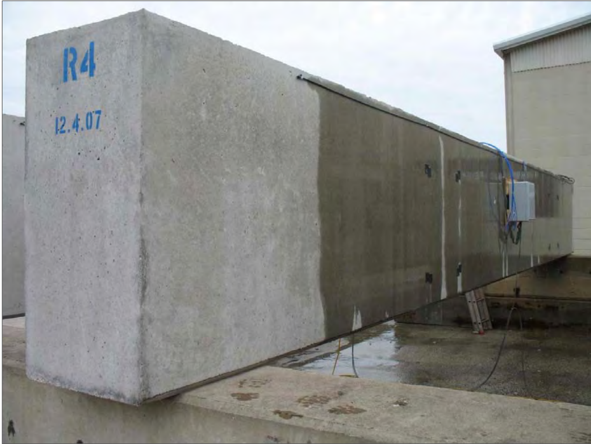
Figure 4-5: Demonstration of Watering System
