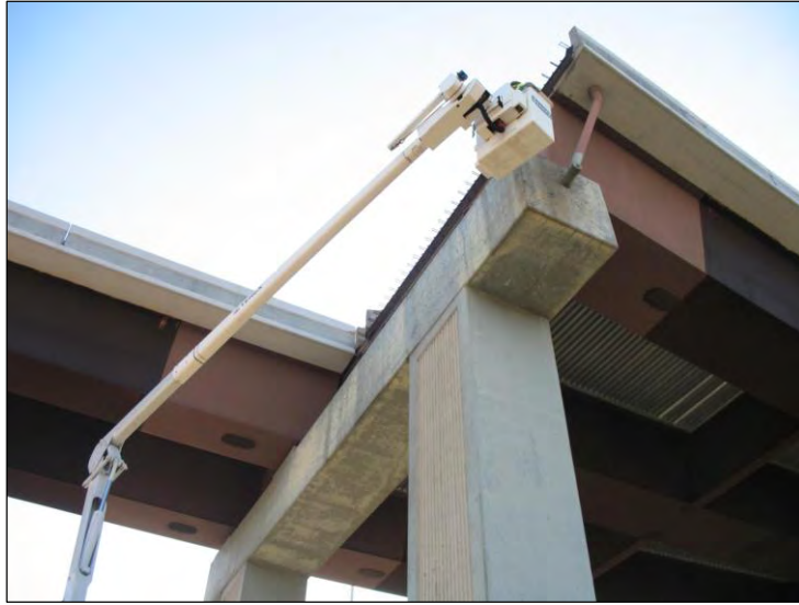
Figure 6-5: Bent 15 Inspection with Aerial Lift
