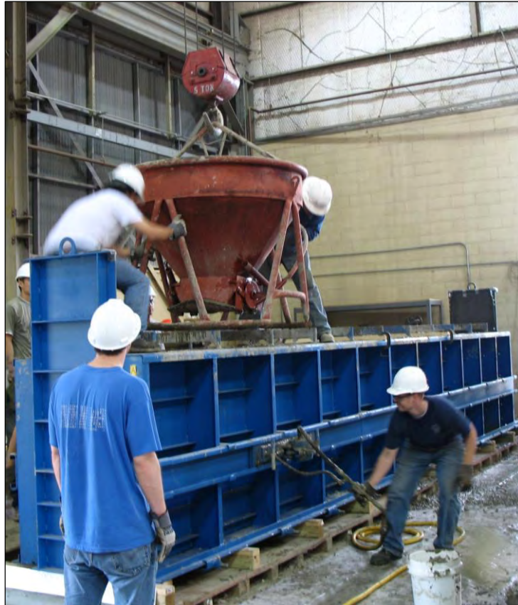
Figure 3-16: Concrete Placement and Form Vibration
