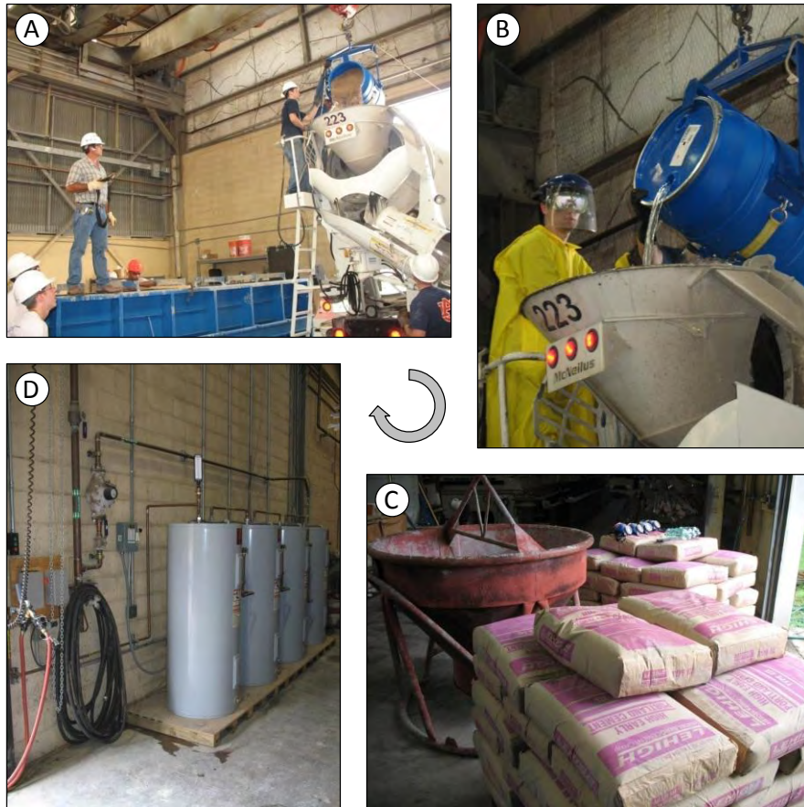
Figure 3-15: Concrete Materials Batching
