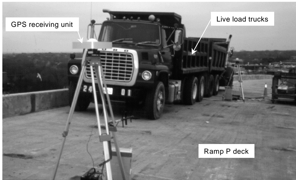
Figure 2.29 GPS deflection measurement equipment
