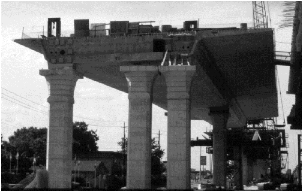
Figure 1.9 Cast-in-place transition spans
