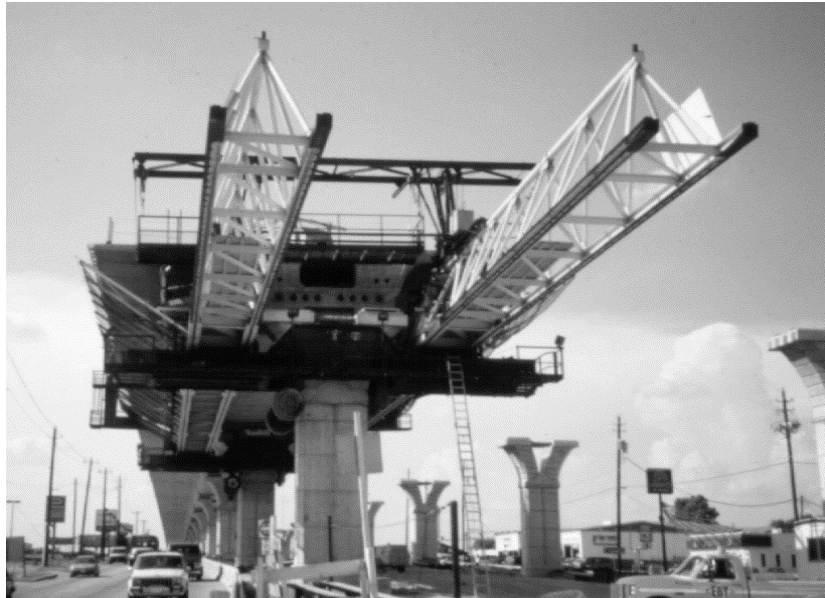
Figure 1.18 Construction of a mainlane girder
