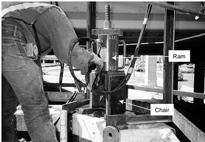
Figure 1.43 Hydraulic ram stressing temporary post-tensioning bars
