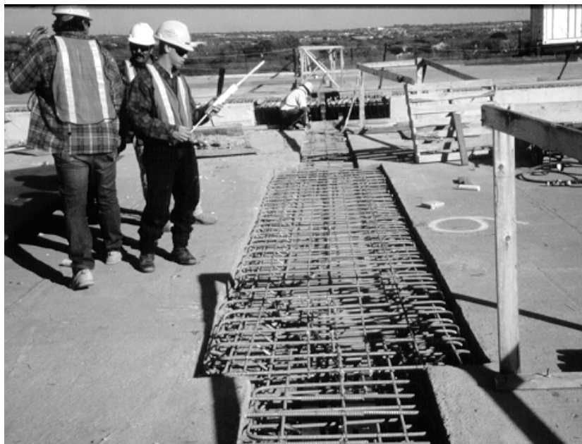
Figure 1.19 Construction of a cast-in-place deck joint
