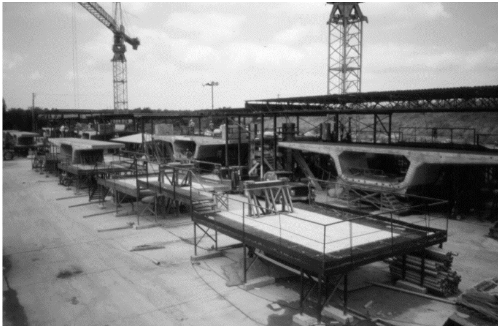
Figure 1.12 Casting machines
