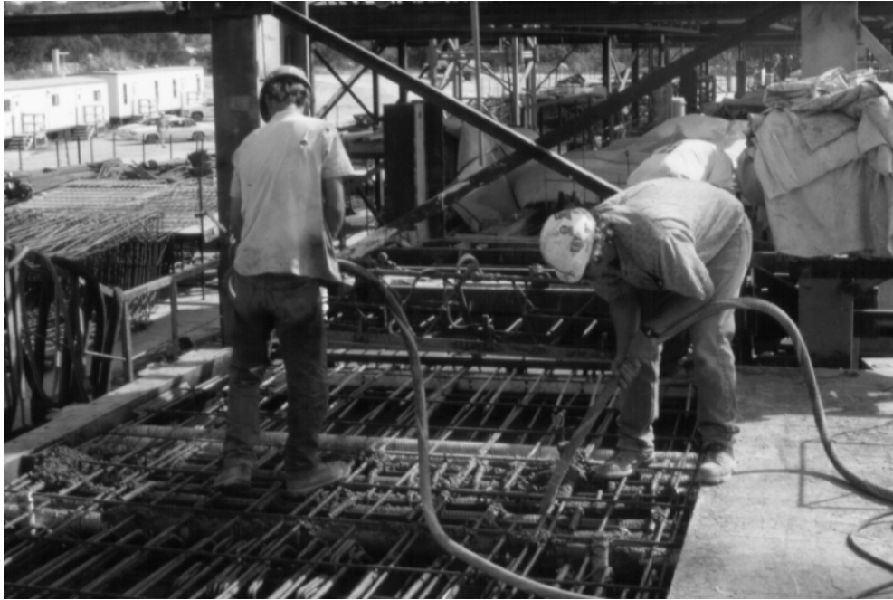
Figure 2.2 Vibrating concrete near instrumentation
