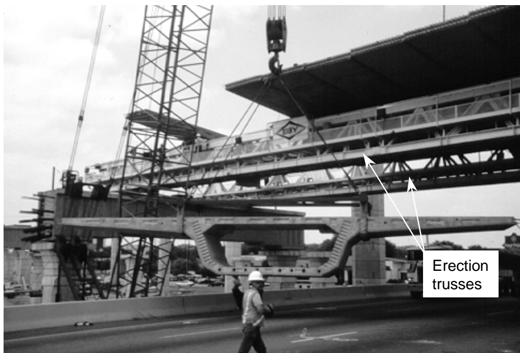
Figure 1.2 Span by span construction
