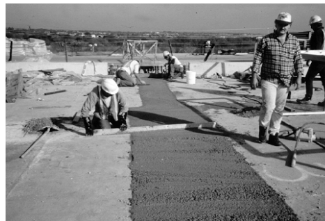
c). Deck joint concreting
