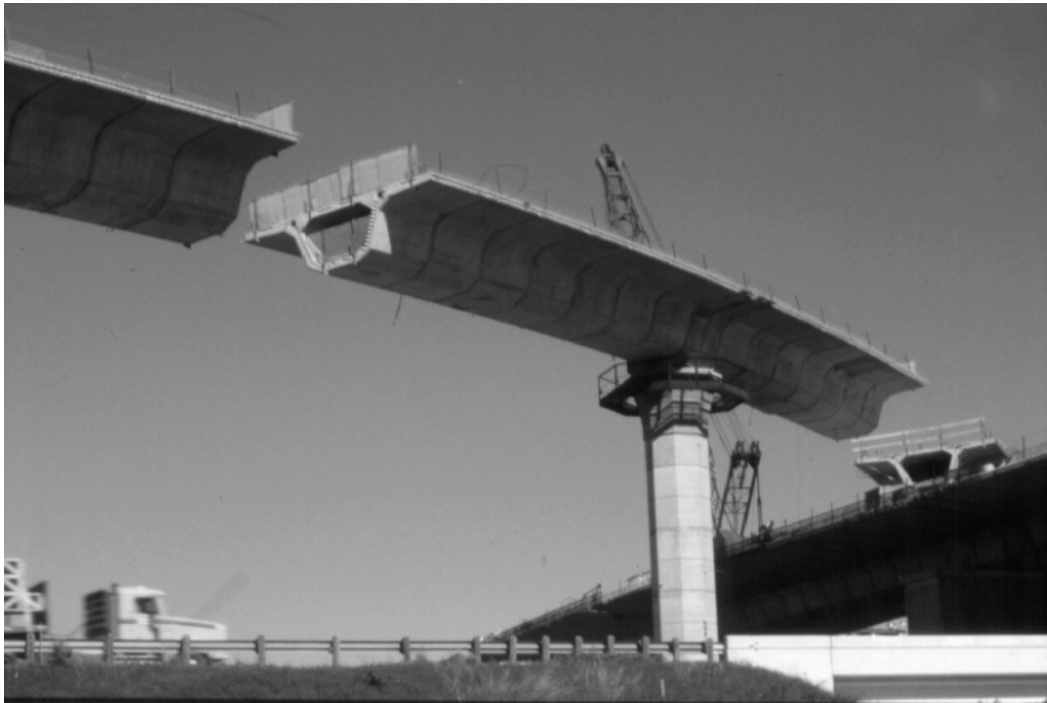
Figure 1.5 U.S. 183 North Ramp P constructed in balanced cantilever
