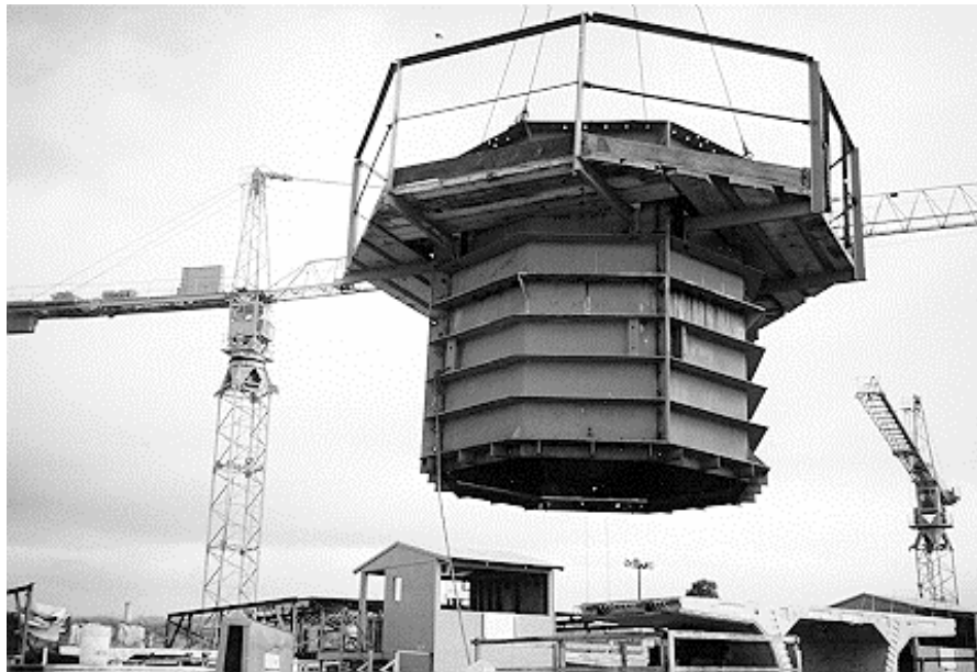
Figure 1.37 Placement of outer pier segment form
