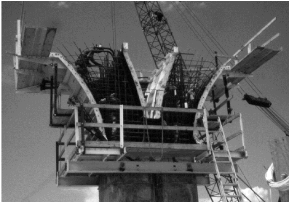
Figure 1.16 Construction of mainlane pier capital
