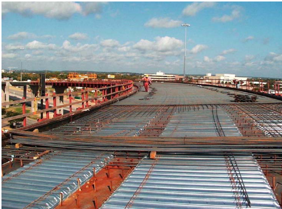
Figure 4.3 Deck Forms and Reinforcement Installation
