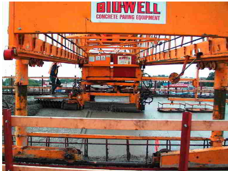
Figure 4.4 Concrete Screed
