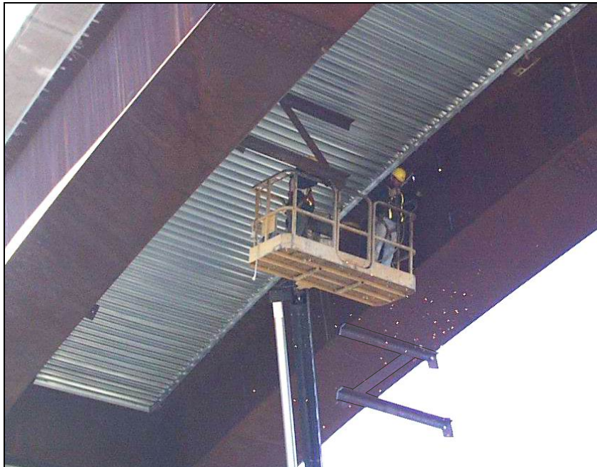
Figure 2.11 Flame Cut Removal of External Diaphragms
