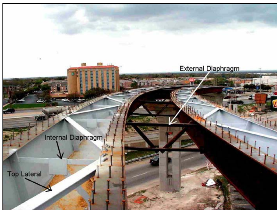
Figure 1.4 Picture of Z-Connect During Construction
