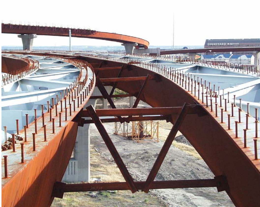
Figure 2.12 Installed External Diaphragm on K-Connect
