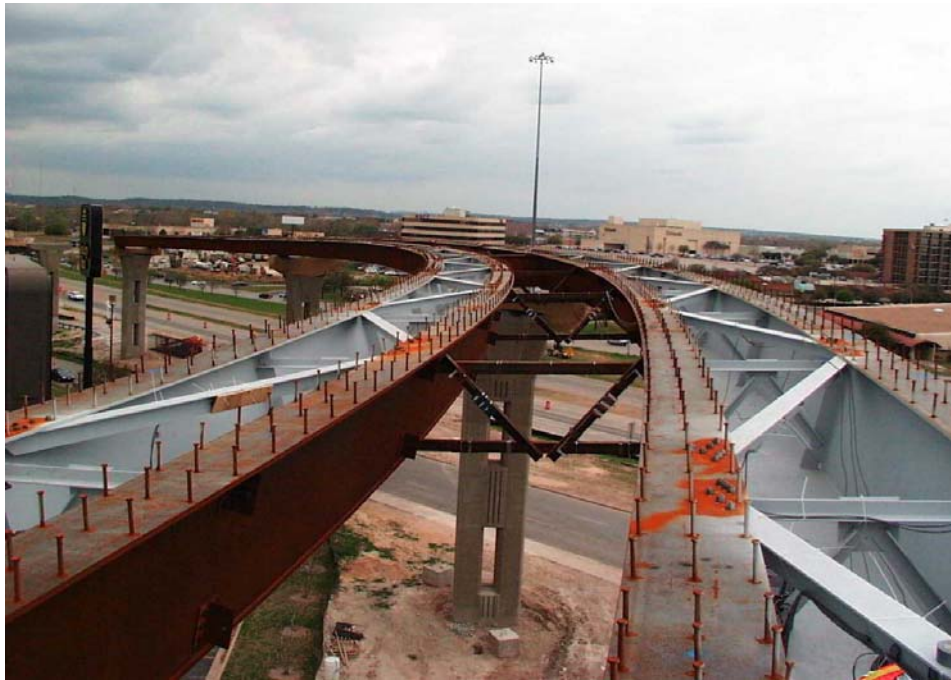
Figure 4.2 View of Z-Connect from Pier 16Z
