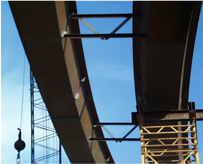
Figure 2.10 Installed External Diaphragms on Z-Connect
