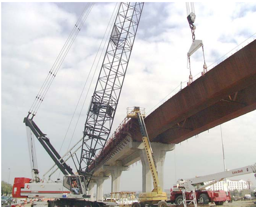
FIGURE 3.4 LOADING CRANE & TOP-FLANGE ATTACHMENT
