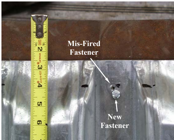
FIGURE 4.14 MIS-FIRED END FASTENER
