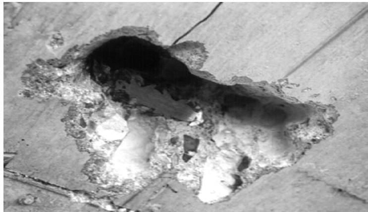
Figure 3.5 Reinforcing steel prepared for strain gage installation.
