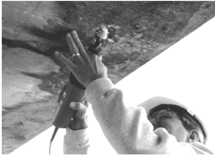
Figure 3.4 Grinding the rebar in preparation for strain gage installation.
