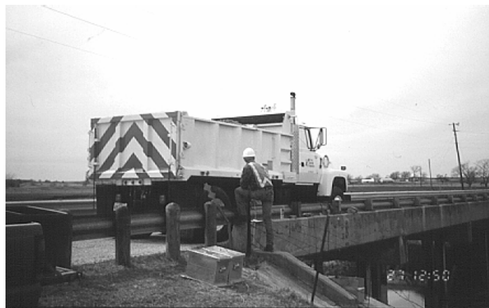
Figure 3.10 Load test in progress.
