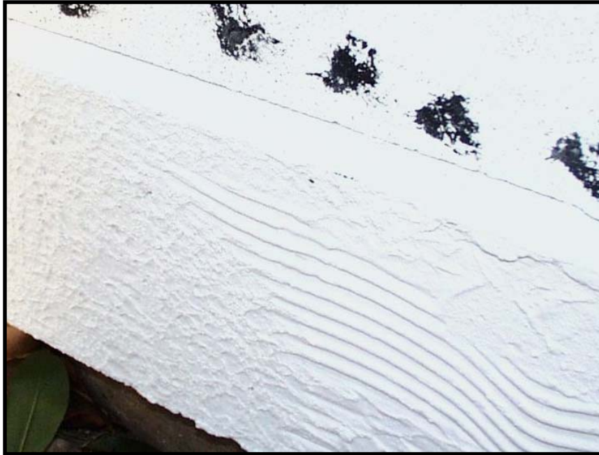
Figure 6-2: Typical vertical thin-bed mortar head joint in Shear Wall Pilot Specimen 1
