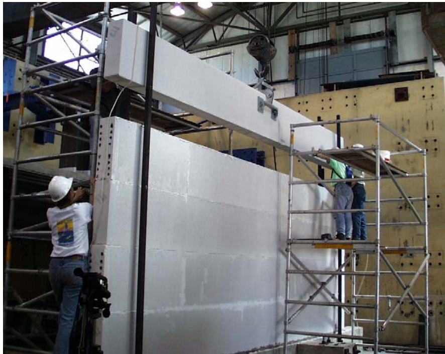
Figure 2-2: Placing horizontal panel during construction
