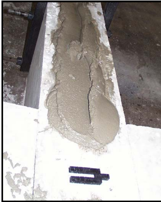
Figure 2-1: Combination of Type S mortar and thin-bed mortar on floor beam
