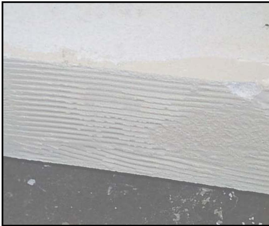
Figure 6-5: Typical vertical thin-bed mortar head joint in Shear Wall Pilot Specimen 2
