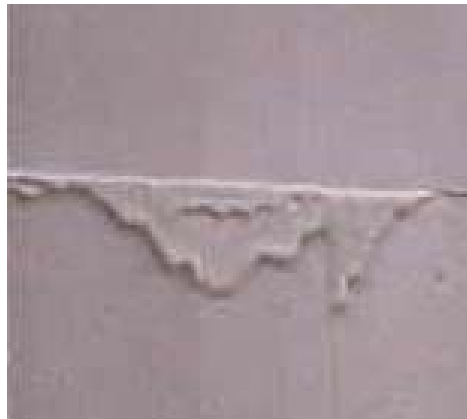
Figure 6-3: Excess thin-bed mortar squeezing out of a bed joint during construction
