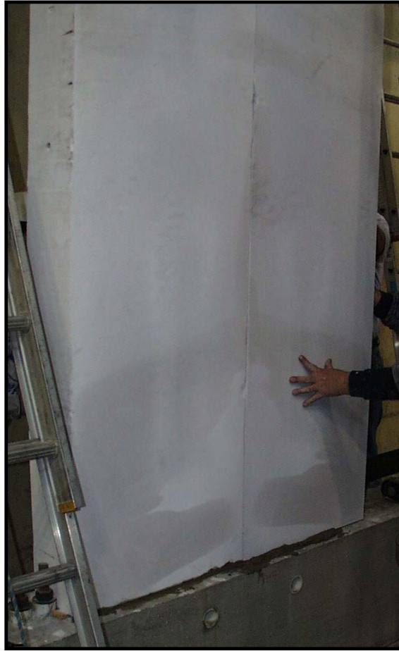
Figure 2-3: Placing vertical panels during construction
