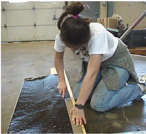
c) Applying epoxy to surface
