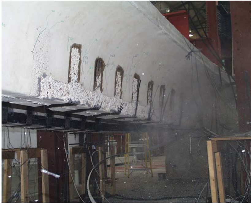
Figure 5.9 East Joist of Specimen J-1 at Failure
