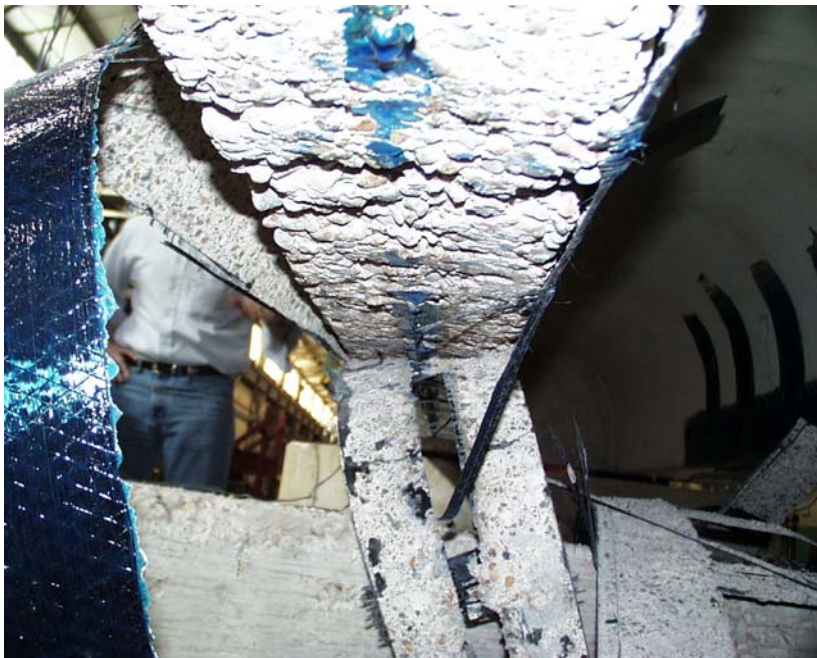
Figure 5.14 Bottom Surface Condition of West Joist after CFRP Debonding
