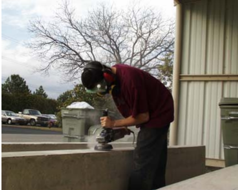
b) CFRP plate cleaning
