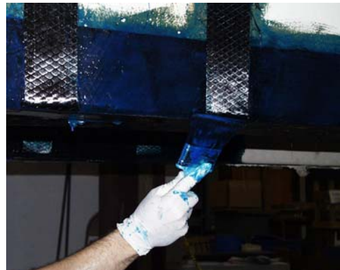
Figure C.4 Application of CFRP Wet-Layup System to Reinforced Concrete Element
