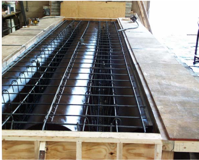
Figure 4.6 Specimen Reinforcement and Formwork
