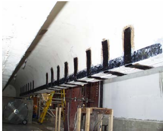
Figure C.3 Application of Woven Straps Around CFRP Pultruded Plates
