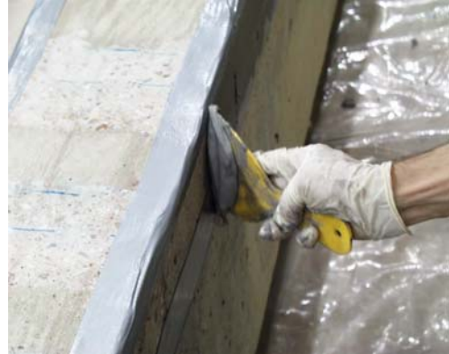
e) Positioning CFRP plate on beam
