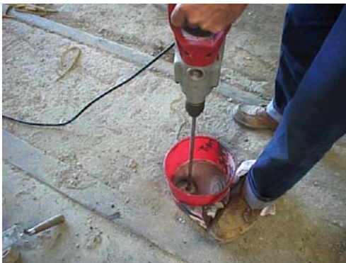
c) Mixing epoxy paste
