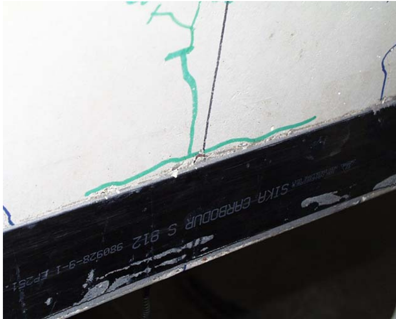
Figure 5.6 Observed Initial Debonding of CFRP Plate on East Joist
