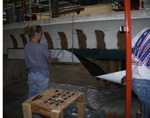
e) Eliminating air bubbles from sheets
