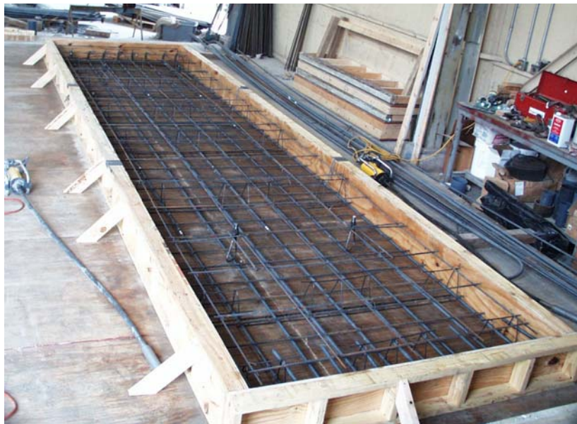
Figure 7.3 Picture Showing Reinforcement in a Typical Flat-Slab Specimen before Casting
