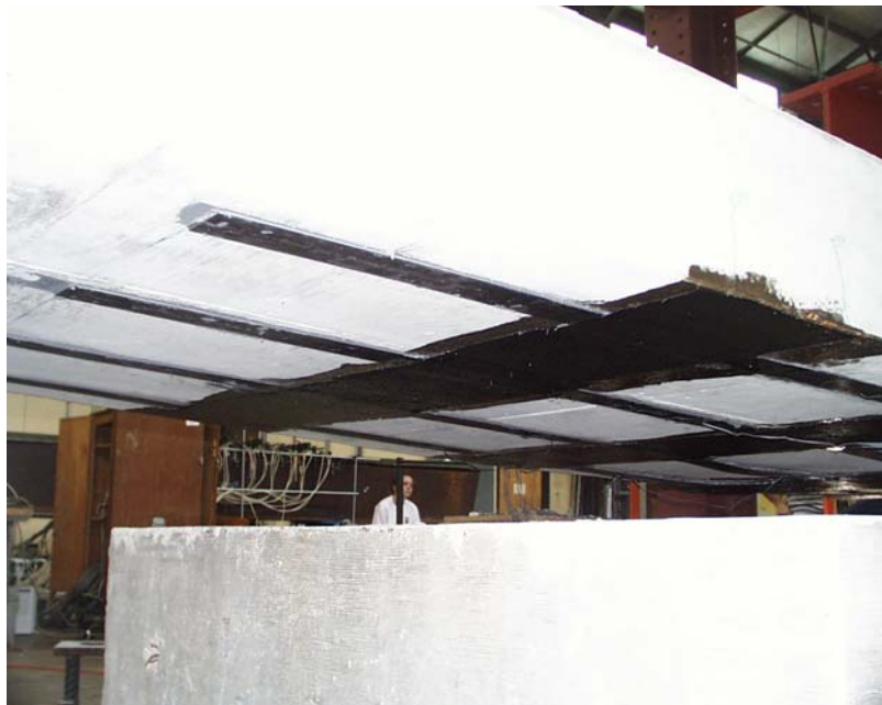
Figure 8.8 South End of the CFRP Plates Still Attached After Failure of Specimen FS-1
