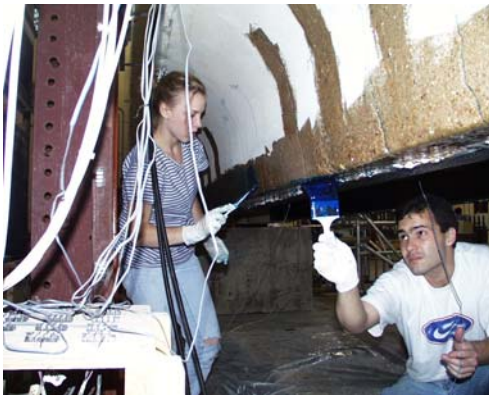
Figure C.4 Application of CFRP Wet-Layup System to Reinforced Concrete Element
