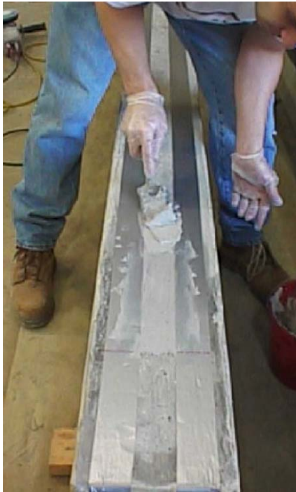
Figure 3.28: Epoxy Application to Concrete Surface
