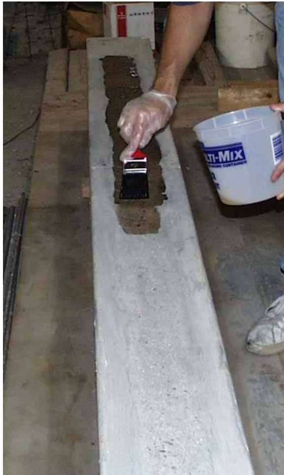
Figure 3.17: Application of Primer
