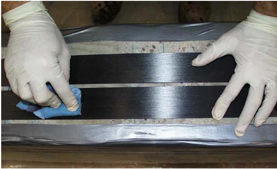
Figure 3.26: Cleaning Composite
