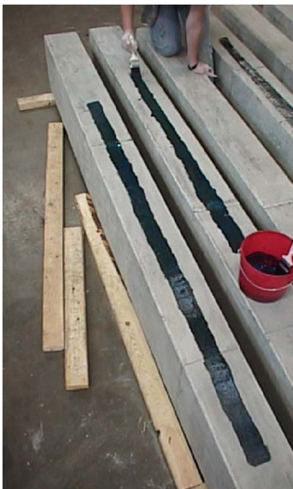
Figure 3.19: Wet Lay-up Method 1 Epoxy Application
