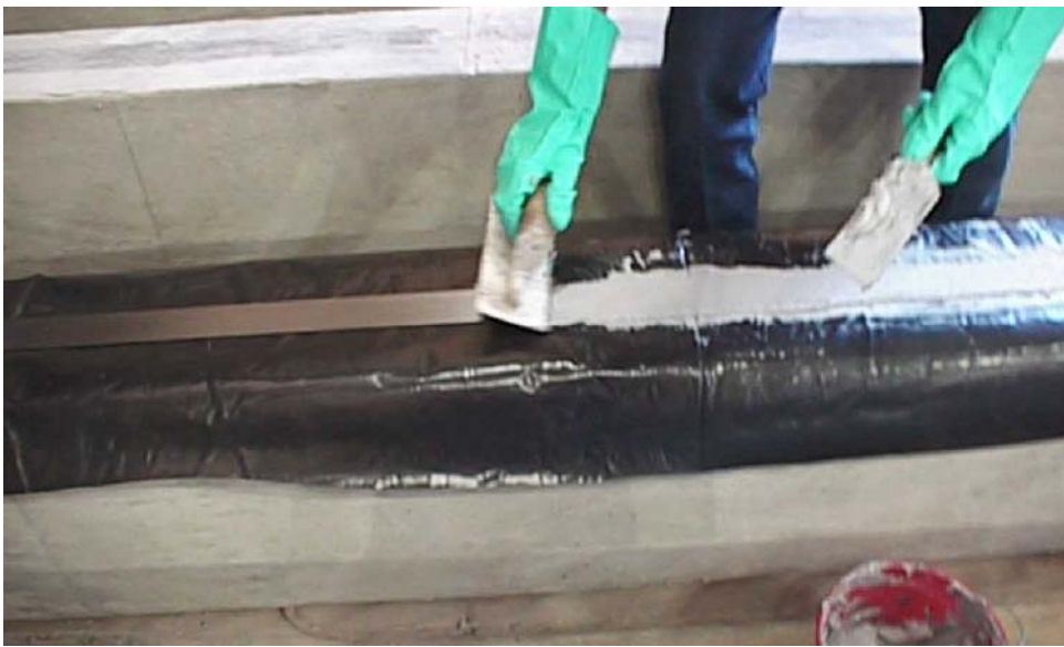
Figure 3.27: Epoxy Application to Composite
