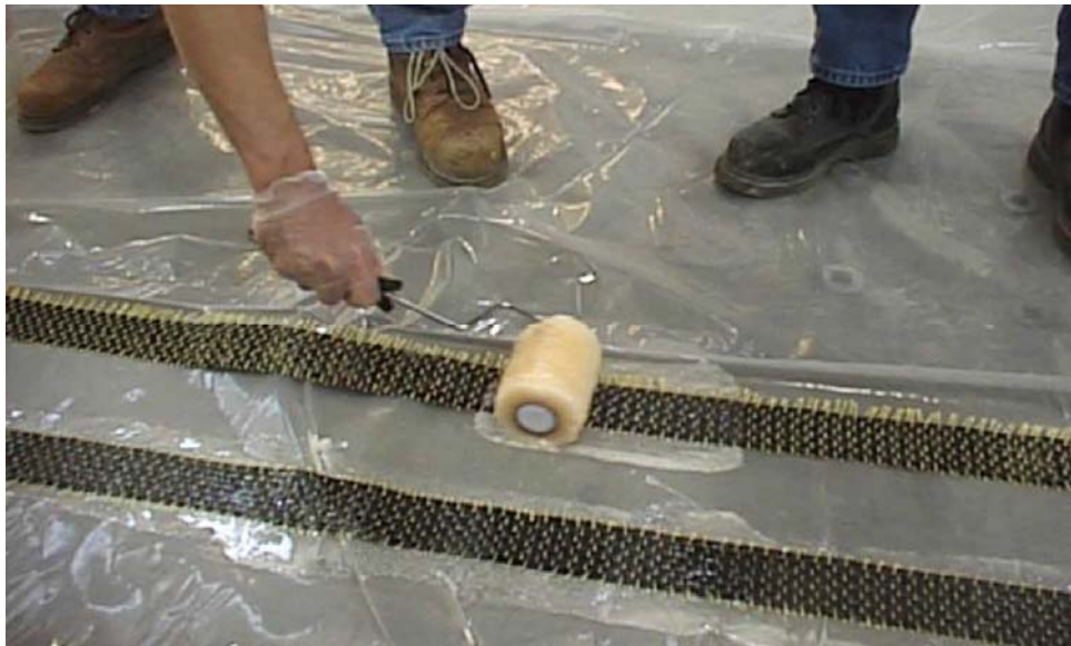
Figure 3.22: Wet Lay-up Method 2 Fiber Saturation
