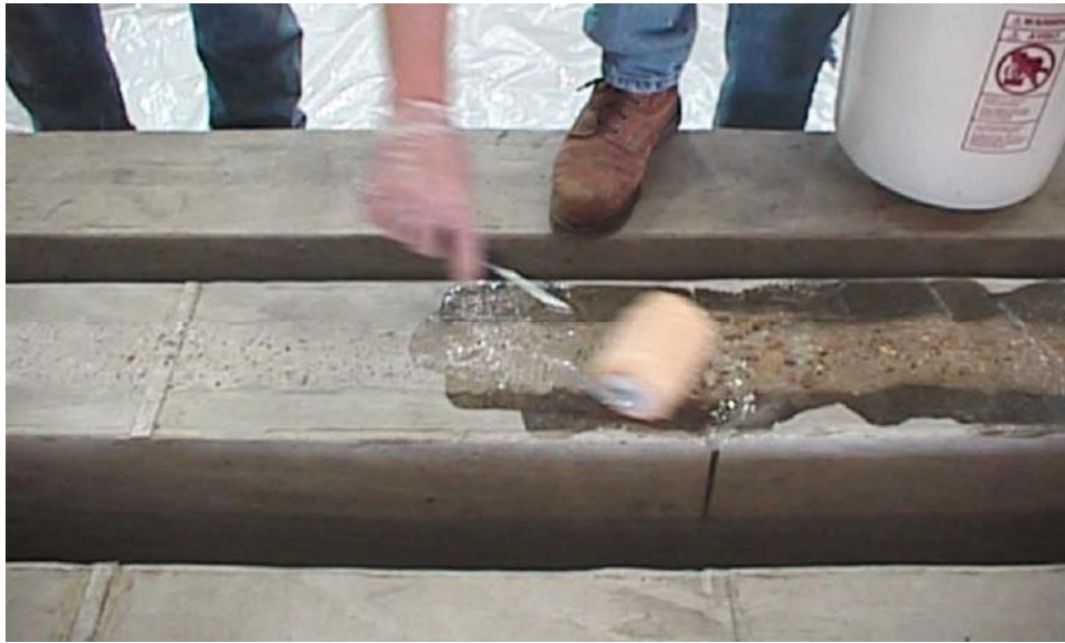
Figure 3.21: Wet Lay-up Method 2 Epoxy Application
