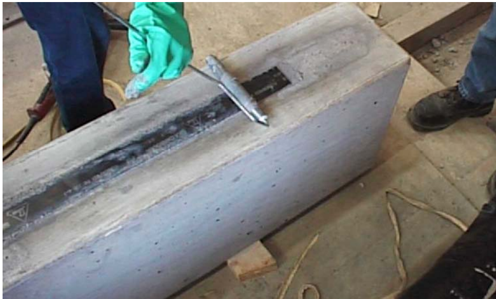
Figure 3.30: Rolling Composite to Remove Excess Epoxy and Air Voids
