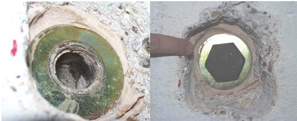
Figure 6.15: Specimens HTFAT01 and HTFAT02 with epoxy
