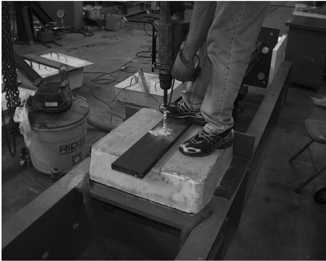
Figure 5.19: Drilling into concrete with rotary hammer drill (Hole predrilled in plate)
