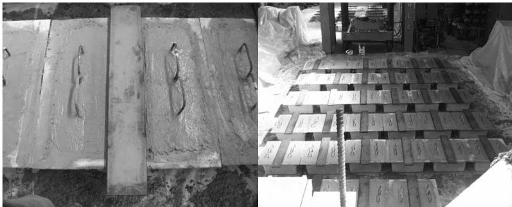
Figure 5.5: (a) Steel plate placed into position; (b) Completed pour
