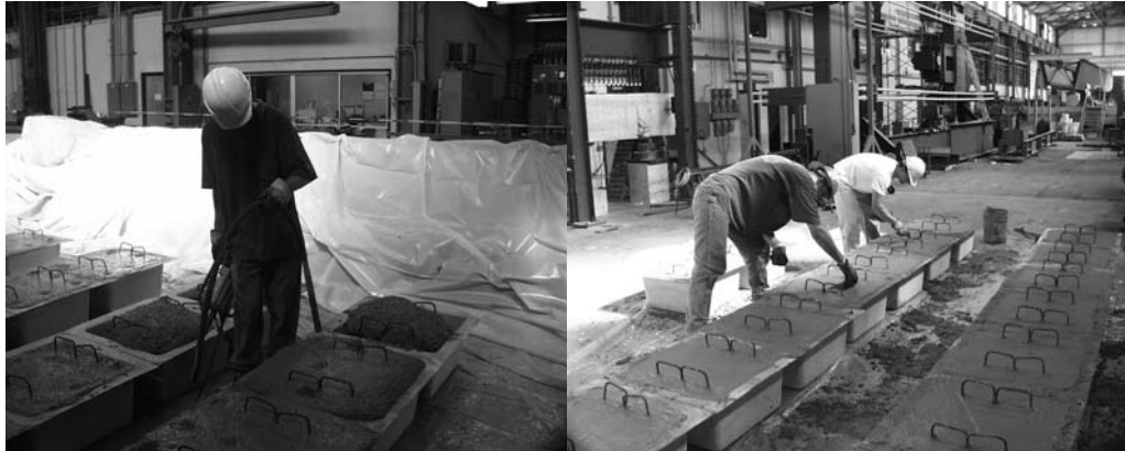
Figure 5.4: (a) Pouring and vibrating concrete; (b) Finishing concrete
