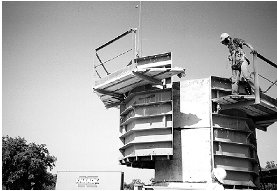
Figure 4.11: Removal of outer formwork.
