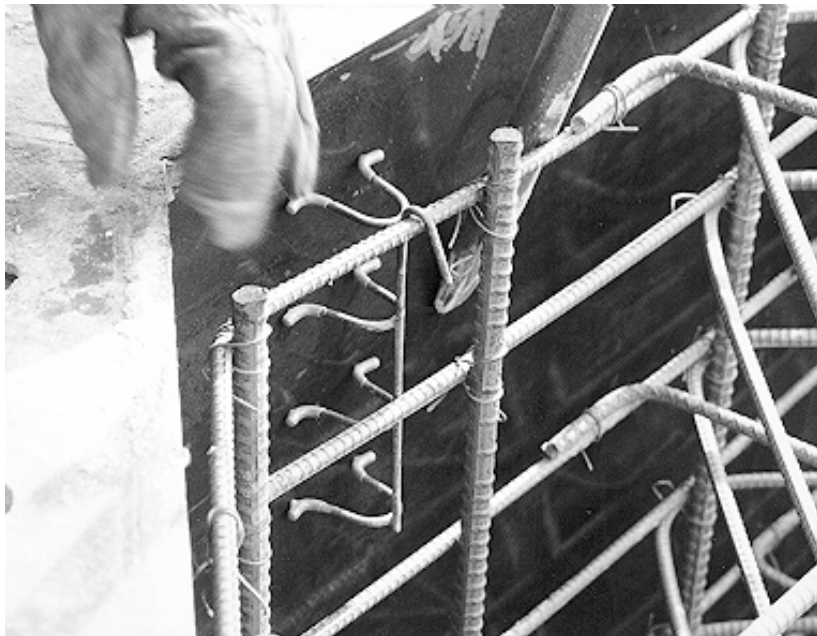
Figure 4.10: Rebar chair used to ensure adequate clear cover.
