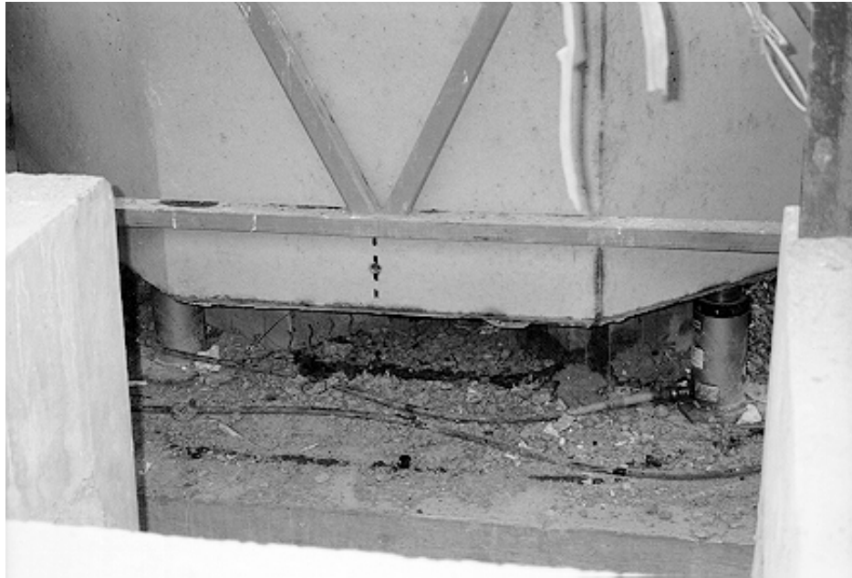
Figure 4.5: Hydraulic jacks used to align the bulkhead pier segment.
