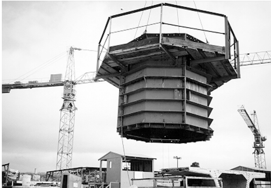
Figure 4.8: Pier segment outer form and scaffolding.
