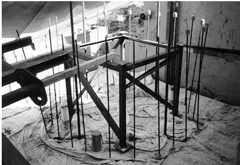
Figure 4.13: Steel support frame for segment prior to cast-in-place base construction.
