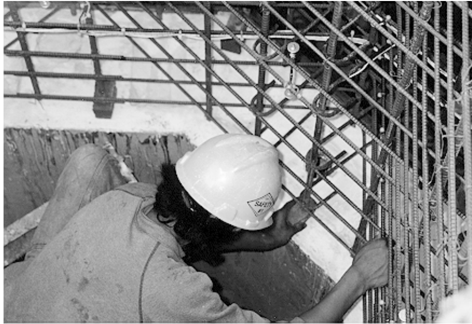
Figure 4.9: Placement of 50 mm thick cinder blocks under reinforcement cage.
