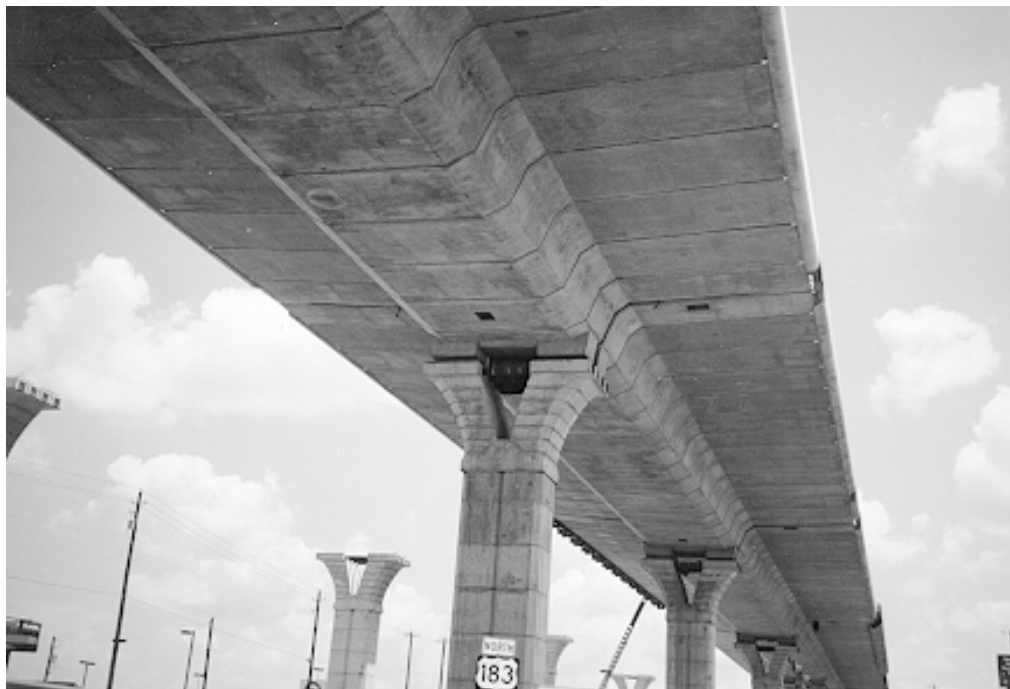
Figure 1.2: U.S. 183 viaduct mainlane superstructure.
