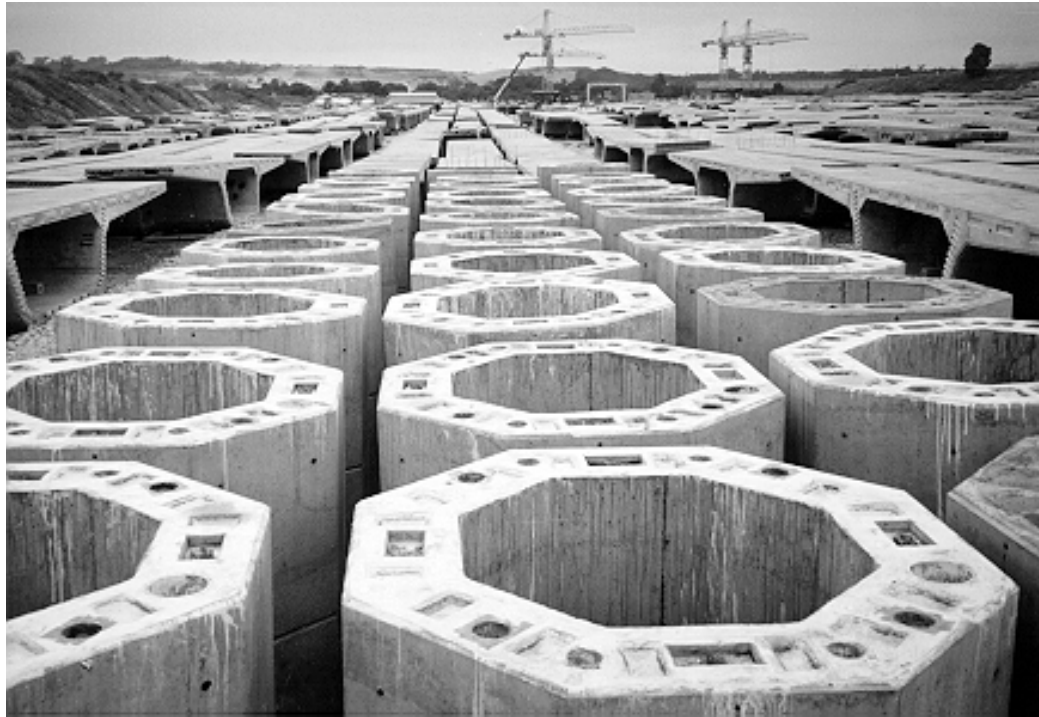
Figure 4.2: Completed pier segments in storage at the casting yard.
