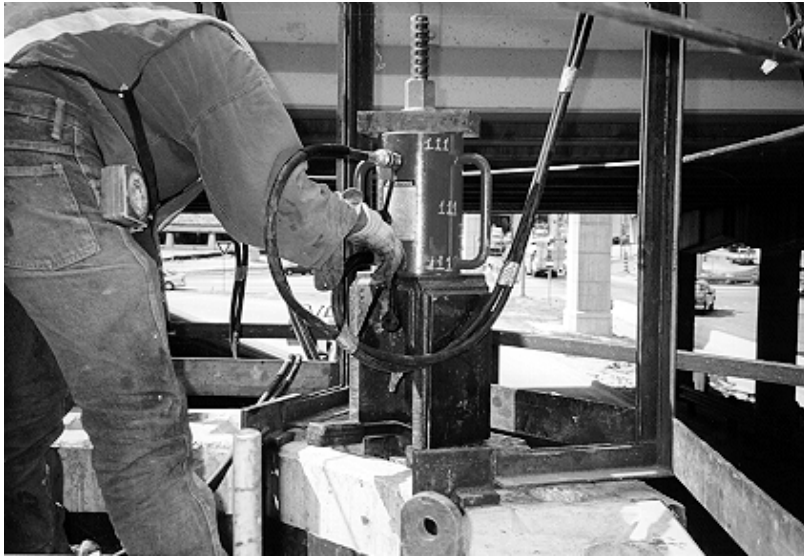
Figure 4.15: Hydraulic ram stressing temporary post-tensioning bars.
