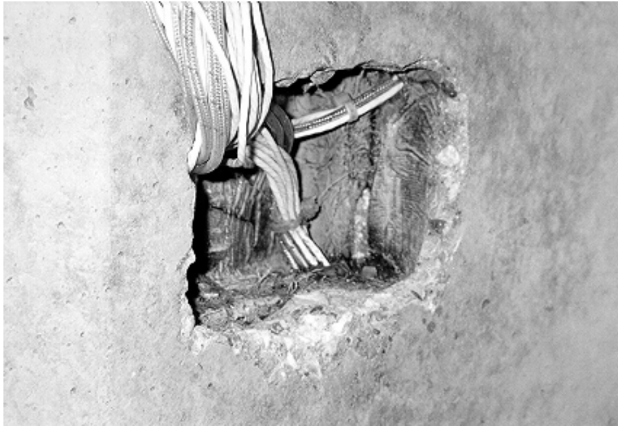
Figure 3.11: Blockout and instrument wires after casting, base segment PC16-1.
