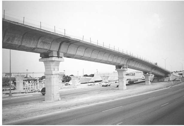
Figure 1.3: Typical access ramp superstructure.
