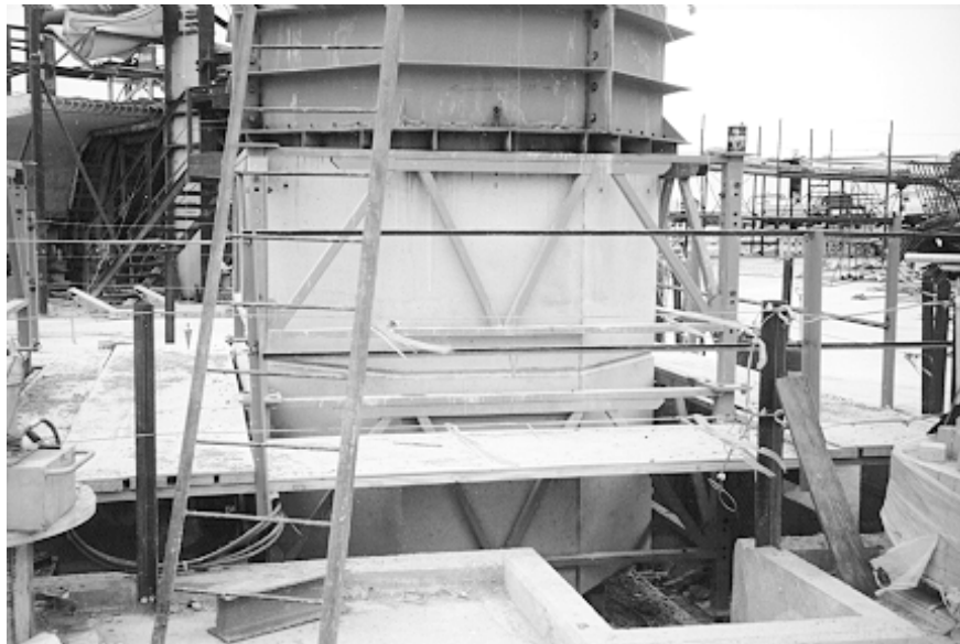
Figure 4.4: Casting bed with steel support frame for formwork.
