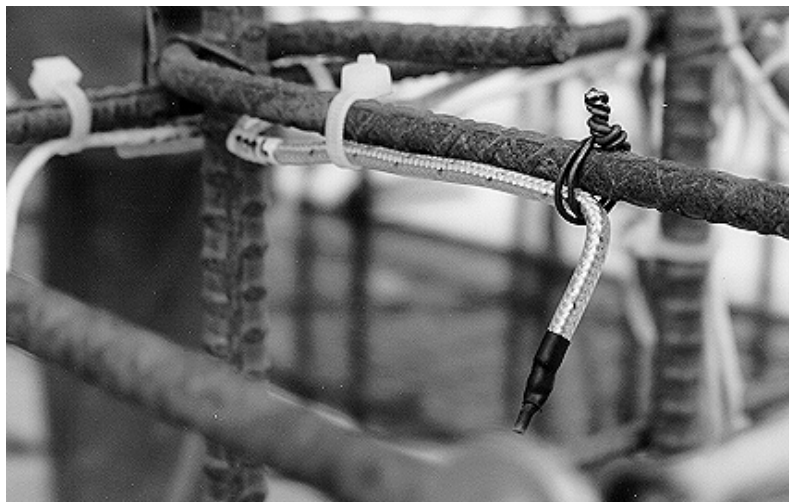
Figure 3.13: Typical thermocouple placement in rebar cage, base segment PC16-1.
