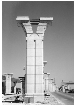
Figure 2.17: Unusually-shaped mainlane pier, U.S. 183 segmental viaduct.
