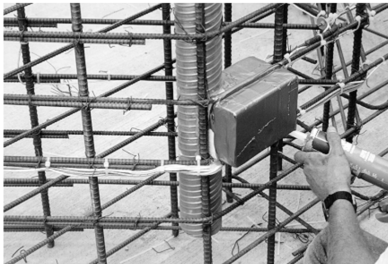
Figure 3.10: Access blockout and conduit for gauge wires, base segment PC16-1.
