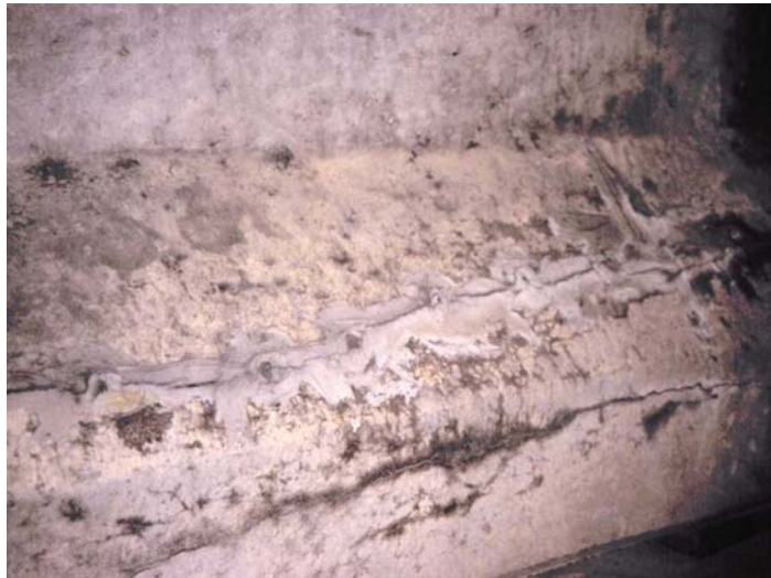
Figure 7.3 Injected sealant on I-10 structure
