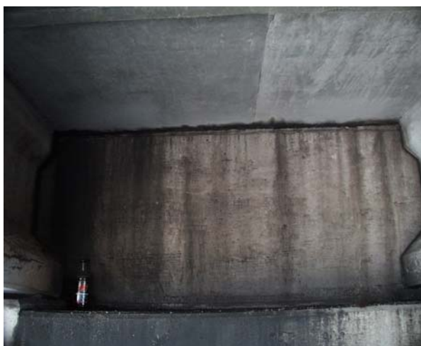
Figure 7.5 View of west abutment between SW Girder 2 (left) and SW Girder 3 (right)
