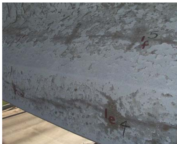
Figure 7.21 Marked points on Faces 4 and 5 at Location 2
