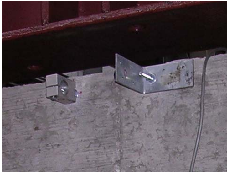
Figure 4-6: Aluminum clamp and angle before DCDT installation
