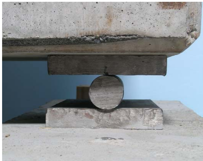
Figure 4-10: Roller support condition at one end of full-scale girder
