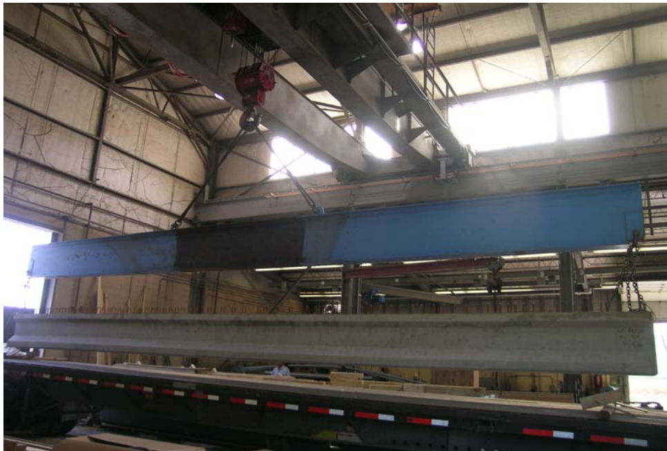
Figure 3-10: Lifting a Type-A girder from a flatbed truck in FSEL
