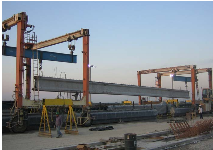
Figure 6-2: Transportation of a Type-IV girder at HEI San Marcos plant
