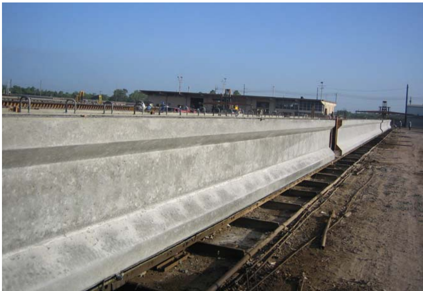
Figure 6-5: Line of Type-IV girders after release at TCC Victoria plant
