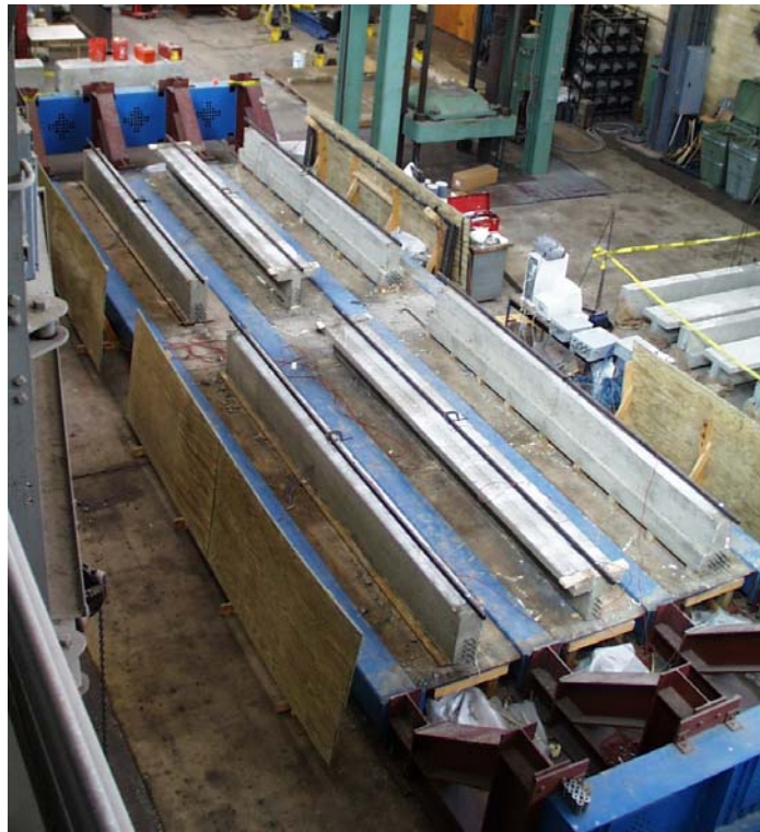
Figure 3-5: Prestressing bed with rectangular, tee, and inverted-tee beams (photograph courtesy of Alfredo Castro)
