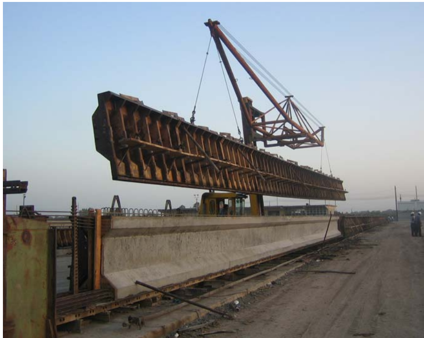
Figure 6-3: Form removal for a line of Type-IV girders at TCC Victoria plant
