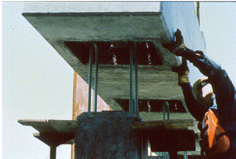
Figure 1.6 Lowering Precast Cap over Dowels onto Piles
