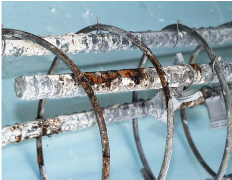
Figure 6.16 Steel reinforcing of CNC10 with a corrosion rate of 3.86 mpy.
