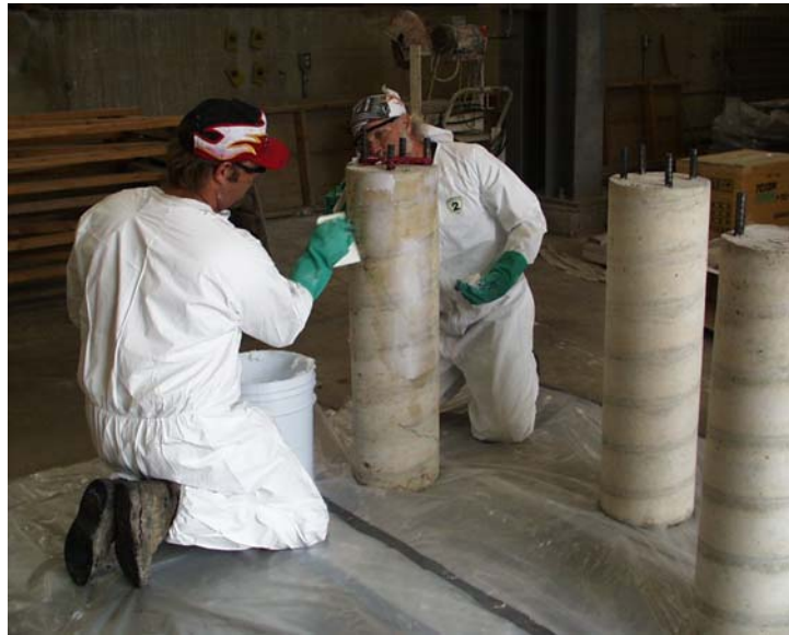
Figure 8.2 Filling voids with a thickened epoxy filler.
