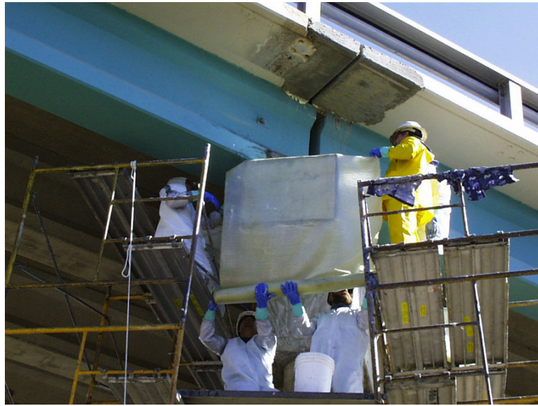
Figure 3.1 FRP composite wrap being applied to the bent of a bridge.
