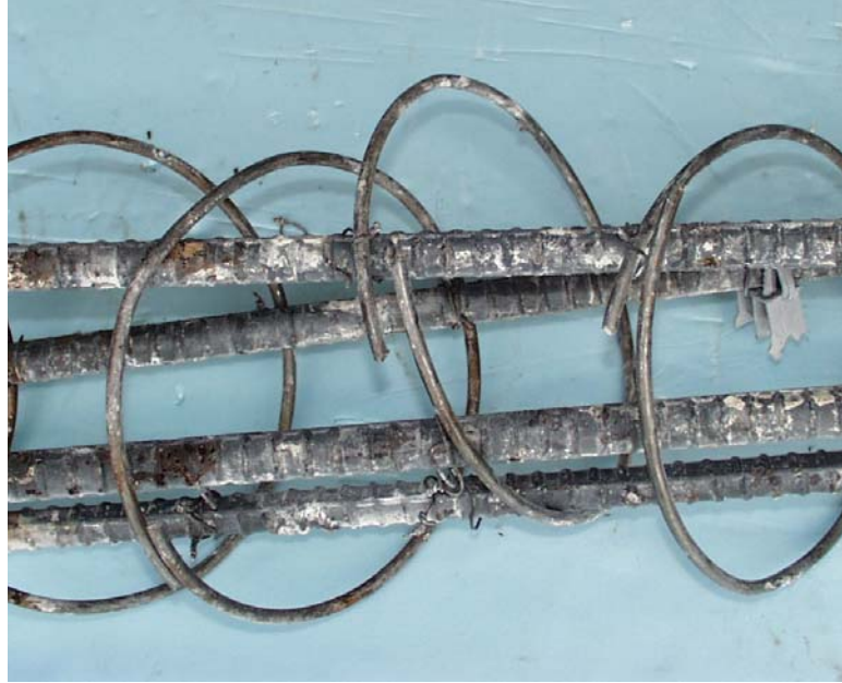
Figure 6.18 Steel reinforcing of CC3 with a corrosion rate of 0.34 mpy.
