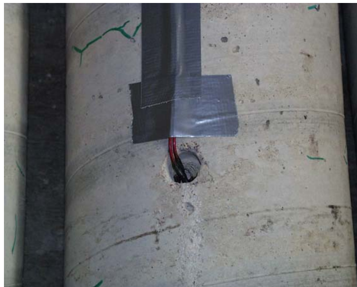
Figure 8.6 Installation of the embedded reference electrodes.
