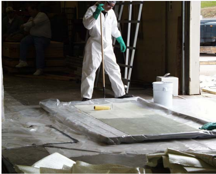
Figure 8.3 Saturating glass fabric with epoxy resin.
