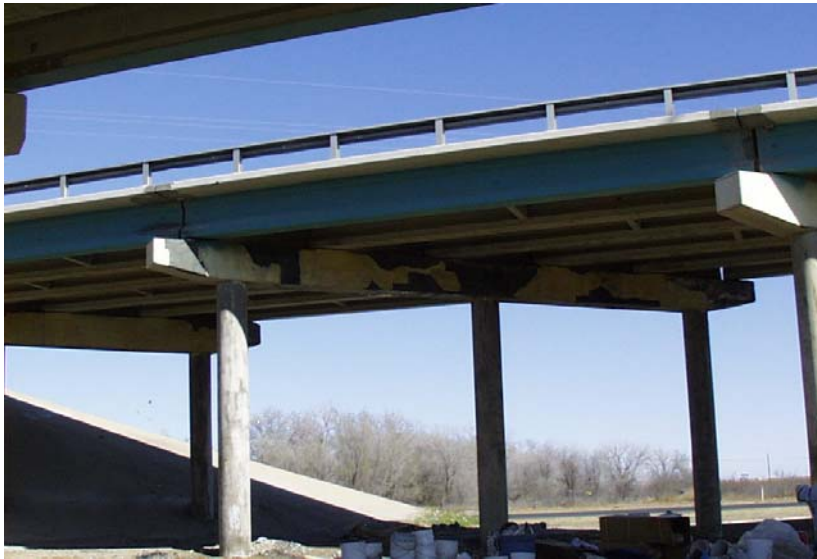
Figure 5.11 Structure #1 prepared for encapsulation.
