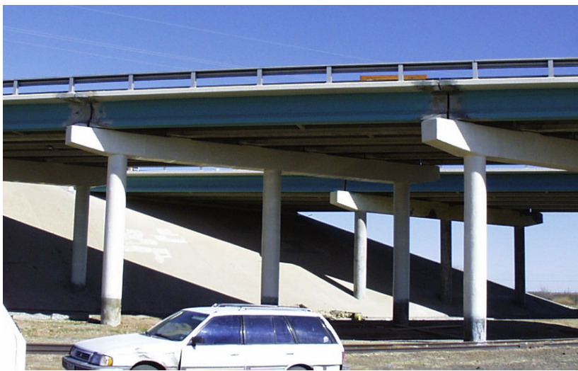
Figure 5.12 Structure #2 encapsulated with FRP wrap.
