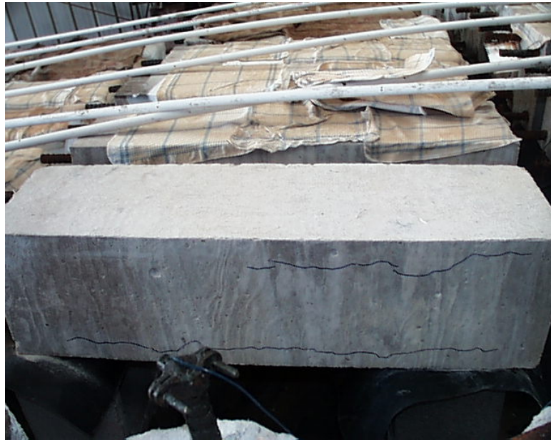
Figure 6.2 Longitudinal cracks forming on an uncracked specimen.
