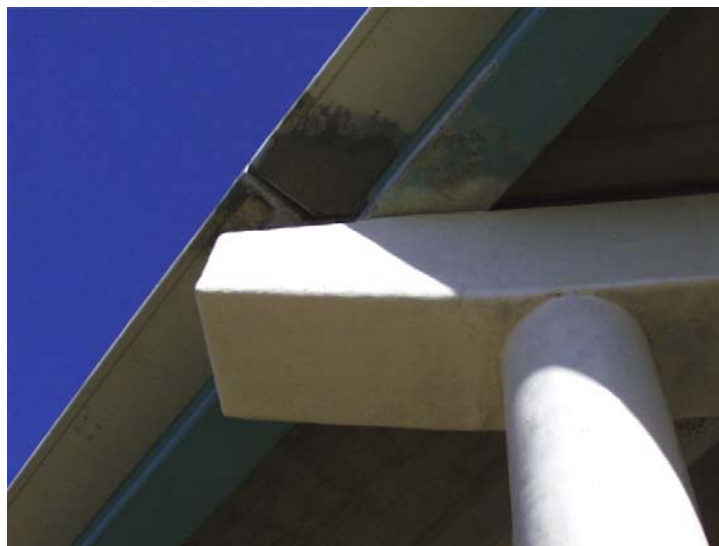
Figure 1.2 Bridge bent and column wrapped with FRP after repair of corrosion damage.
