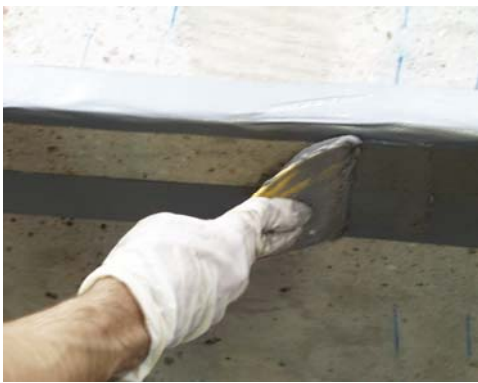
Figure 4.8.c: Apply epoxy resin.
