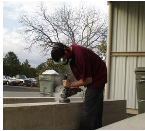
Figure 4.6.b: Grinding of the concrete surface.
