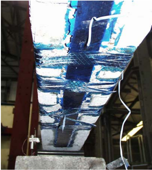
Figure 5.30.a: Debonding and slipping of longitudinal sheet initiated between the 2 nd and 3 rd strap; propagation of debonding along beam.
