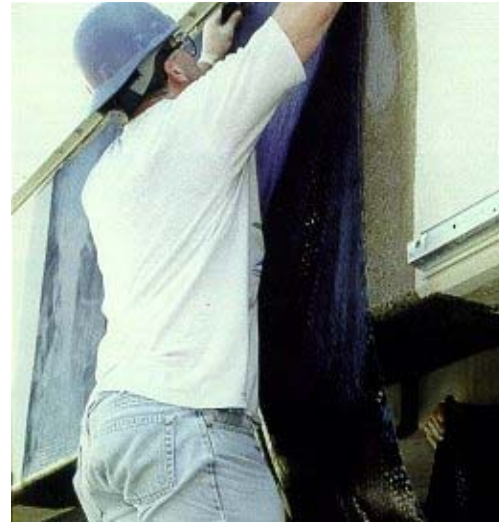
Figure 2.3.b: Guider flexural and shear strengthening
