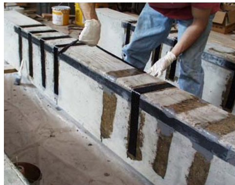
Figure 4.8.f: Apply CFRP flexible sheets for lateral anchorages.
