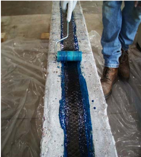
Figure 4.7.c: Apply slight pressure to impregnate the fibers.
