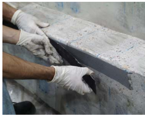
Figure 4.8.d: Place pultruded plate.
