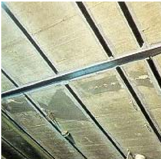
Figure 2.4.a: Slab flexural strengthening
