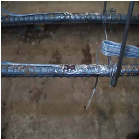
Figure 4.12.a: Electric strain gages on #5 reinforcing bars.
