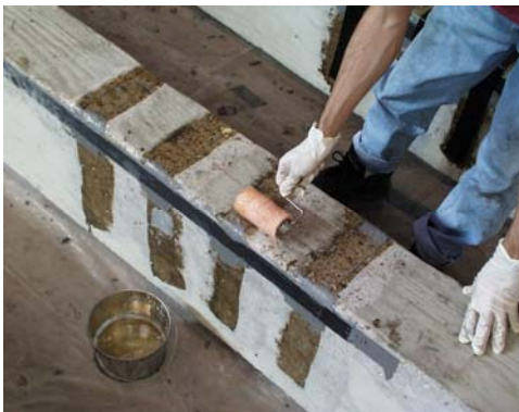
Figure 4.8.e: Apply epoxy resin for lateral anchorages.
