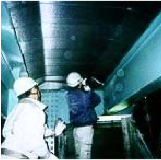
Figure 2.3.a: Slab flexural strengthening
