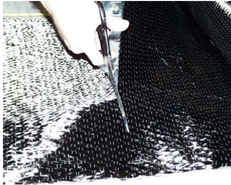
Figure 4.8.a: Cut CFRP flexible sheets.
