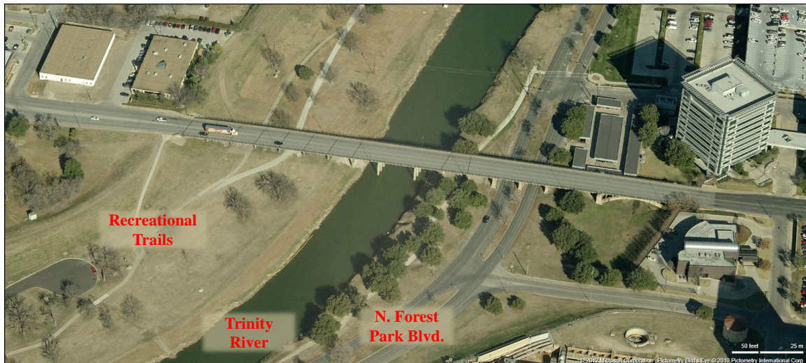
Figure 2-3: Existing Bridge (Bing Maps)
