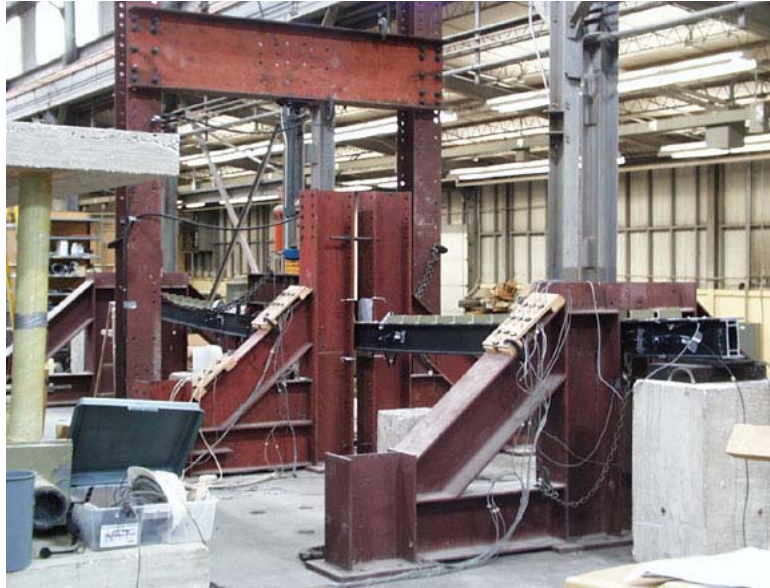
Figure 6.32: Specimen SW2 During Testing
