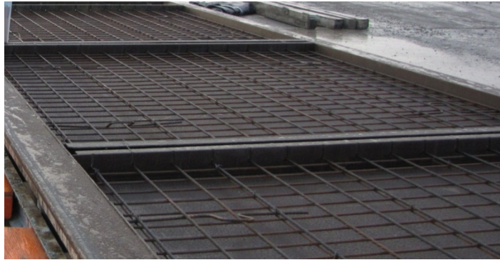
Figure 5.1 Welded wire mesh and strands in place at Plant B
