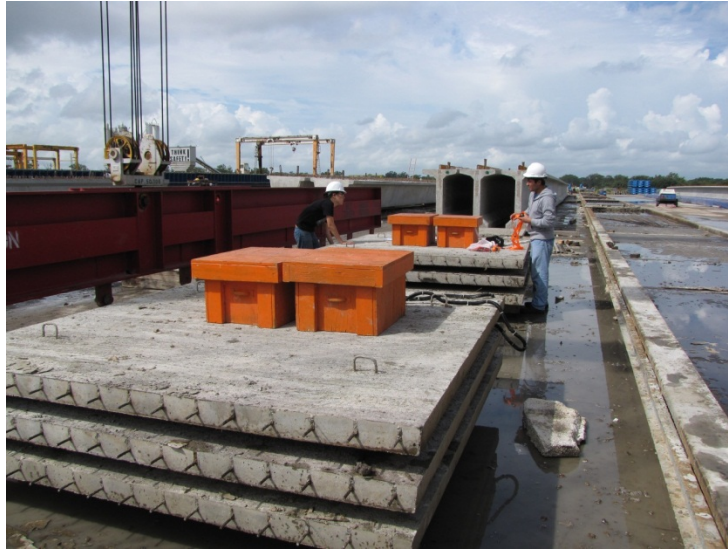
Figure 5.14 Panels stacked and stored at Plant B
