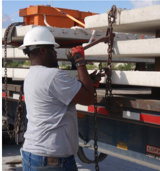
Figure 4.20 Panels strapped to flatbed truck, Plant A
