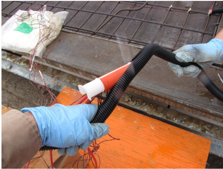
Figure 5.8 Routing wires at Plant B
