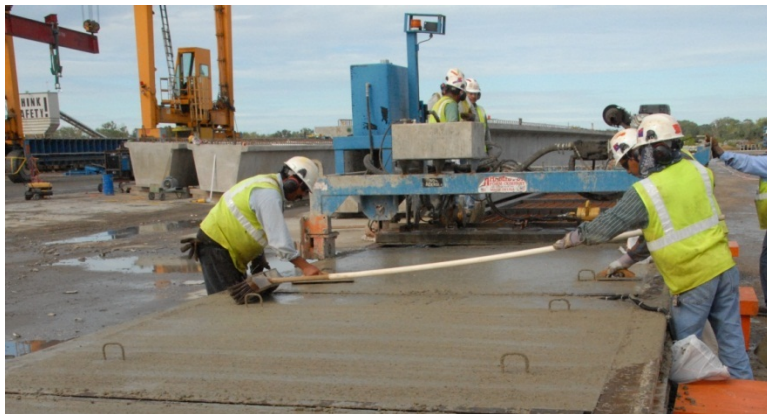
Figure 5.11 Vibrating, screeding and finishing concrete at Plant B
