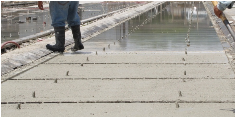
Figure 4.15 Panels being ponded with water at Plant A
