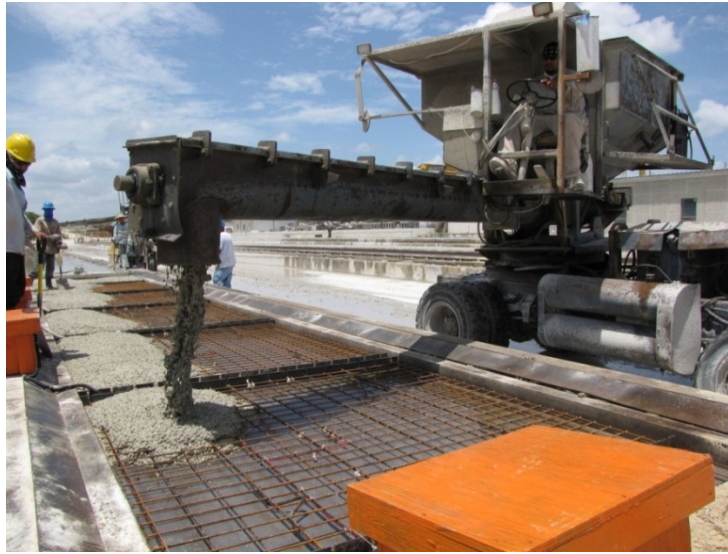
Figure 4.13 Casting concrete at Plant A
