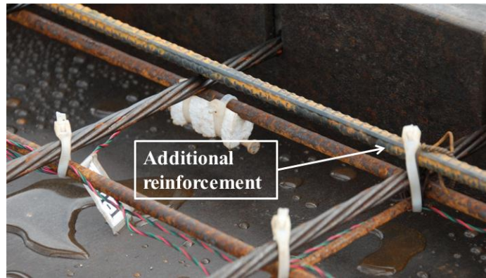
Figure 5.2 Two additional reinforcing bars at one edge at Plant B
