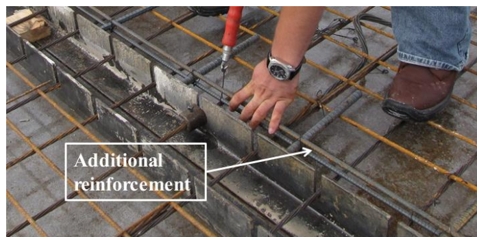
Figure 4.2 Two additional reinforcing bars at one end at Plant A
