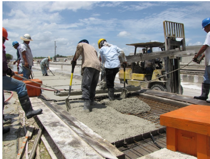
Figure 4.14 Vibrating and screeding concrete at Plant A
