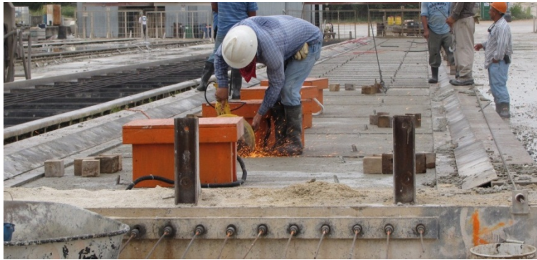
Figure 4.17 Interior strands being cut with chop saw at Plant A
