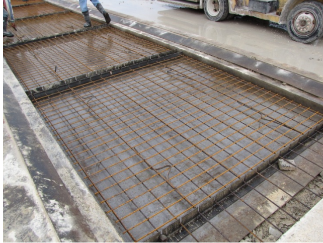
Figure 4.1 Welded wire mesh and strands in place at Plant A
