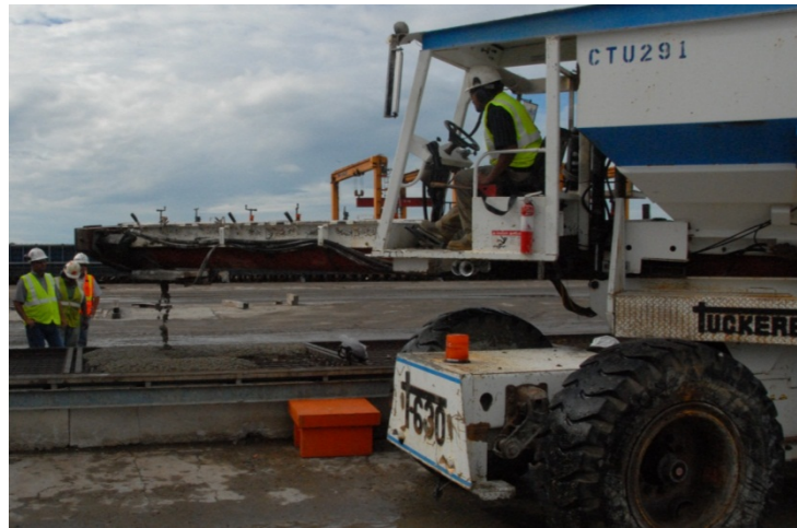
Figure 5.10 Casting concrete at Plant B
