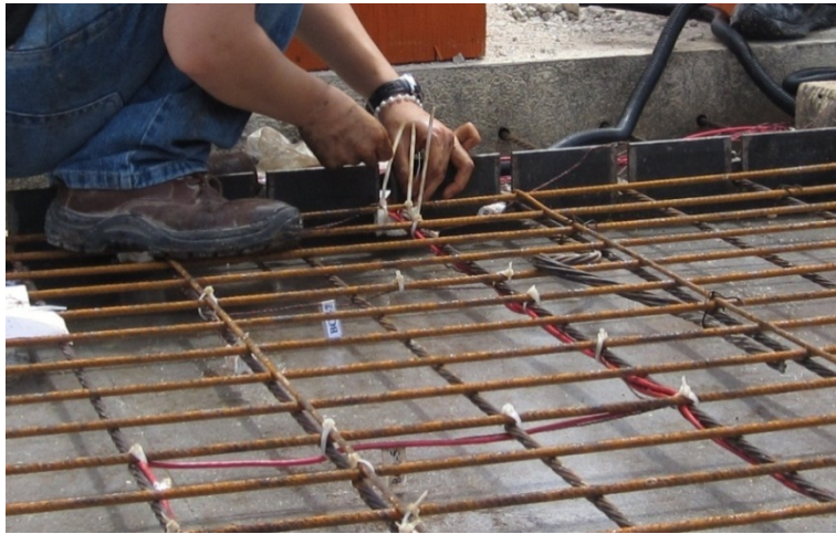
Figure 4.11 Installing gages at Plant A
