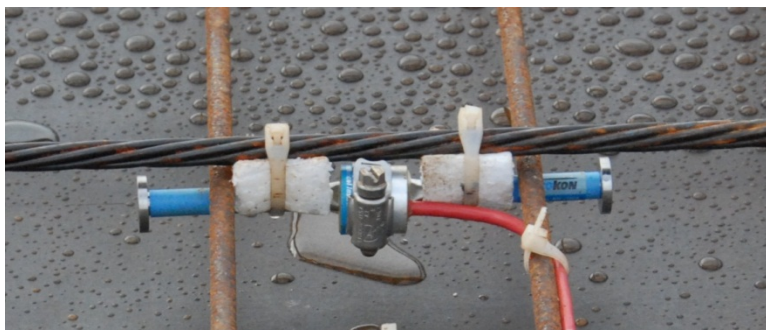
Figure 5.7 Vibrating-Wire Gage installed parallel to a prestressing strand
