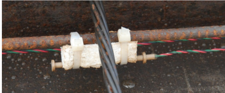
Figure 5.6 Embedment gage installed parallel to a transverse rebar
