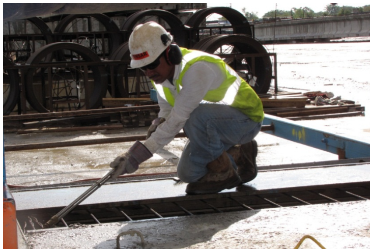
Figure 5.13 Strands being torch-released at Plant B
