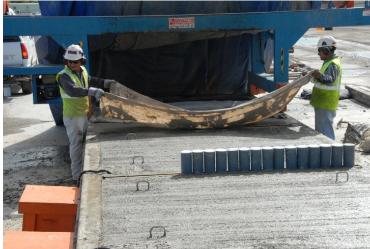
Figure 5.12 Panels being covered with wet blankets at Plant B
