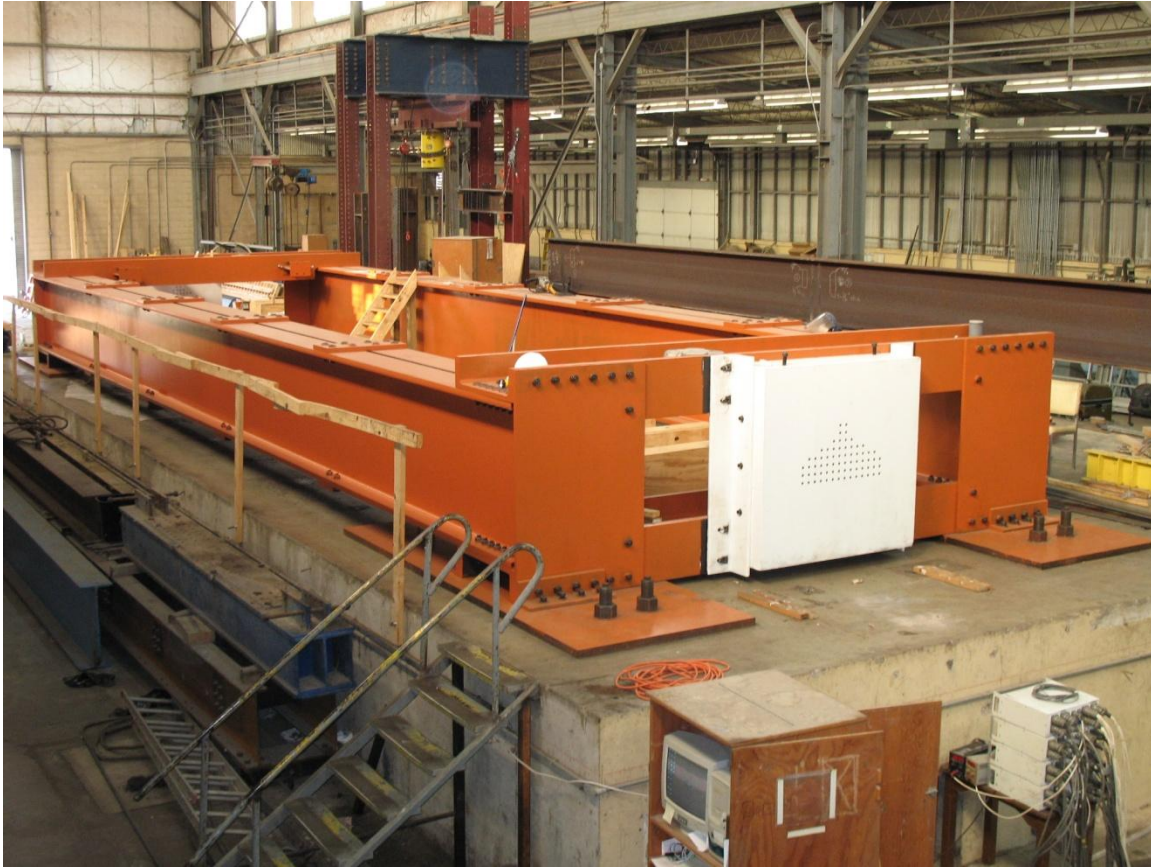
Figure 2-17: Prestressing Bed facility in FSEL
