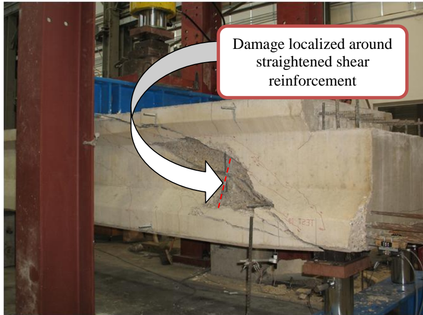
Figure 4-21: Failure of Square end of BB-09 (SCC).
