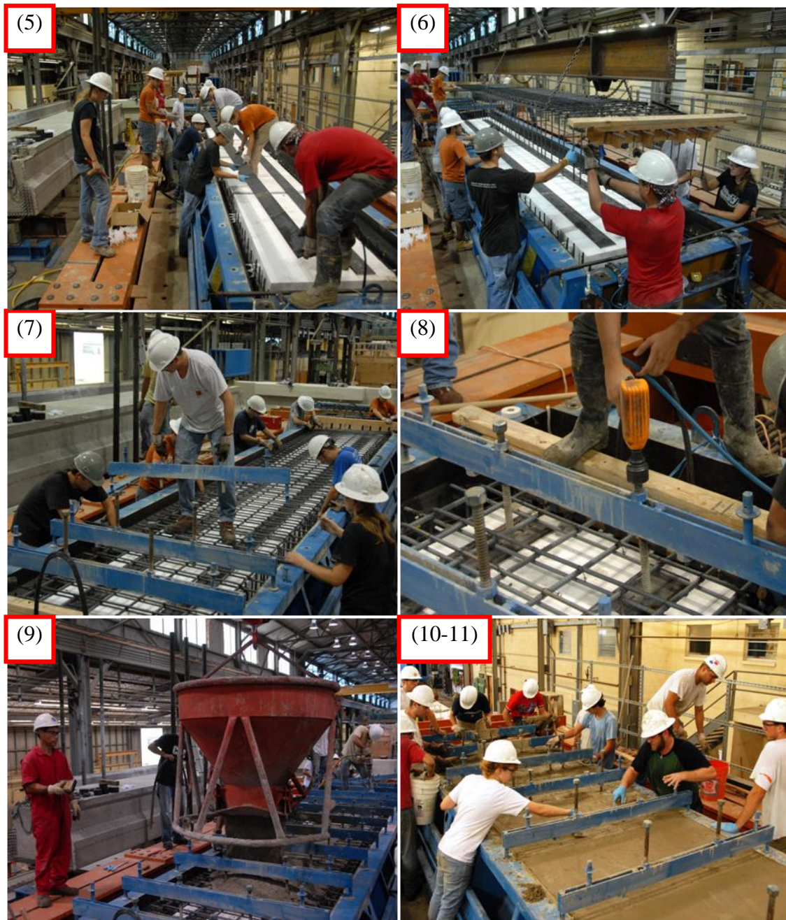
Figure 3-17: Step-by-step Box Beam fabrication process (continued)
