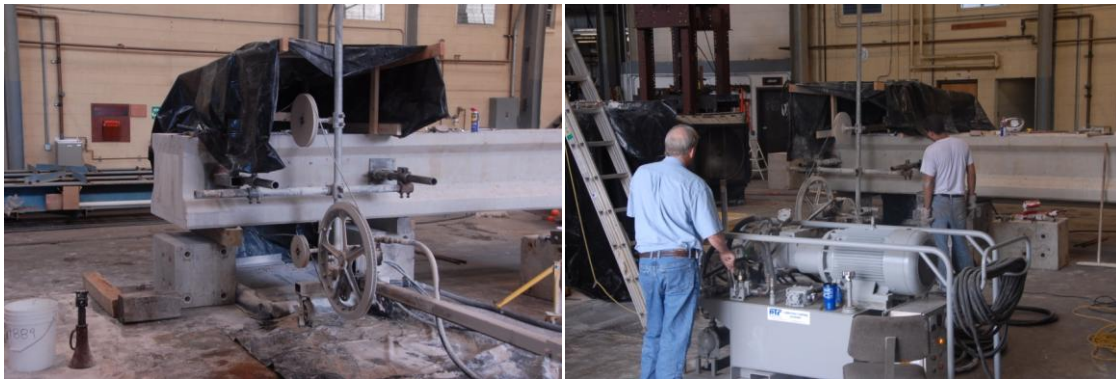
Figure 4-28: Diamond wire cutting saw cutting through 4B28 beam.
