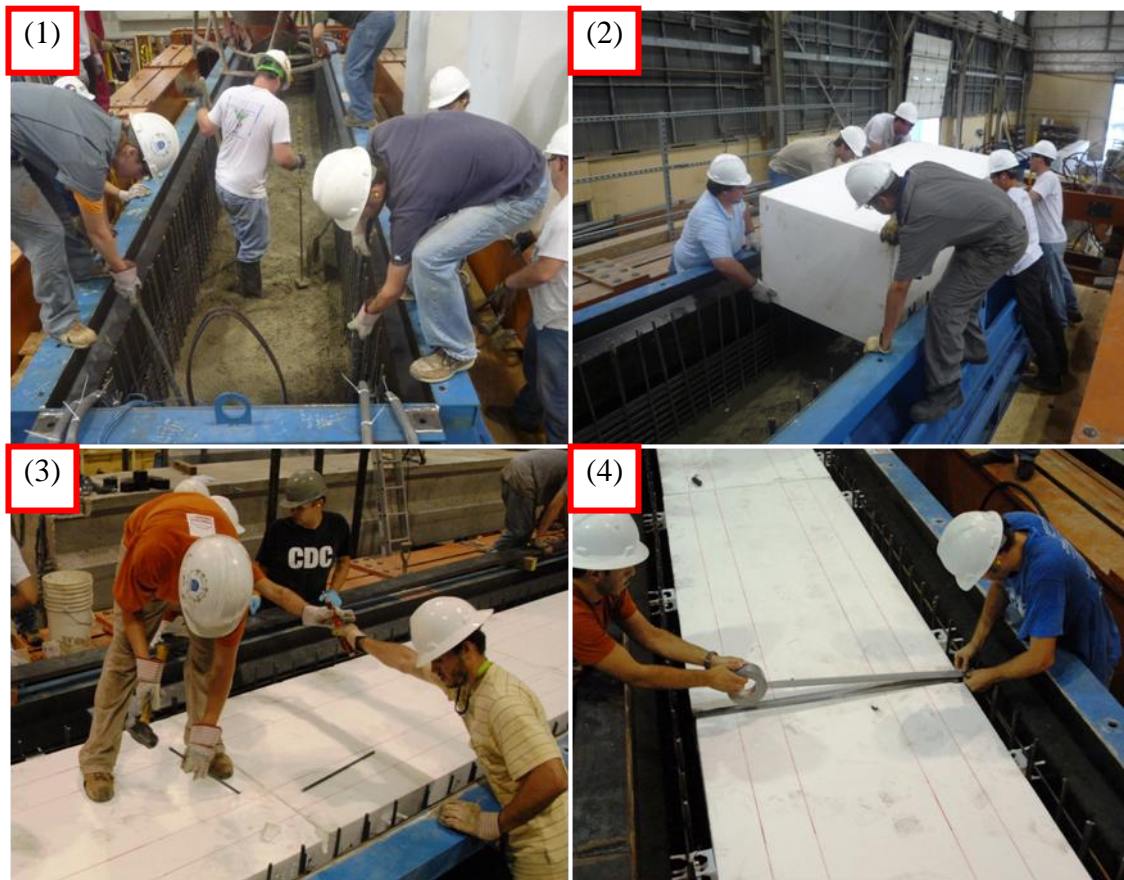
Figure 3-17: Step-by-step Box Beam fabrication process
