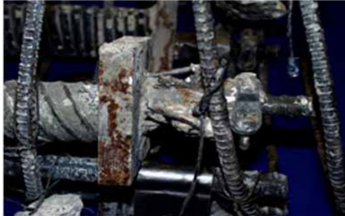
Figure 4.19 PT Bar Top Anchorage Condition for Specimen PT-TC-N-PD 1
