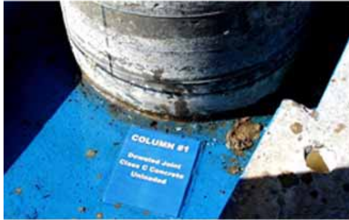
Figure 4.9 Condition of Specimen DJ-TC-N at the End of Testing 1
