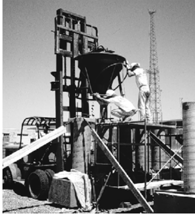
Column Reinforcement on Foundation
