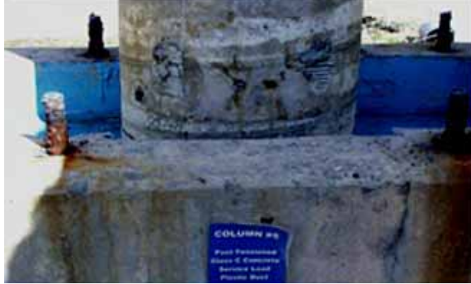
Figure 4.21 Condition of Specimen PT-TC-S-PD at the End of Testing 1
