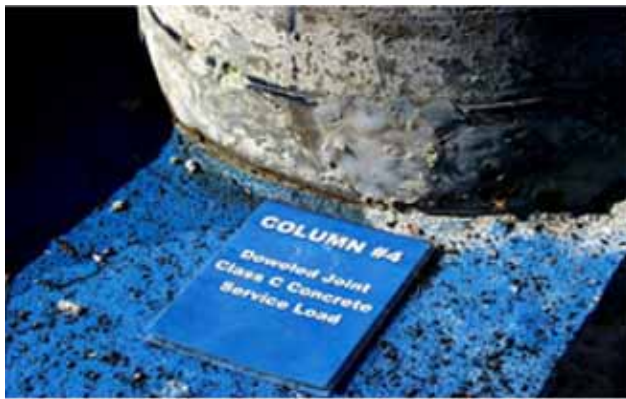
Figure 4.13 Condition of Specimen DJ-TC-S at the End of Testing 1
