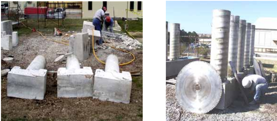
Figure 4.1 Saw Cutting of Column Foundation 1
