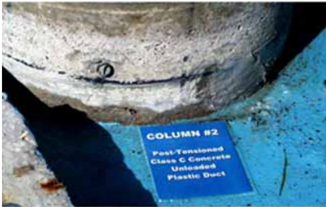
Figure 4.17 Condition of Specimen PT-TC-N-PD at the End of Testing 1
