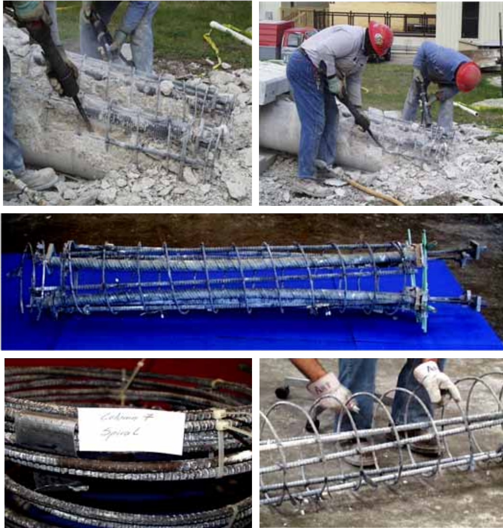
Figure 4.2 Concrete Removal and Reinforcement Dismantling 1
