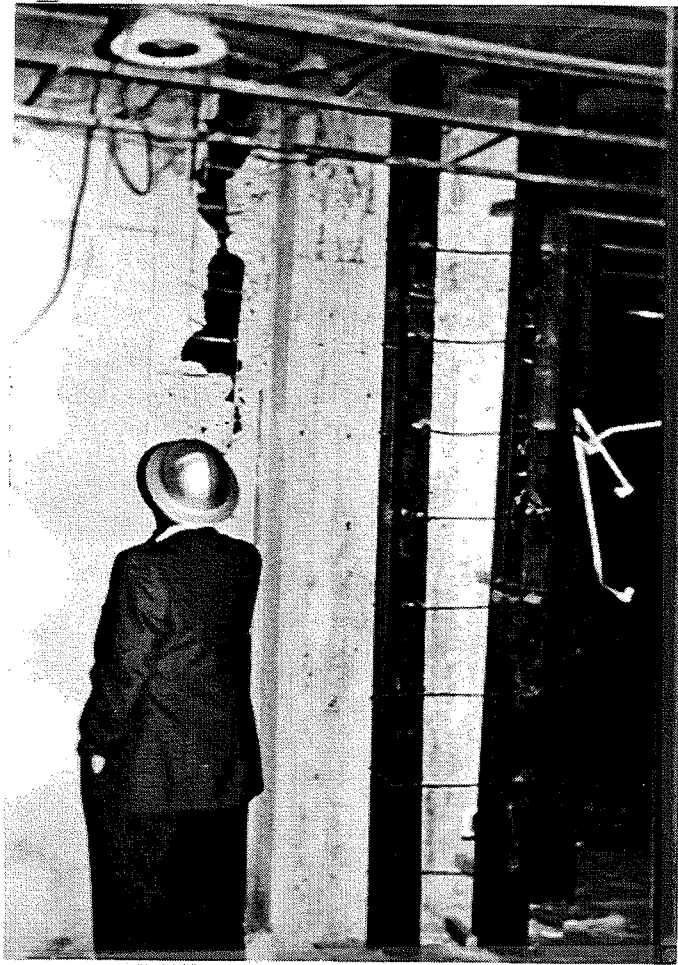
Figure 5- F8 Damage in concrete walls
