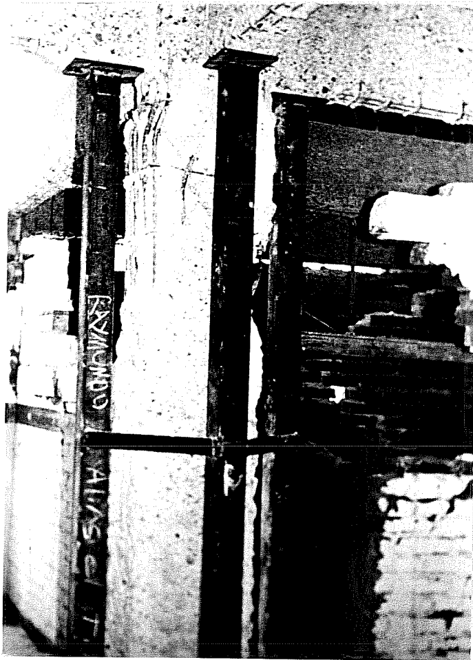
Figure 5- A5 Short column failure
