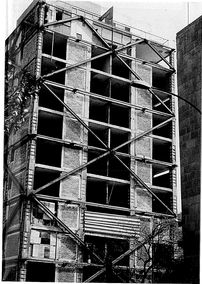
Figure 5- B18 Bracing system
