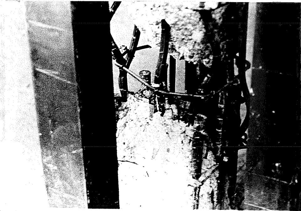
Figure 5- A3 Excessive splicing of reinforcement
