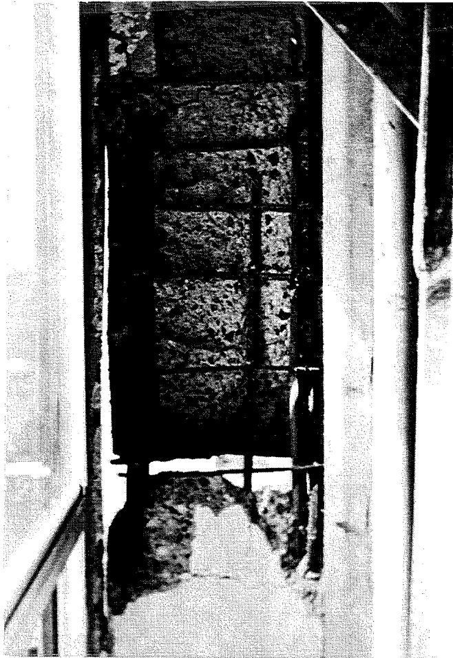
Figure 5- H5 Damage in column A-1 due to pounding with adjacent building
