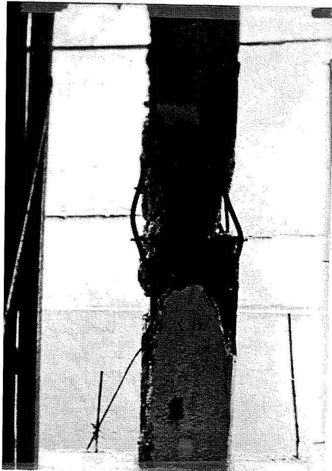
Figure 5- H3 Damage in column D-3
