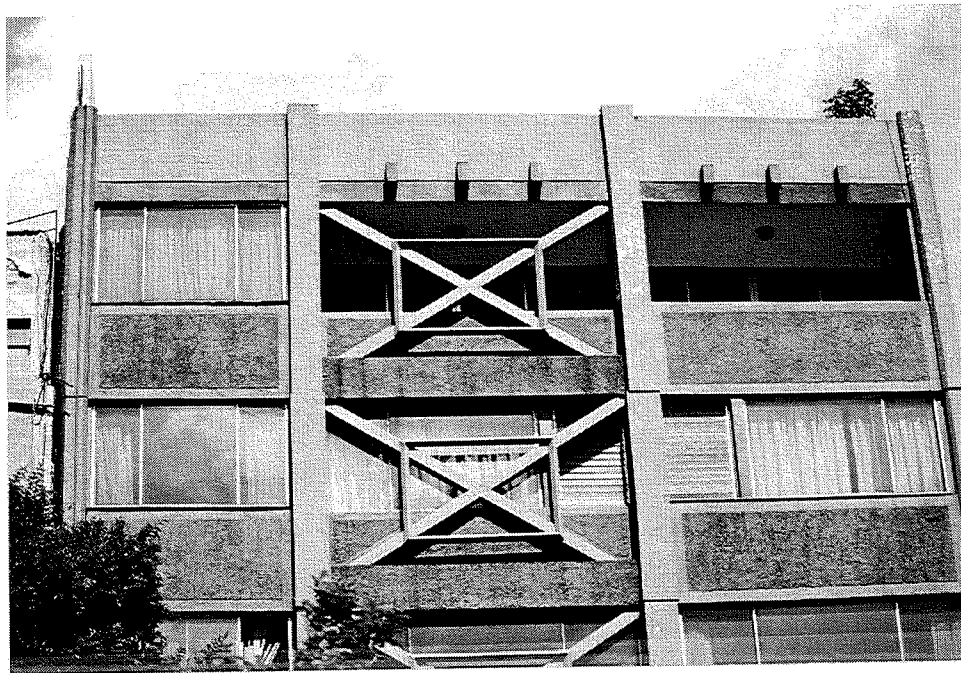
Figure 5- J8 Steel bracing in the upper levels
