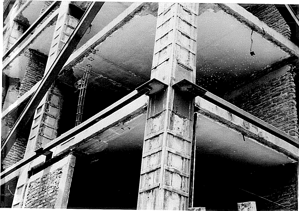
Figure 5- B15 Connection between collector elements
