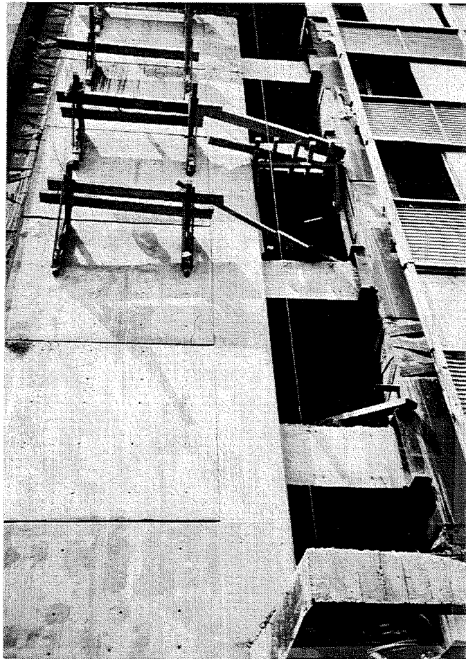
Figure 5- L9 Reinforced concrete wall in line A
