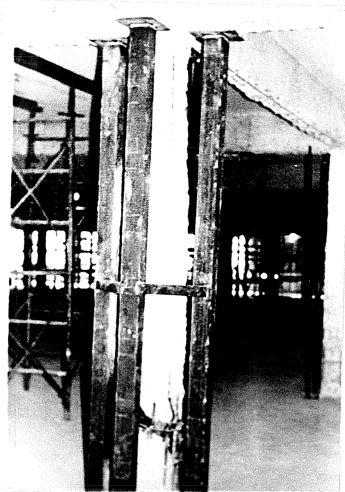
Figure 5- A4 Failed column
