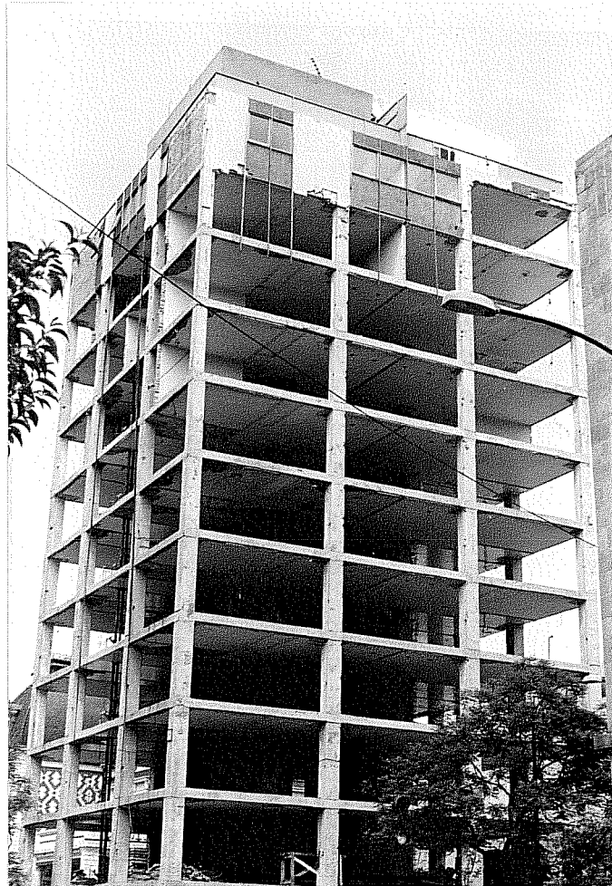
Figure 5- B3 Facade removal
