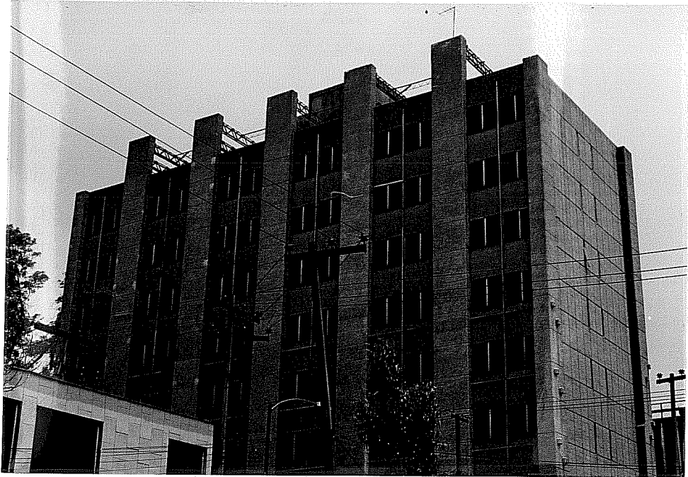
Figure 5- C10 Retrofitted building
