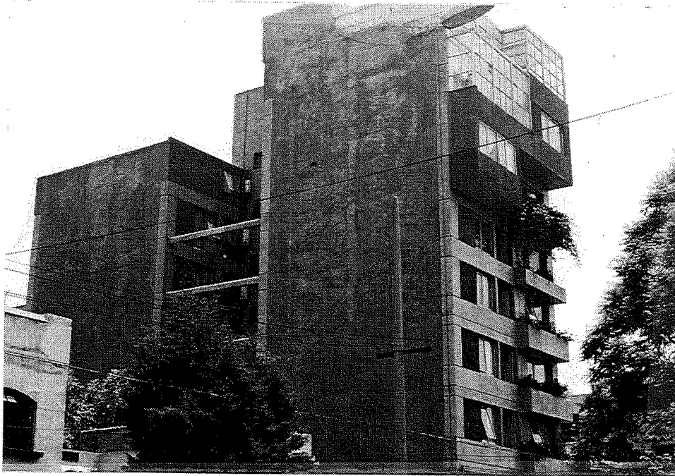
Figure 5- E18 Repaired building
