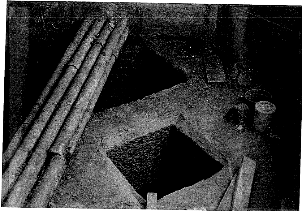
Figure 5- B6 Pile cap
