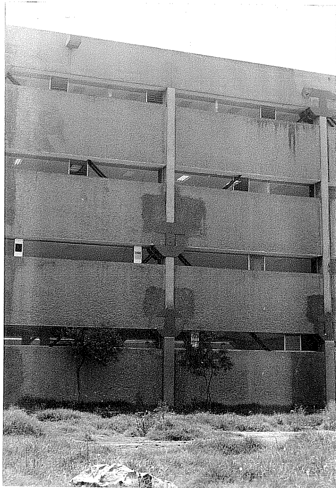
Figure 5- D5 Cable brace in line A
