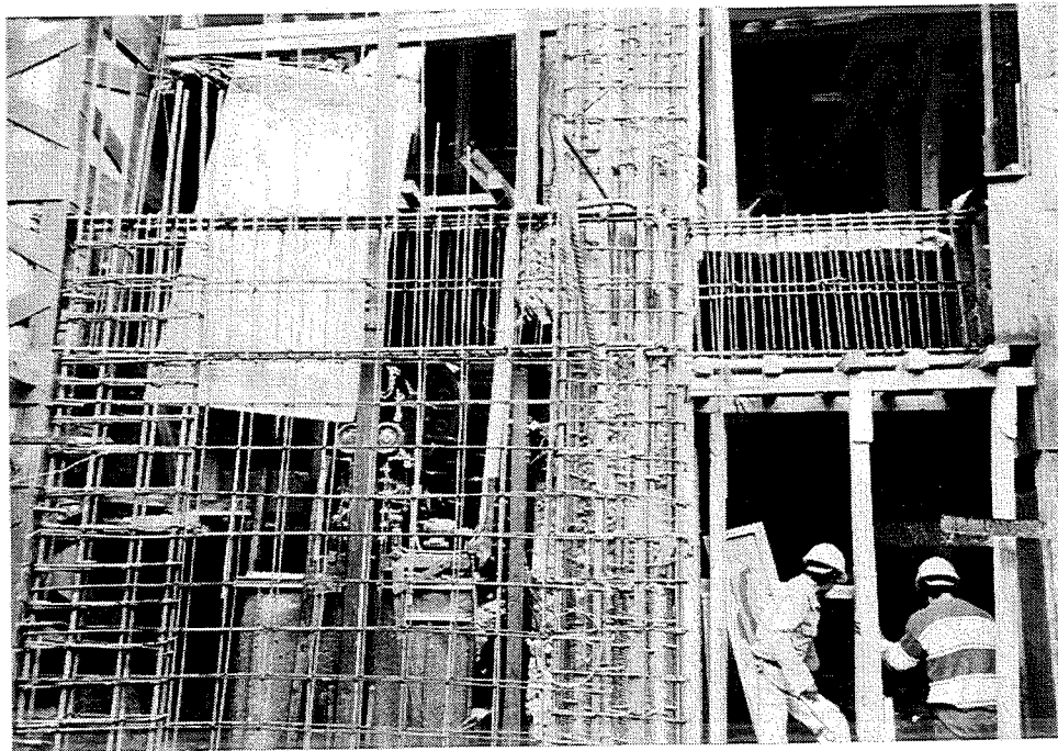
Figure 5- L8 Reinforcement in new concrete wall
