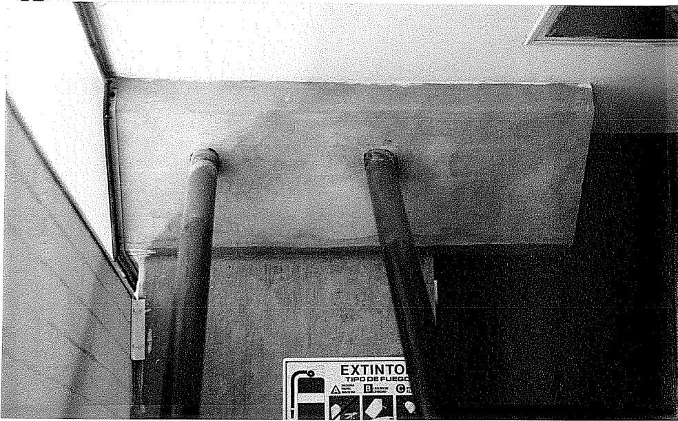
Figure 5- D8 Cables through slab-column joints
