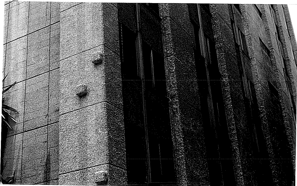
Figure 5- C11 Post-tensioning cable anchorage after completion of project
