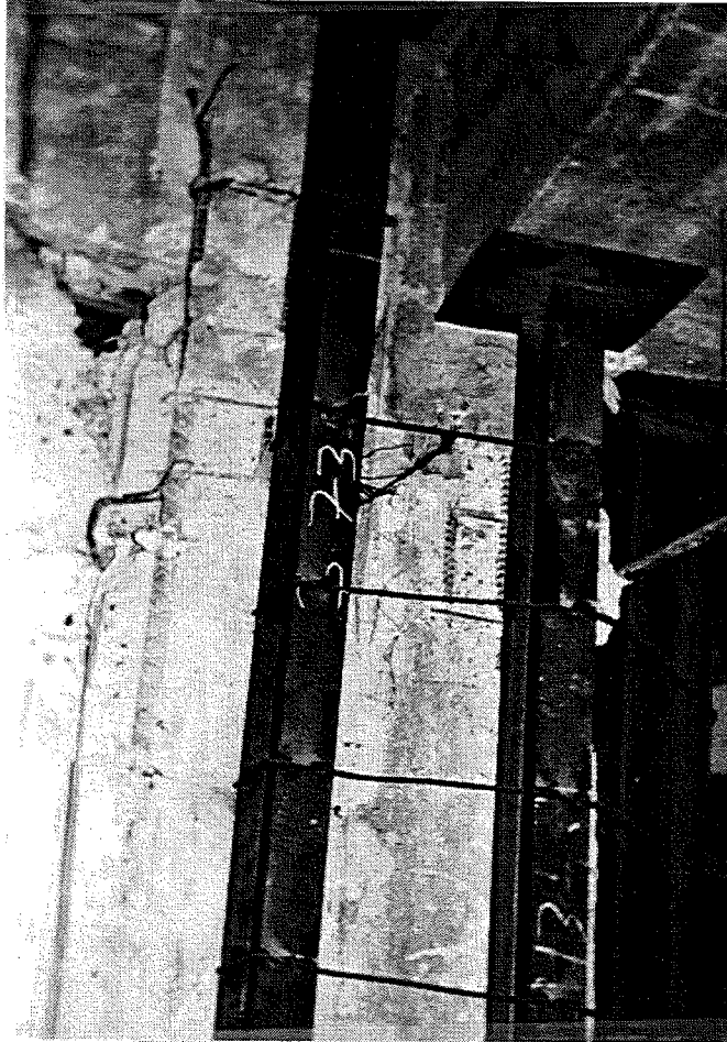
Figure 5- F11 Shoring for vertical loads
