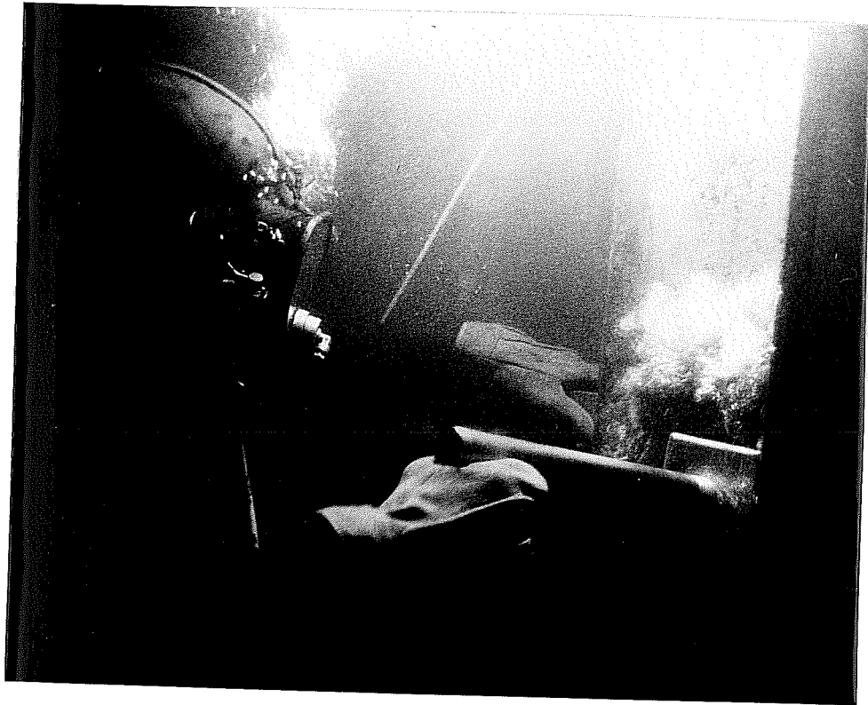
Figure 2.1 Diver using an underwater powder actuated tool. (photo courtesy of ITW Ramset/Redhead).
