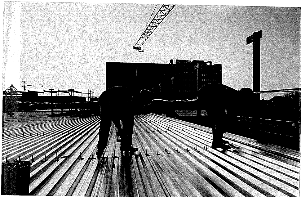
Figure 2.7 Metal floor decking with shear connectors for composite beams. (photo courtesy of Hilti)
