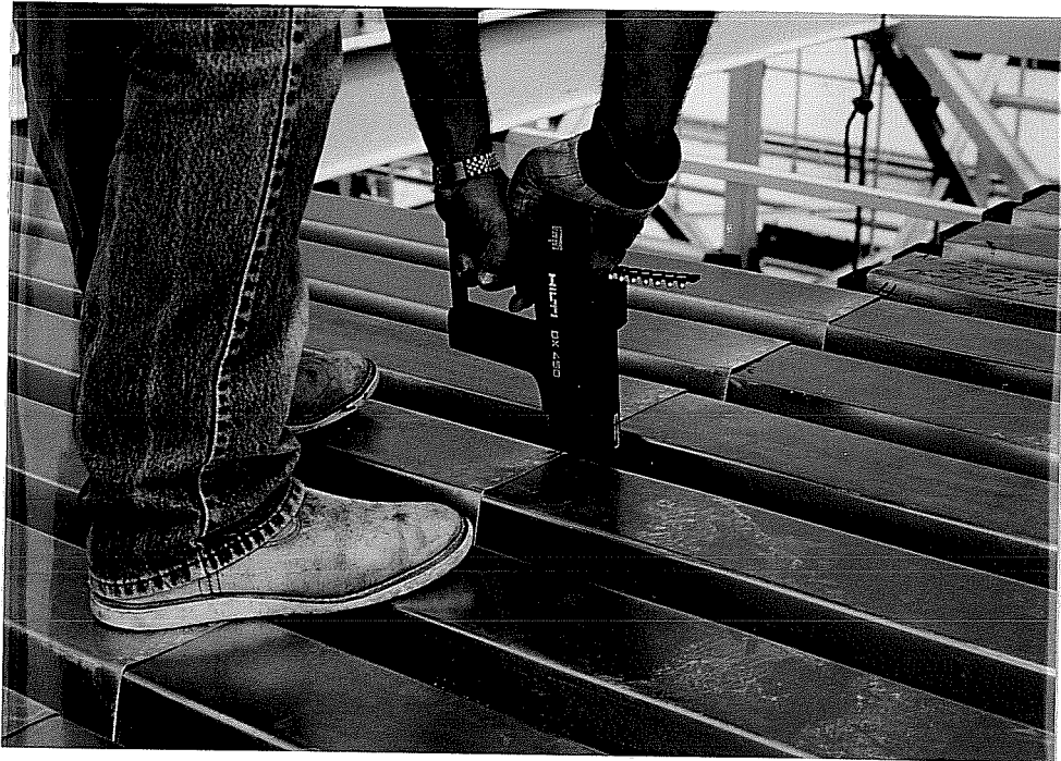
Figure 2.6 Metal floor decking. (photo courtesy of Hilti)
