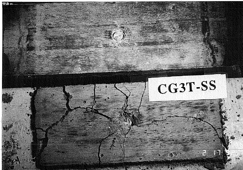
Figure 4.66 Cracking of interface grout – Test CG3T-SS.
