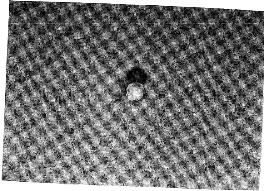
Figure 3.18 Sandblasted concrete surface.
