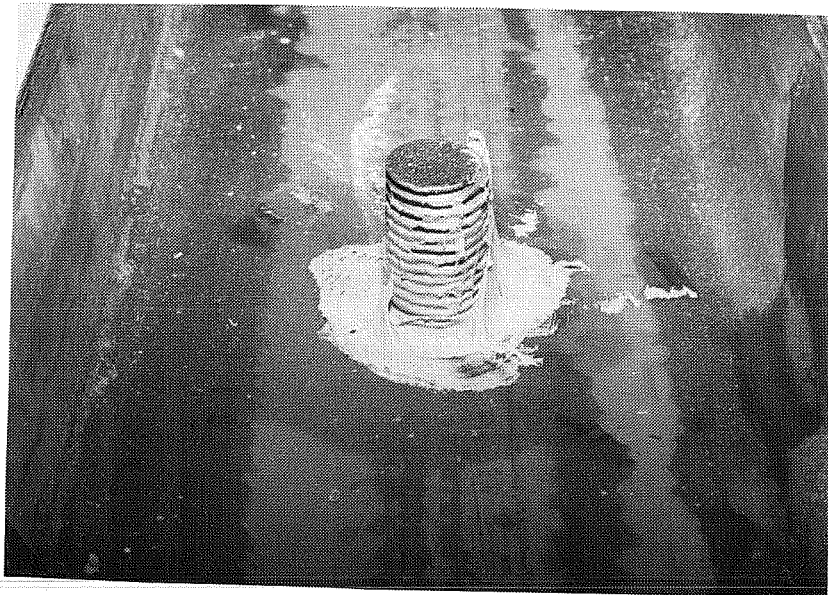
Figure 3.21 Channel in position with extruded adhesive.
