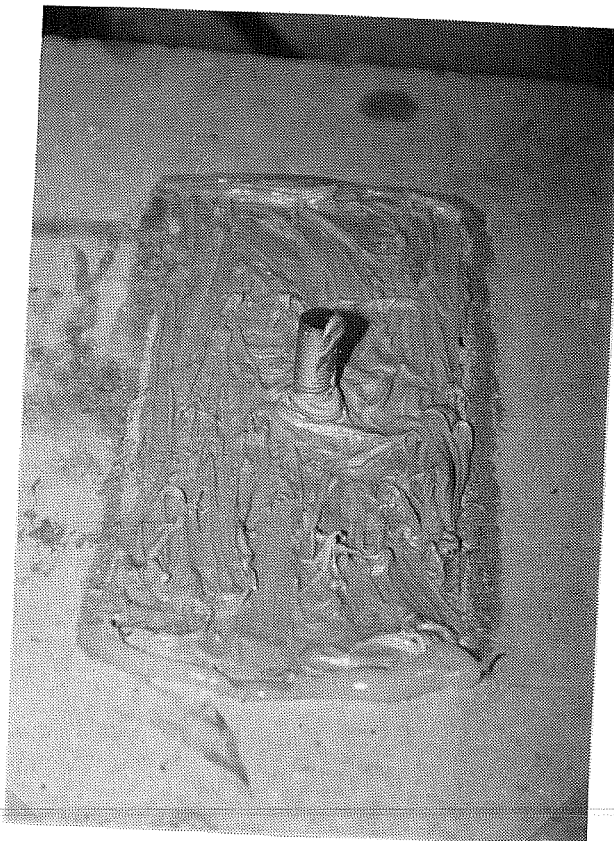
Figure 3.19 Epoxy adhesive in place over concrete surface.
