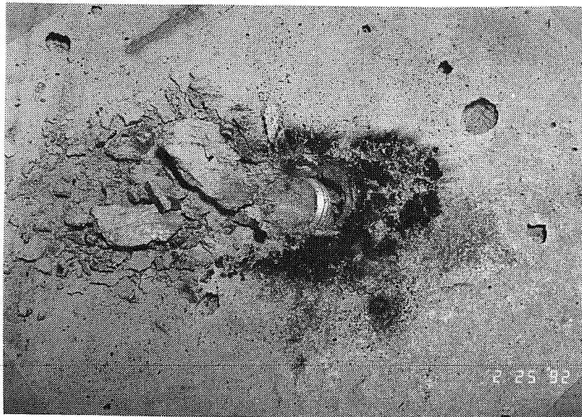
Figure 4.53 Crushing of concrete around bolt hole – Test CN3h-WN.
