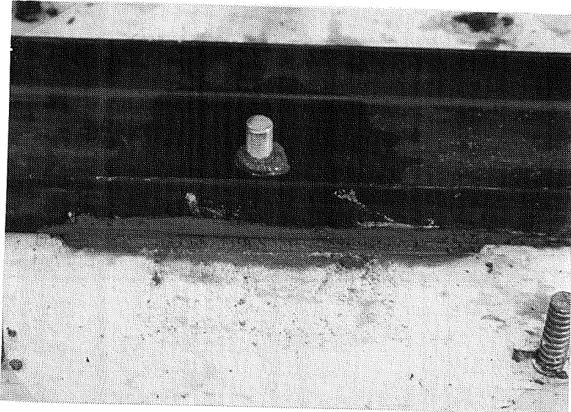
Figure 3.24 Channel placed over applied grout.
