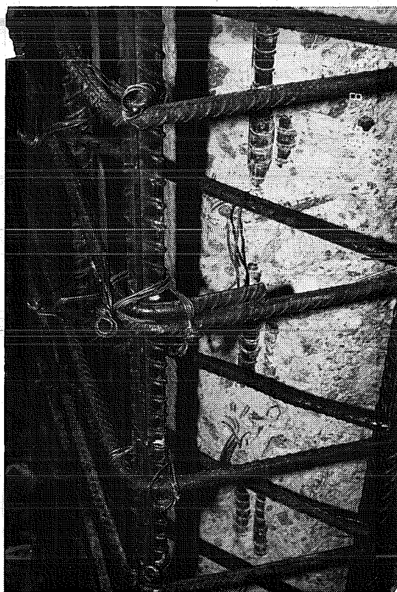
Figure 1.5 Column Jacketing Using Distributed Reinforcement
