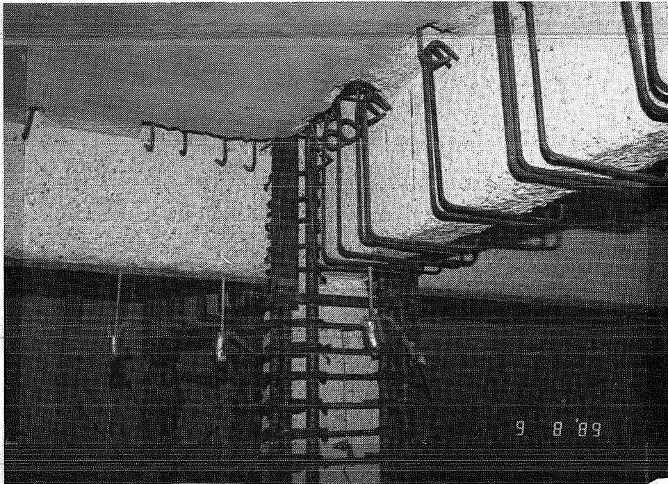
Figure 2.16 Specimen SD-B - Assemblage of Beam Jacket
