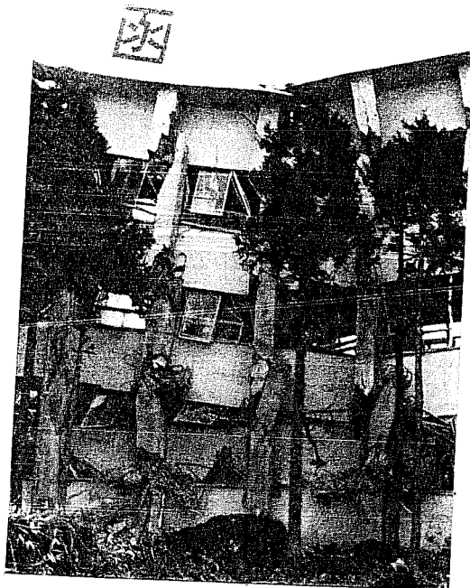
Fig. 1.2 Hakodate University (1968 Tokachioki Earthquake)
